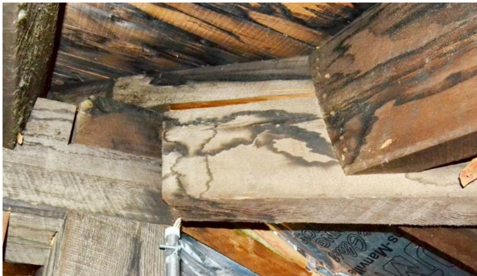
Figure 10 Split in a notched timber
