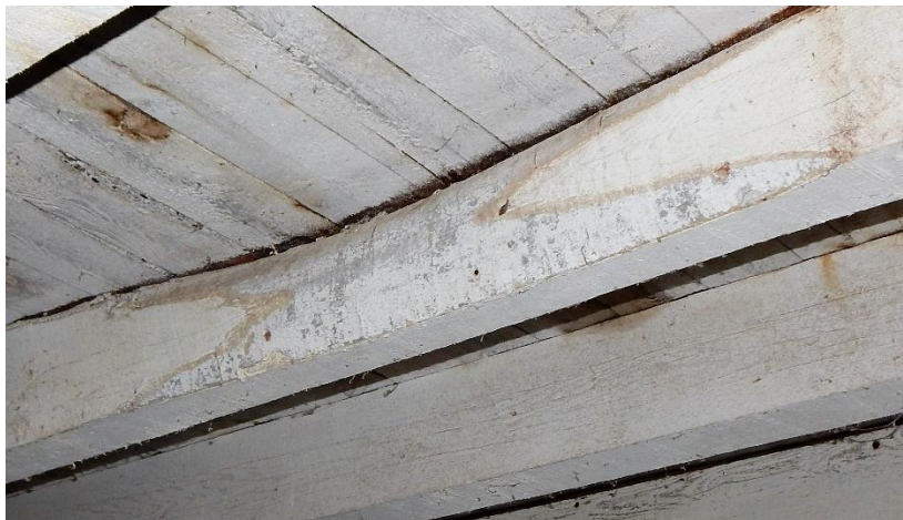
Figure 30 Joist in service with wane that exceeds grading rule limits
