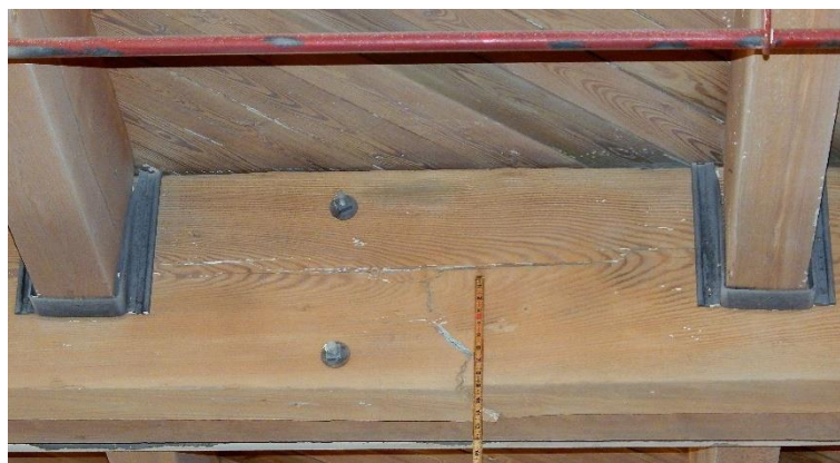
Figure 29 Fracture terminating at a check
