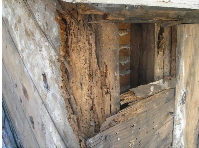
Figure 5 Termite damaged timber
