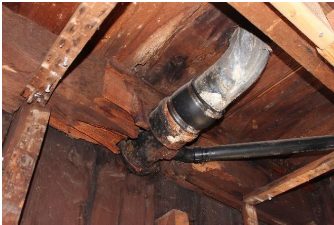
Figure 7 A timber that has been compromised
