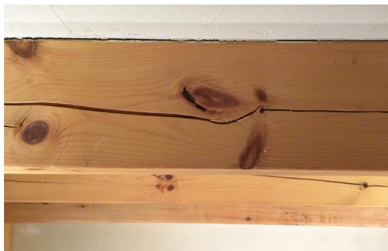
Figure 28 Grain deviation at knots
