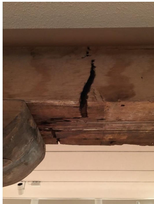
Figure 8 Fractured timber due to overloading
