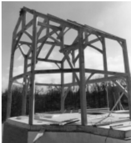
Figure 1. — Timber framing shown for a “great room” near Blacksburg, VA. Nominal timber sizes typically range from 140 mm (6 in.) by 140 mm (6 in.) to 292 mm (12 in.) by 292 mm (12 in.) and common species include southern pine, Douglas-fir, and mixed oak.
