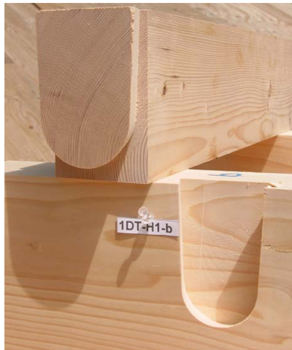
Figure 1-1: Rounded Dovetail Connection
