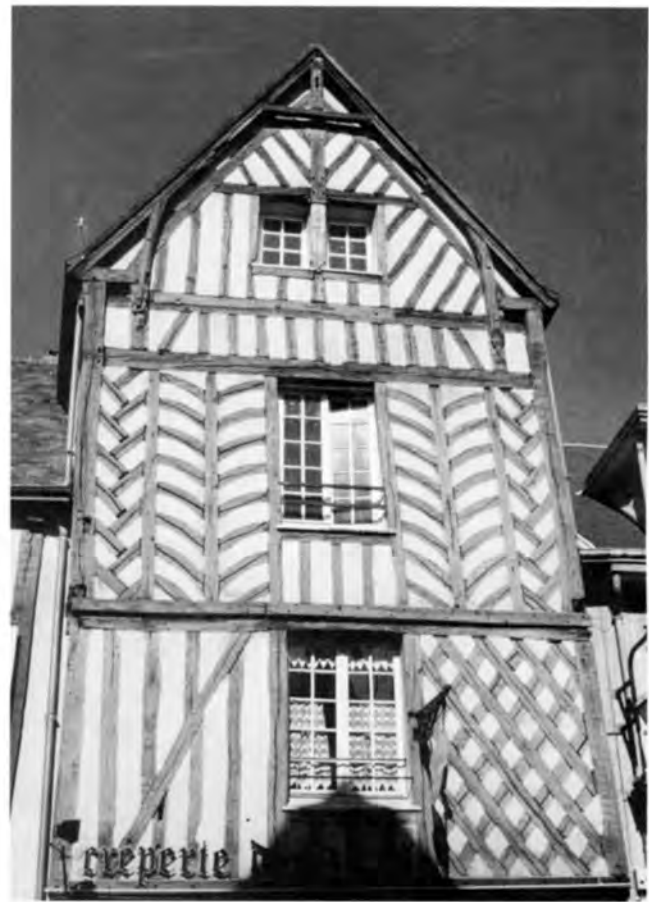
Above and below, restaurants and crêperie in old Chartres. Direction of down bracing is not intuitive. Framed overhang is typical. Below left, a tower enjoys a fresh coat of paint over its plaster.
