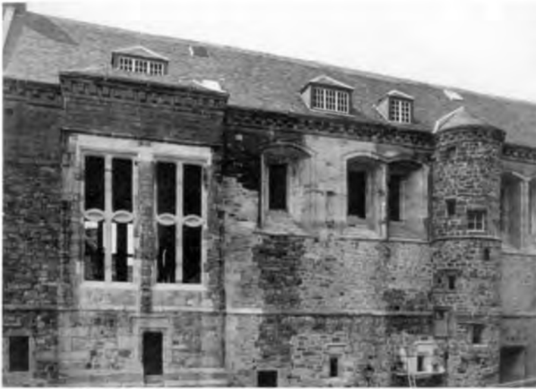
At top, model of Stirling's Great Hall as it will appear when restored to its 16th-century form, including parapets and uninterrupted roof. Above, the east wall and the 18th-century dormers before restoration. Sash, casements have been removed to make way for medieval glazing.
