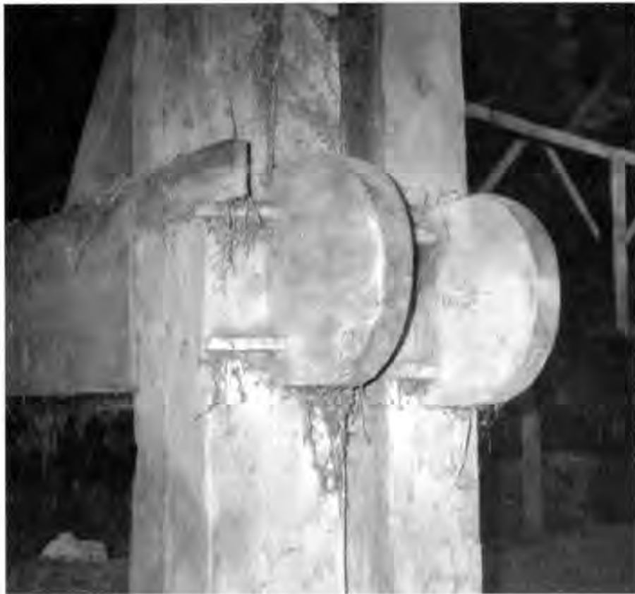
Two Dutch barns set end to end in an exceptional arrangement, Montgomery County, New York. Pine anchorbeams, typically rounded through-tenons.
