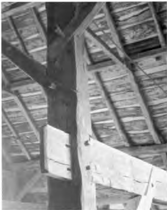
Oak anchorbeam at Saugerties, New York. Typical square, chamfered through-tenon. Outside wedges missing.
