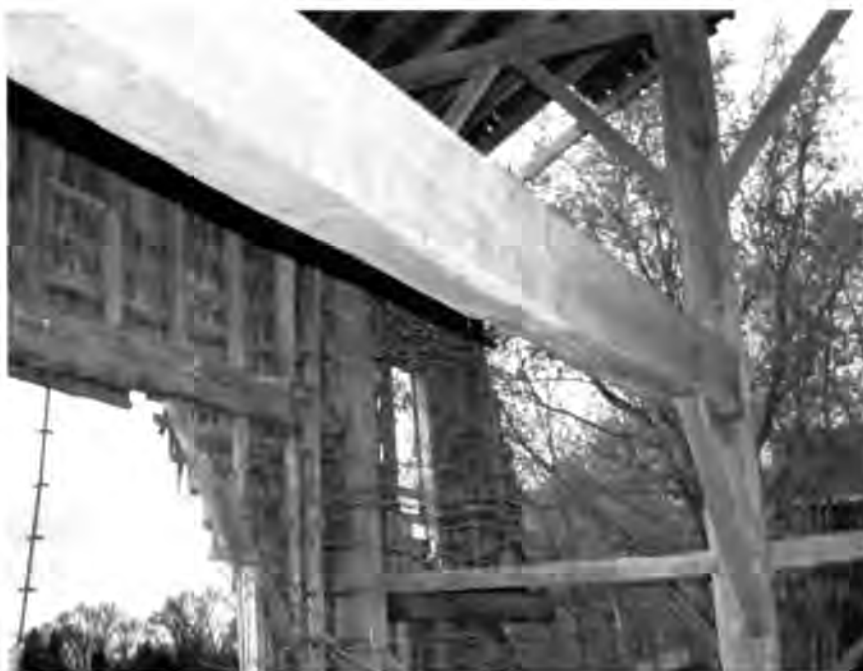
Somerset County, New Jersey, Anglo-Dutch barn with oak anchorbeams 22 in. deep. The roof has been rotated 90 degrees over the H-frames.
