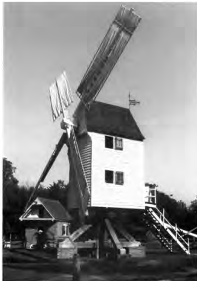
Colonial Williamsburg The post mill at Williamsburg, a rare form of windmill, of which only reproductions exist in America. Below, a restored stone-built French smock mill. Only the cap turns.
