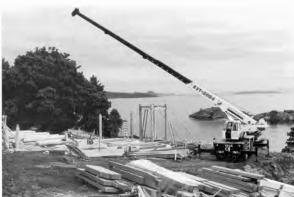
Framing for the central spine takes shape in view of a watery paradise and will support the arched portion seen in the end view (facing page) of the finished house.
