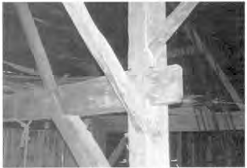
Anchorbeam-column joint, Richer barn, ca. 1750, Saugerties, N.Y.
