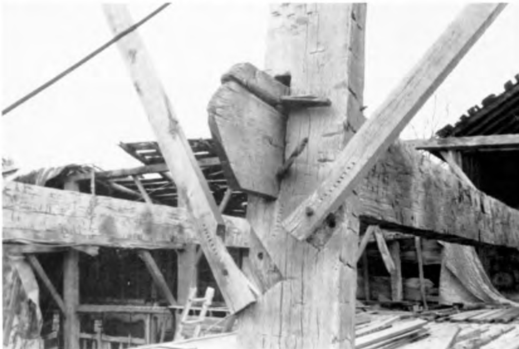
Dutch Barn Lap Dovetail Joinery
