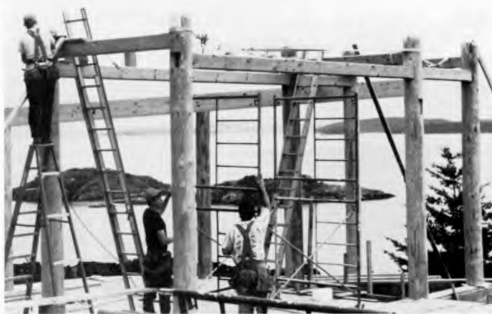
Framing for the central spine takes shape in view of a watery paradise and will support the arched portion seen in the end view (facing page) of the finished house.
