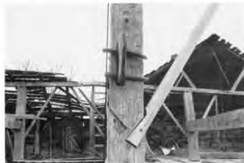
The ruinous Hoornbeck barn, Accord, N.Y., dated 1766, showing cup marks and the characteristic short verdiepingh. Lap-scarfed purlin plate in background. See also cover photo.
