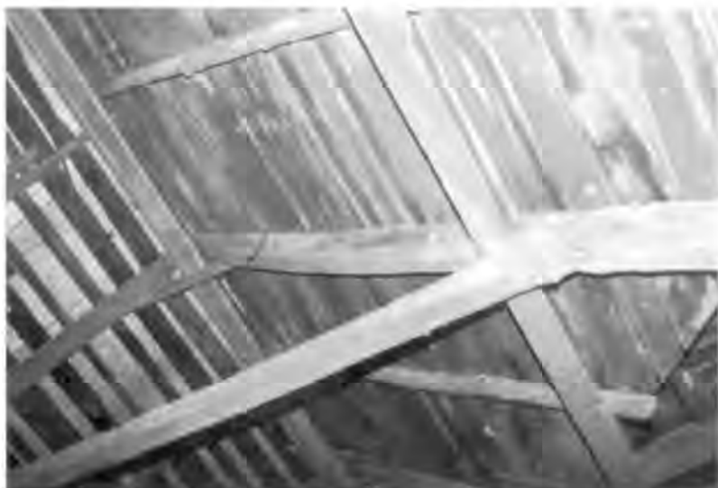
Secondary clapped purlin, ridge beam and pole rafter roof, barn in Accord, N.Y. Collars dovetailed to rafters, clapped purlins supporting alternating pole rafters, ridge detail mysterious.
