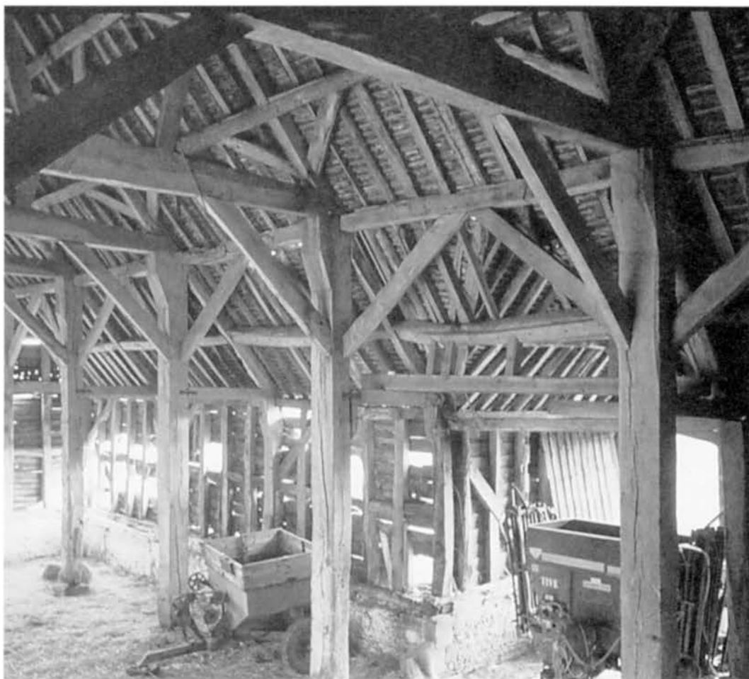
Above, view of south arcade, central threshing floor and east three bays, face to threshing floor; shared brace mortises in plate. Below, queen post collar cross-frame fully wind-braced, butt purlin roof.
