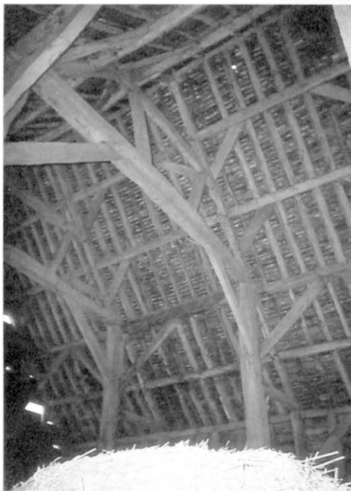
Above, view of south arcade, central threshing floor and east three bays, face to threshing floor; shared brace mortises in plate. Below, queen post collar cross-frame fully wind-braced, butt purlin roof.
