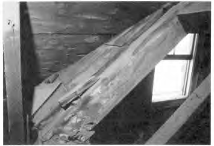
11. Original roof boards on a house in Cohoes, New York, with beveled lapped edges preserved by a later ell roof.
