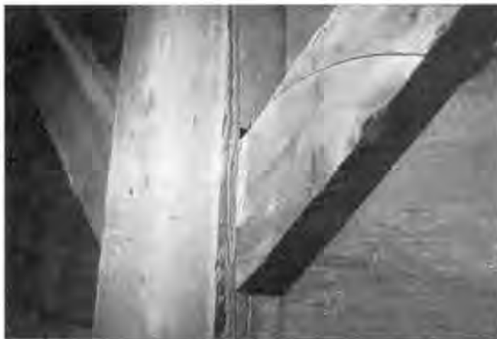
2. The braces in this Massachusetts barn were thickened by pushing them partially into a table saw.
