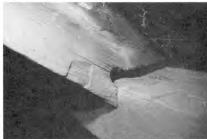
8. In this Orange County, New York, barn, the hole was likely bored over the line to save chiseling work.
