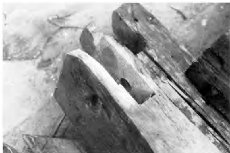
6. Rip-sawed rafter peak mortises in a Cohoes, New York, Dutch house.
