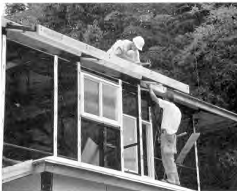
Assembling a typical house maker's steel-framed house.
