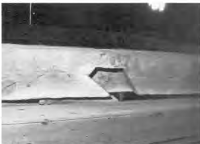
4. Lap dovetail mortises often have the acute angled point squared off at the width of the chisel used.
