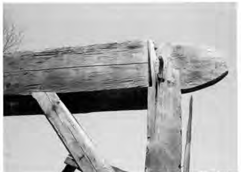
1. Exposed anchorbeam tenon in a ruinous Dutch barn showing broadaxed surface.
