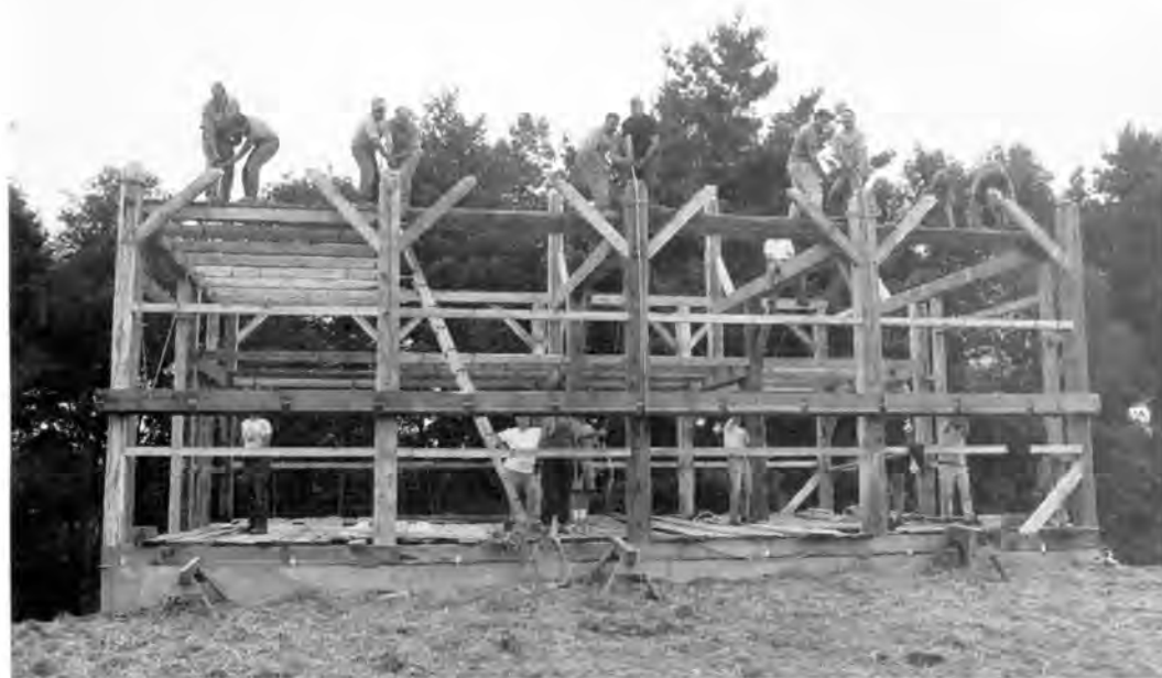
10. Parbuckling a 40-ft. 8x10 plate on a barn, Lenoxdale, Massachusetts.
