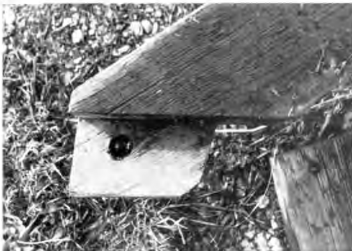
3. Reducing the width of a brace tenon saves on mortising work.
