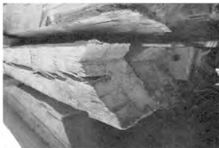
7. Dutch barn rafter butts showing evidence of bored and chopped birdsmouths.
