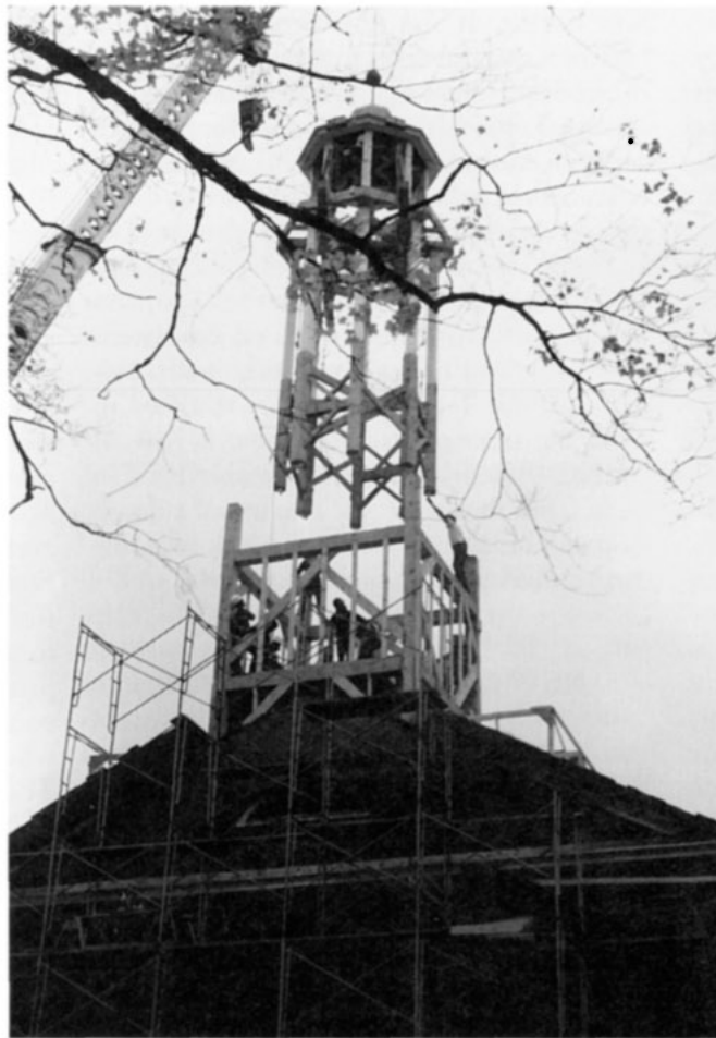
Jan Lewandoski Setting of steeple into reconstructed roof of meeting house (1826), at Weathersfield, Vermont, 1988.
