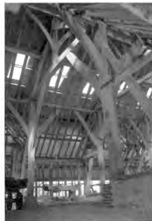
A typical crossframe. Note early repair strap.
