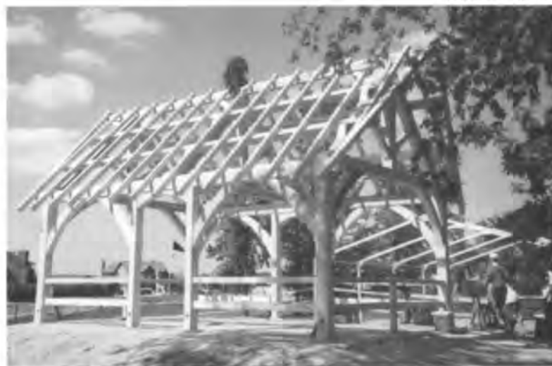
And the finished frame ready for roofing.
