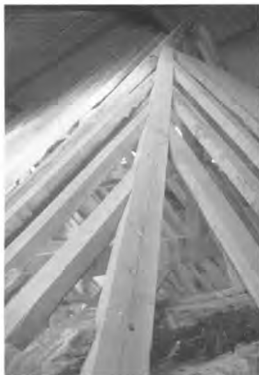
Views of the reconstructed pre-Georgian hip. Old timber at the bottom is an end-wall tie-beam. Hip is laid in plane with one of the meeting roofs, jack rafters in the adjacent roof are scribed and bird's-mouthed.
