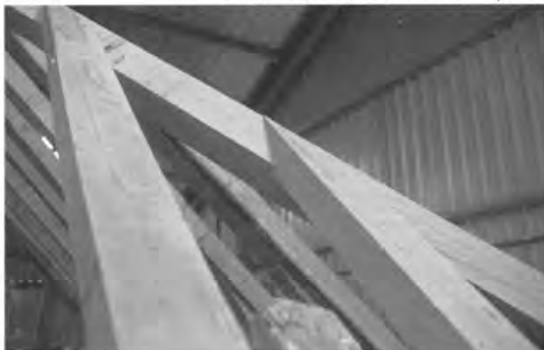
Views of the reconstructed pre-Georgian hip. Old timber at the bottom is an end-wall tie-beam. Hip is laid in plane with one of the meeting roofs, jack rafters in the adjacent roof are scribed and bird's-mouthed.
