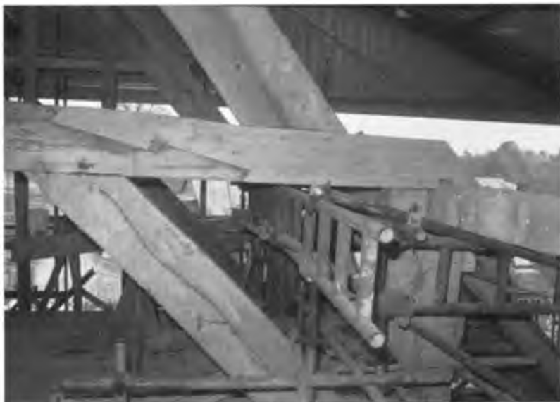
Finished repair to a tie-beam...
