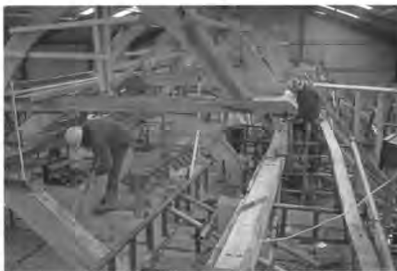
View South along the west arcade plate. The barn has been covered by a temporary steel shed for the duration of the repairs.
