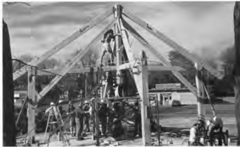
The other cardinal "bents" hold the first in place.
