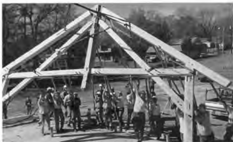
First bent goes up with tackle and poles.
