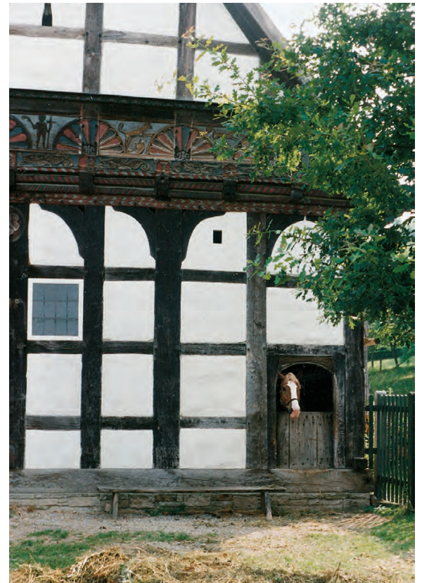
(5) Dutch barn displaying carved infill and short bracing (open air museum at Detmold, Nordrhein Westfalen).
