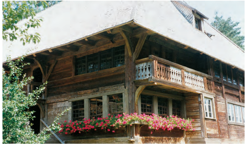
(2) Allemanic combination of log and frame construction (open air museum at Neuhaus ob Eck, Baden Württemberg).
