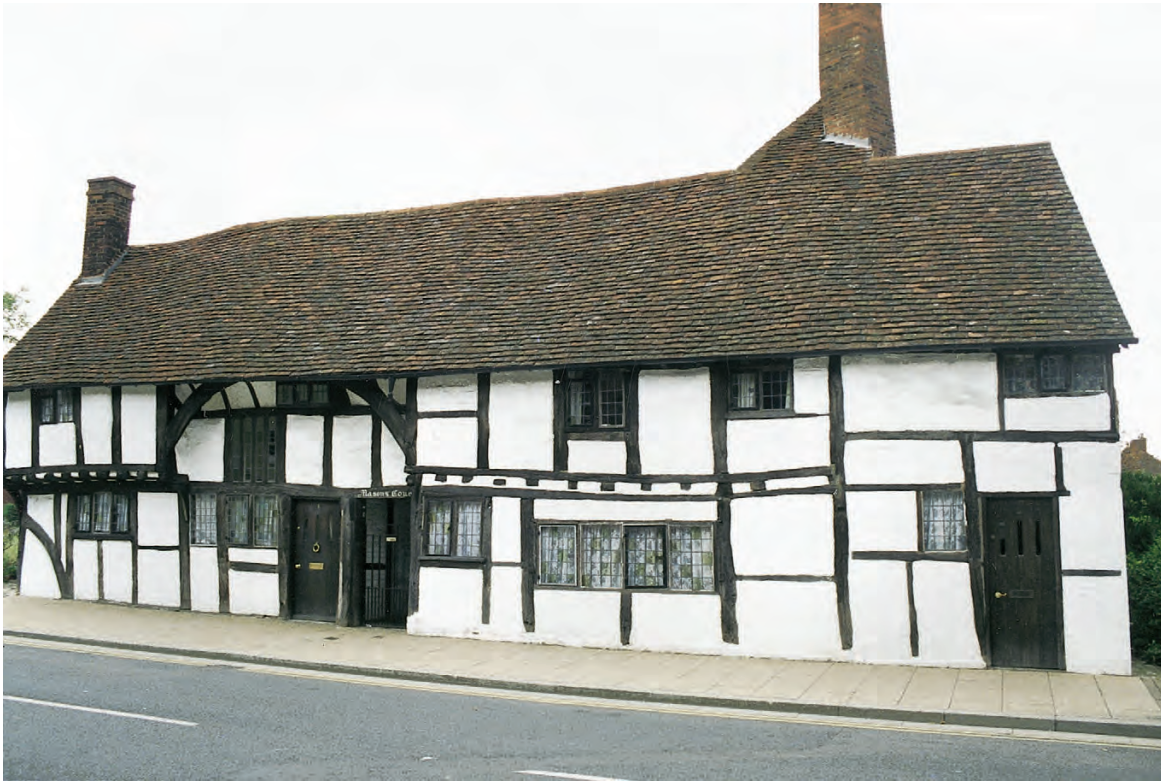
Above, herringbone strutting in Warwick. At left, Mason's Cove, a Wealden-style house with recessed front and square panels.
