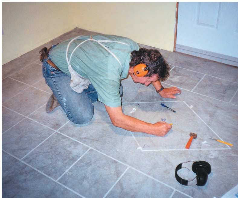
Floor craftsman Chris Bartsch acid-etching the floor in the front hall.
