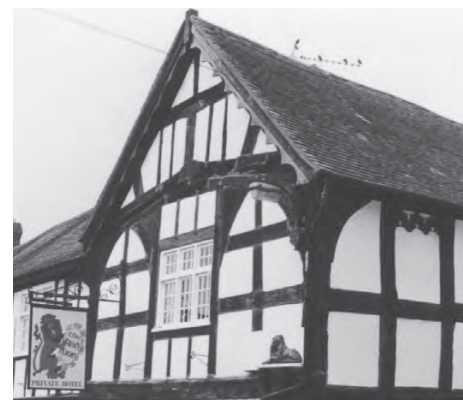
Hereford-style roof framing.
