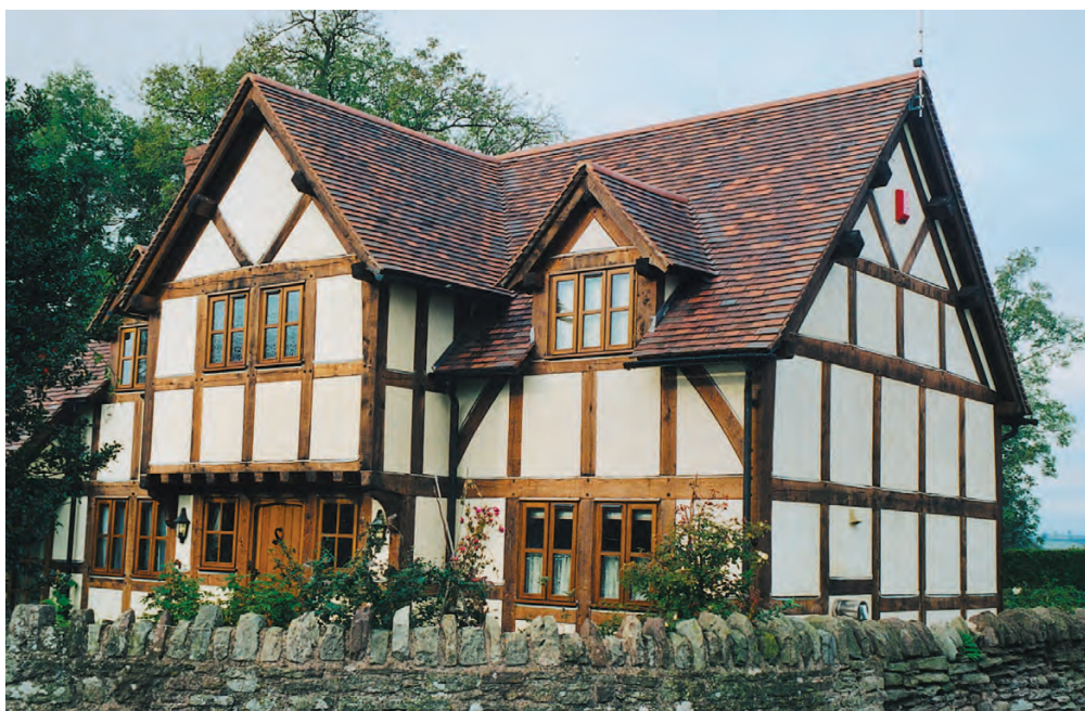
Modern timber-framed house by Border Oak. Infill is specially designed for the weather.
