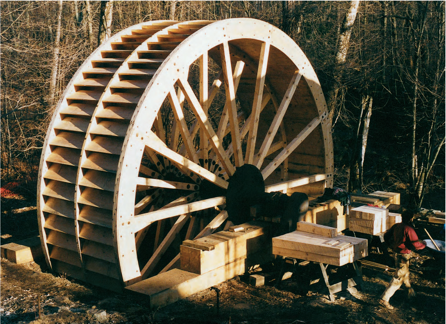
Long Pond Iron Works 24-ft.-dia. water wheel, reconstructed in 1994 from the remains of a double wheel at a Civil War blast furnace site at Hewitt, New Jersey. The crank arms at each end of the shaft drove pistons to provide the draft for the furnace, of which nothing remains save the foundations. Below, Rondout's Bruce Murray removing the substantial iron shaft and hubs.
