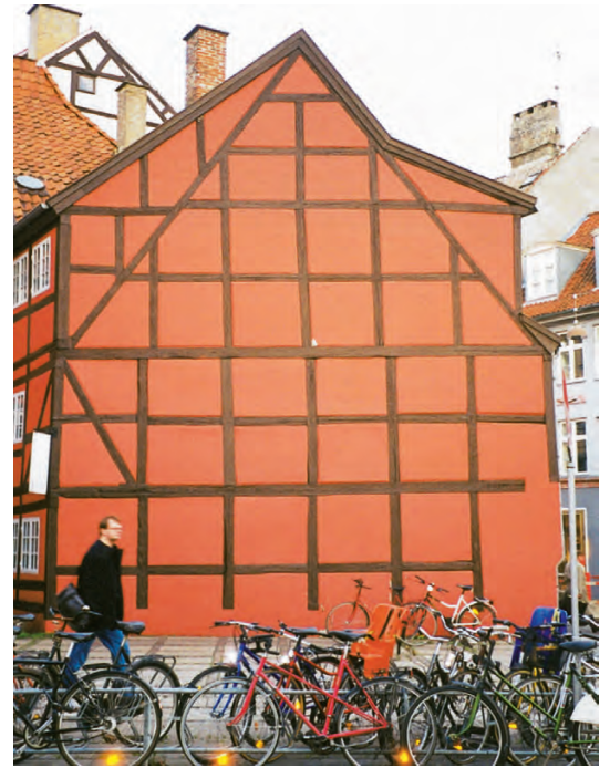
Above, brick-infilled timber frame in Malmö shows mix of short and long timbers, as well as typical projections of upper story floor framing, including ties and tying joists. Note healthy wooden sill at base of wall. Above right, house in Copenhagen whose wooden sills have been replaced with masonry, yielding the peculiar floating look. Below left, Malmö's buildings generally run eave (or wide) side to the road, unlike other urban buildings in northern Europe. Bottom left and below right, tying joists and supports for jettied overhang pierce the walls.
