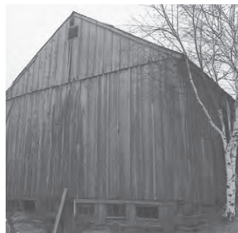
Boarding lapped at tie beam.
