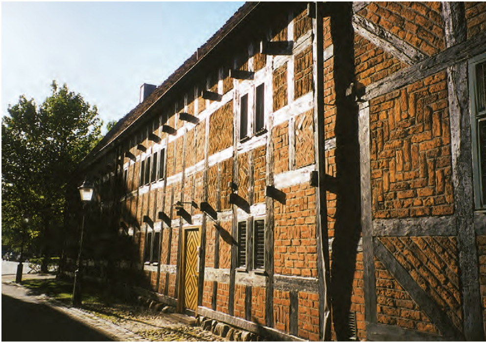
Above, brick-infilled timber frame in Malmö shows mix of short and long timbers, as well as typical projections of upper story floor framing, including ties and tying joists. Note healthy wooden sill at base of wall. Above right, house in Copenhagen whose wooden sills have been replaced with masonry, yielding the peculiar floating look. Below left, Malmö's buildings generally run eave (or wide) side to the road, unlike other urban buildings in northern Europe. Bottom left and below right, tying joists and supports for jettied overhang pierce the walls.
