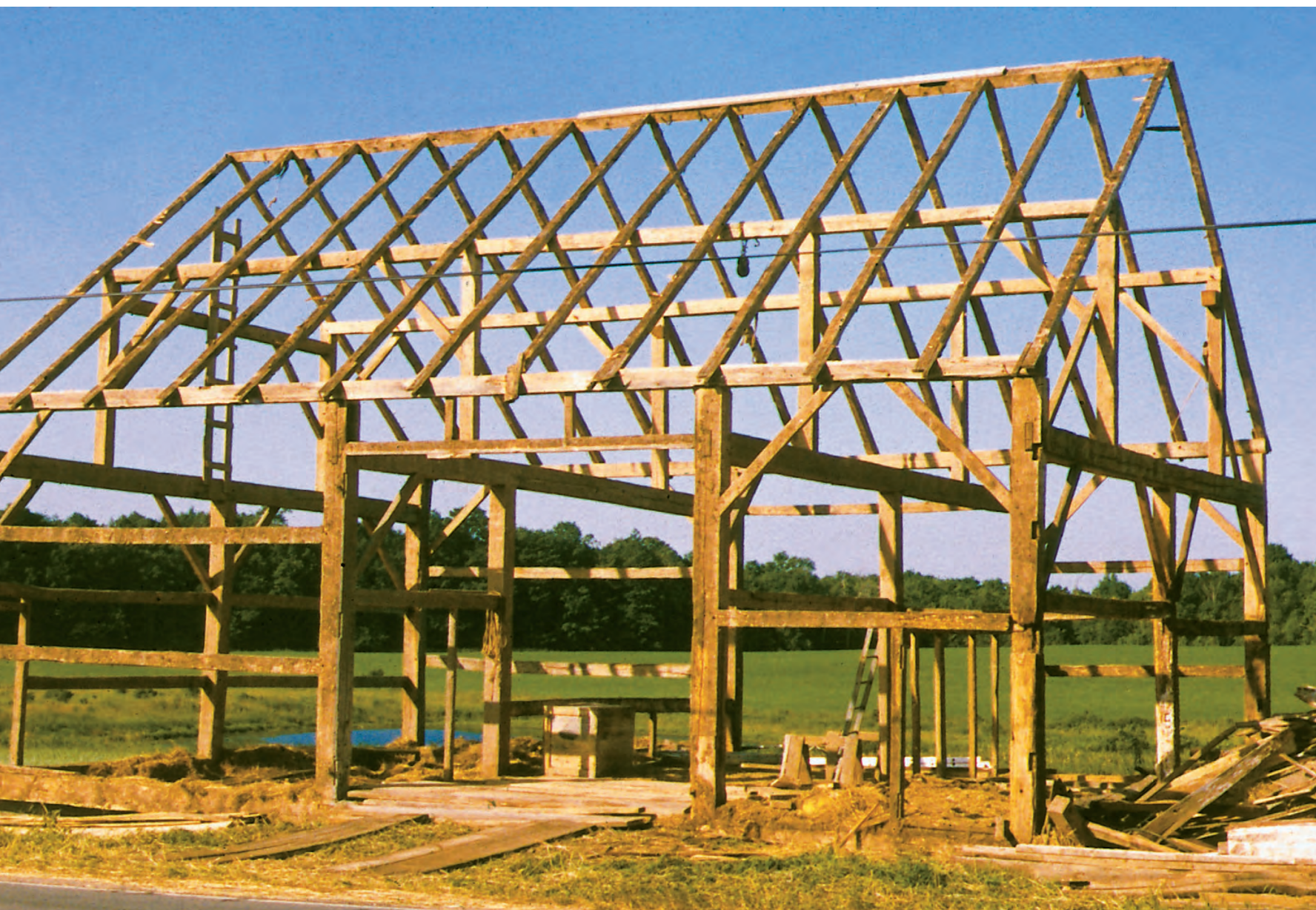
Central New York State barn, with typical dropped tie beams and purlin plates supporting the rafters. See TTRAG 2000, page 16.
