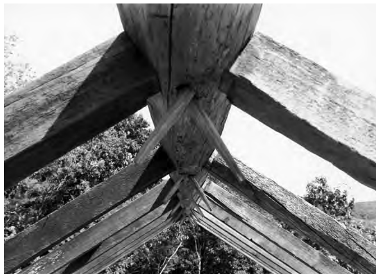
View down the ridge beam of a mid-19th-century 40x50 barn in Hinsdale, Massachusetts. The 3x4 rafters have barefaced tenons.
