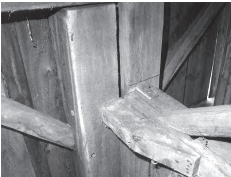
When the builder added to this barn in Savoy, Mass., he saved on a new 30-ft. tie beam by framing a piece into the post and pinning and nailing it to the existing barn's tie beam. Notice how the end is hewn down to permit better nailing.
