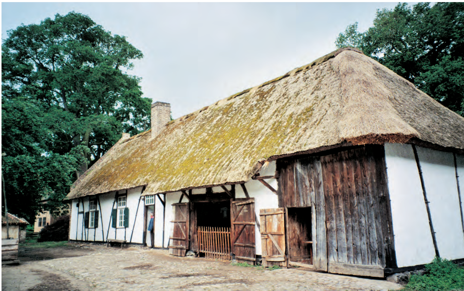
A typical Campine region long farmhouse. House to the left, barn to the right. Campine framing spreads the posts, adds full-height braces.
