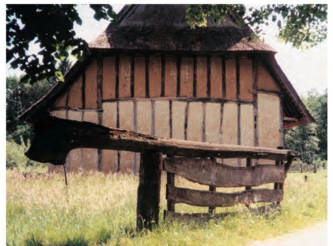
A barn built in regelbouwtechniek , or Flemish half-timbering, which appears to have evolved from Scandinavian wall construction in solid upright timbers. Above, view of barn gable end and farm gate cunningly counterweighted by the butt end, complete with roots, of a log rail.
