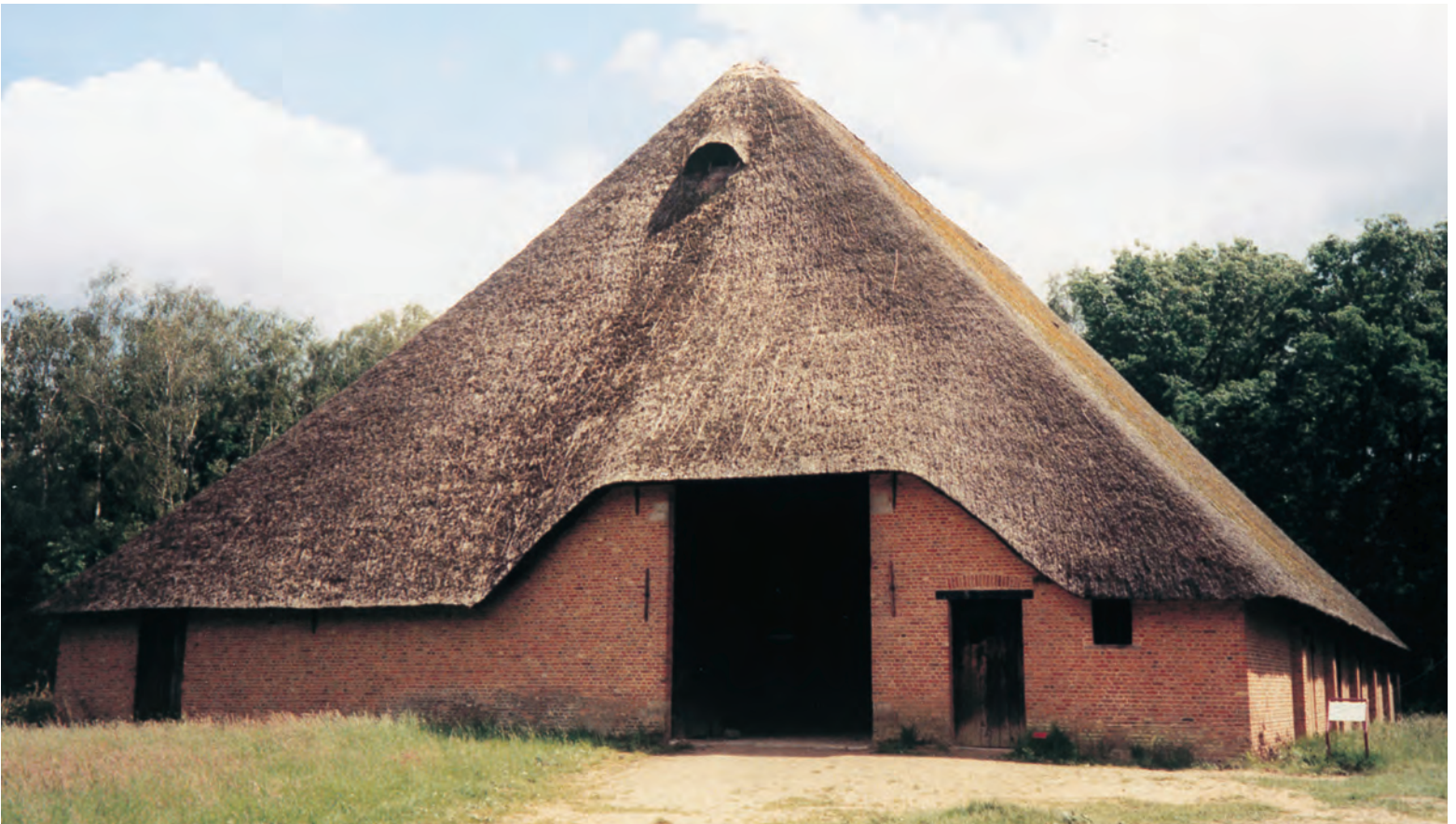
A square mikke barn with masonry walls, pyramidal thatched roof and central aisle entrance.
