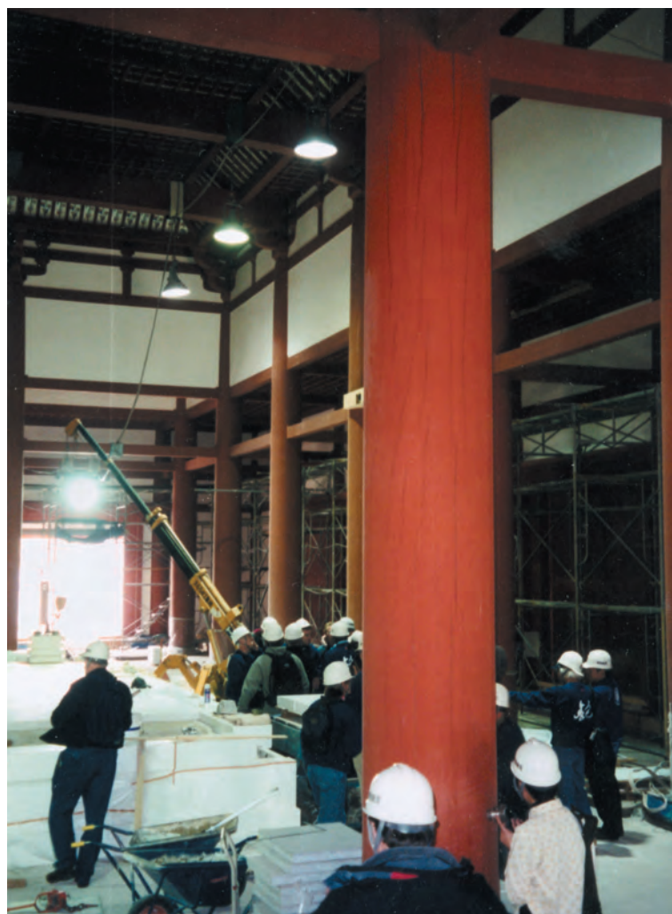
Views of the Lecture Hall at Yakushiji. A colonnade of painted exterior posts, all on a slight batter to counter the thrust of the roof, surrounds the exterior. Inside, some timbers and other surfaces are decorated with iron oxide paint. Most timber is hinoki cypress imported from Taiwan.
