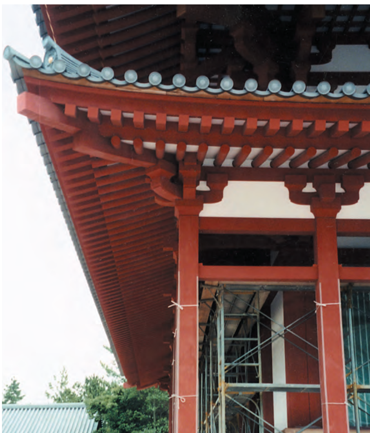
Views of the Lecture Hall at Yakushiji. A colonnade of painted exterior posts, all on a slight batter to counter the thrust of the roof, surrounds the exterior. Inside, some timbers and other surfaces are decorated with iron oxide paint. Most timber is hinoki cypress imported from Taiwan.
