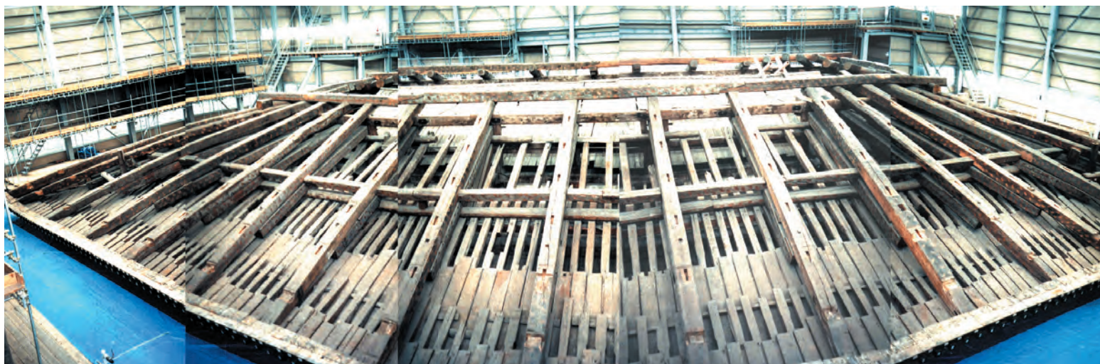
Author's photomontage giving fish-eye view of lower roof system at Toshodaiji, originally built 759, last modified around 1800.
