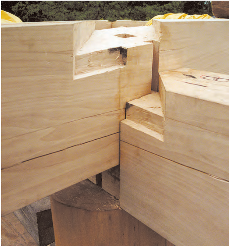
The two plates (keta) partly assembled, seen from outside. The slope of the seat line on the face of each plate is at half the common rafter pitch. On the left-hand plate above, it rises from left to right and is mirrored on the right-hand plate. Analogous lines bound the rear faces of the seat.
