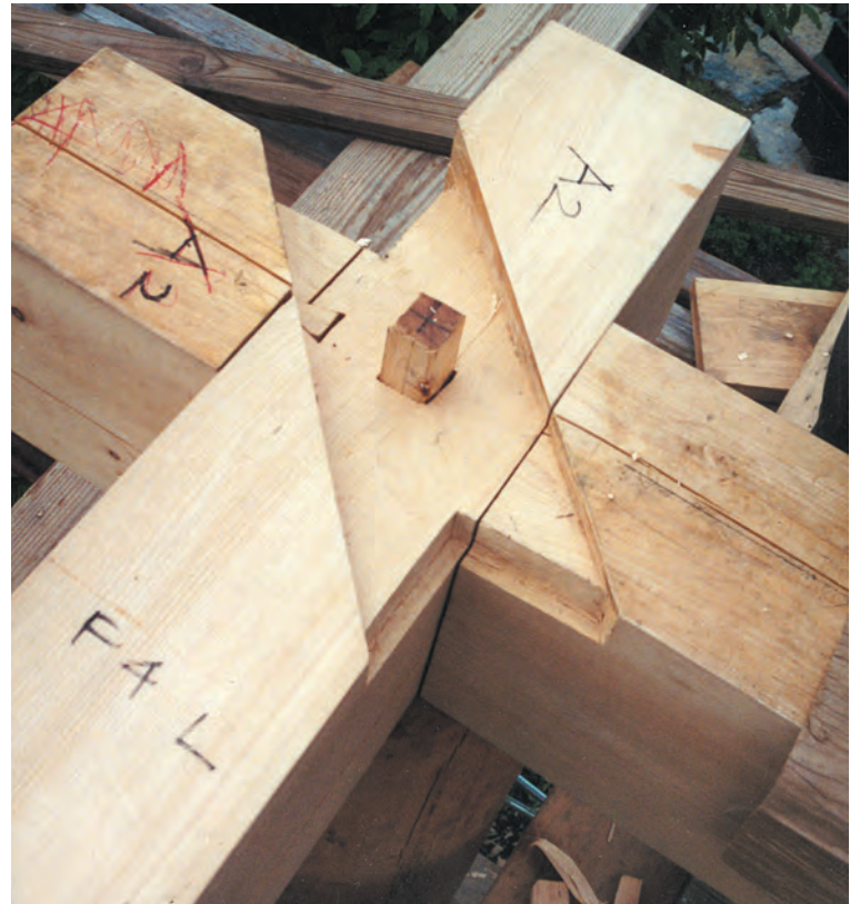
The joint assembled, seen from inside. Though the hip is firmly registered by the rabbets at the inside and outside corners of the joint, the tenon rises from the post through both plates and enters the hip for good measure. The dovetail connection probably serves mostly as a spline.
