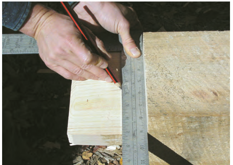
Framing square yields traditional peg center distances from shoulder.
