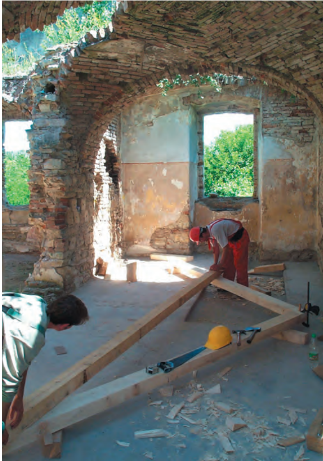
At left, students lay a scissors brace on top of two principal rafters already positioned over the chalk lines.
