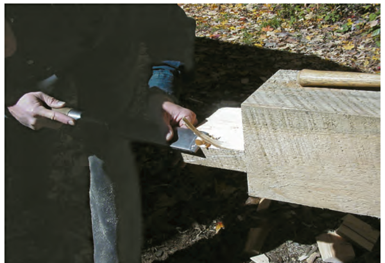
First step in trimming the cheek is to establish the edges.
