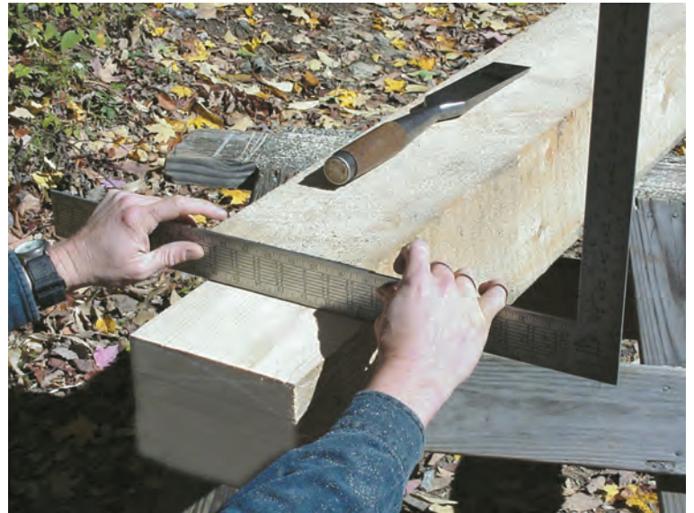
Checking for flat across the cheek.
