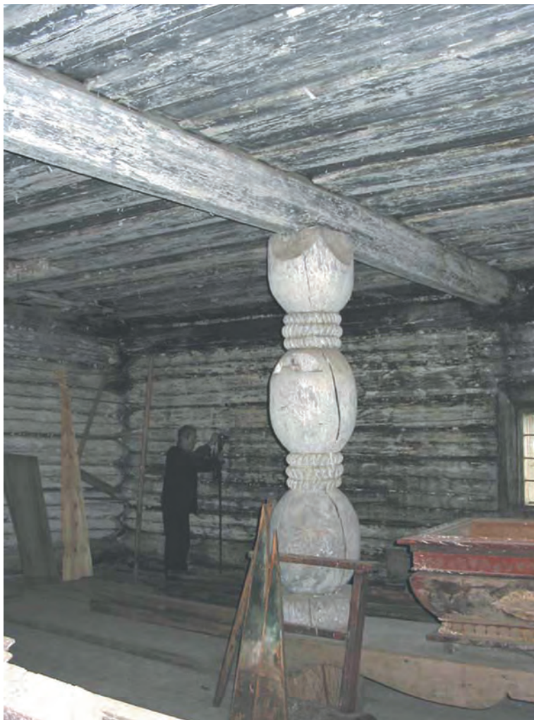
Large (18-in.-dia.) interior columns at the Church of the Protection of the Virgin near Kargopol. Ceiling above is framed with closely spaced joists grooved to receive plank infill; surface texture echoes the log walls. Bulbous turnings, possibly shaved, are unusual. The three laces of rope at each neck are carved. On the story above, columns in corresponding positions are cased as paneled pilasters, in a style more appropriate to the mid-18th-century period of the building.
