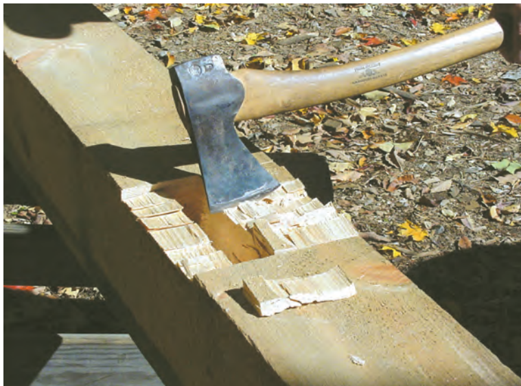
Removing housing waste with an axe.
