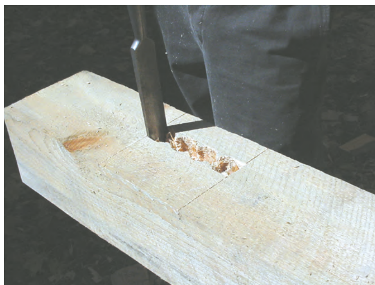
Squaring up the end of the mortise after boring out waste. Full depth is achieved incrementally by alternating between mortise ends and sides.
