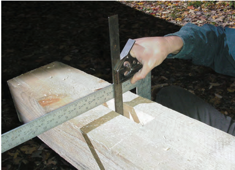
Checking for plumb mortise sides when top surface is not square to adjacent reference surface.
