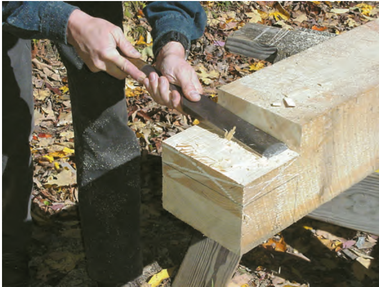
Cross-grain paring levels the surface between the prepared edges.
