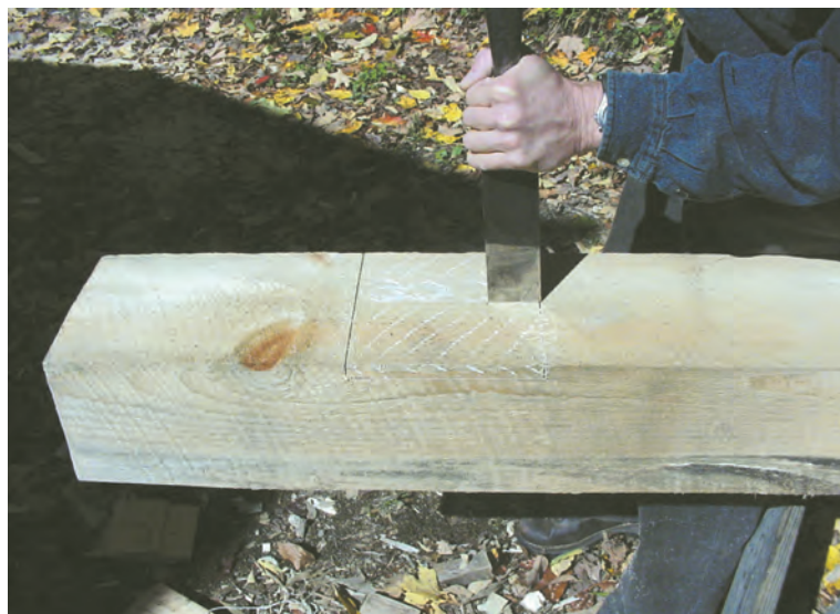
First steps for a housed mortise are to sever the ends and score the sides.
