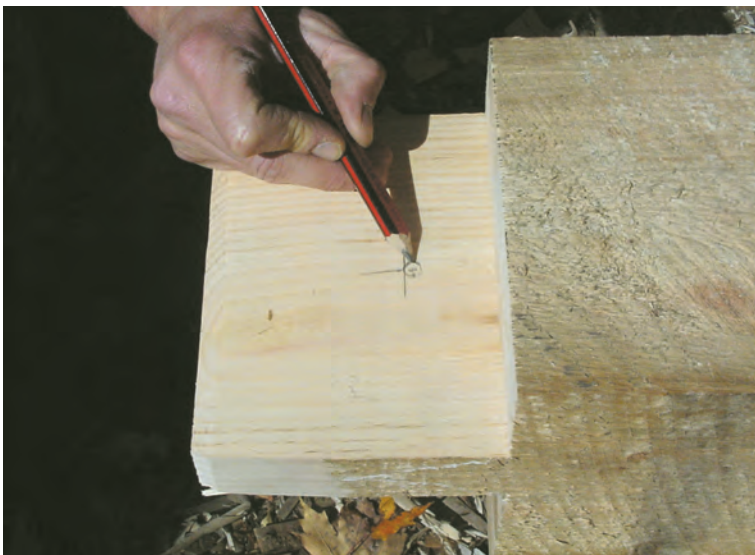
To draw and keep a simple mortise and tenon joint together, the peg hole for the tenon is deliberately offset toward the shoulder of the joint.
