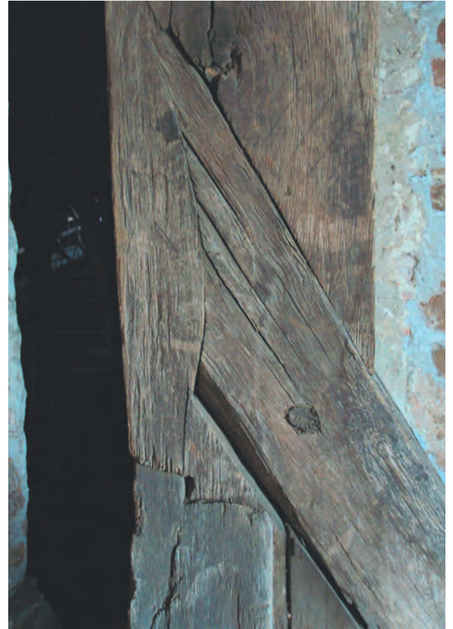
At right, lap joint with curved end seen in the roof framing of the ancient church at Sighisoara. Joint has remained tight for 500 years.
