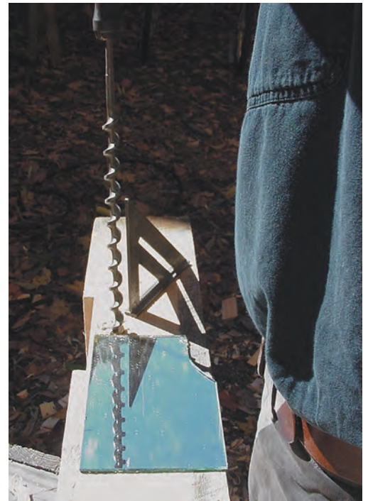
Peg hole drilling plumb, with timber on its side. Some workers find it easier to hold the long drill level, with the timber right-way-up and the mortise in view.
