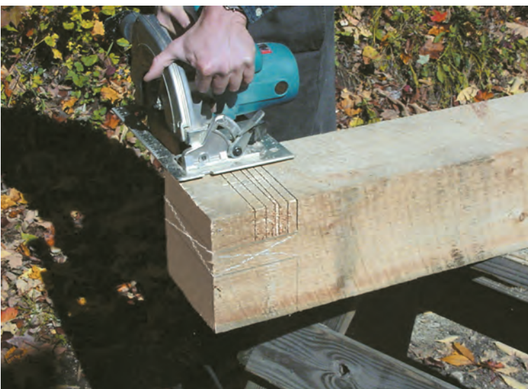
Kerfing the waste on a tenon cheek. Many kerfs make for easy chipping.
