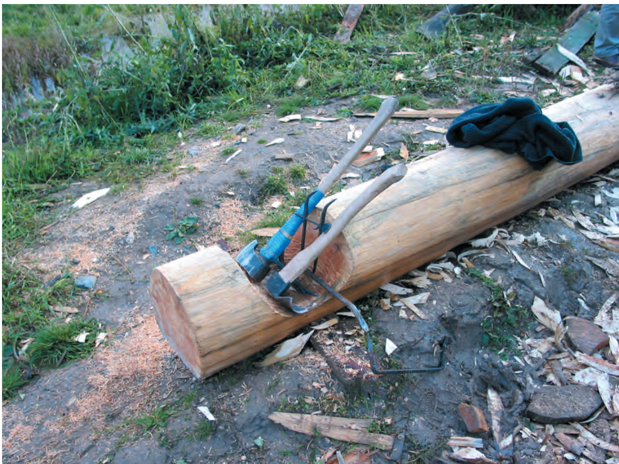
Completed corner notch housing tools of the trade except for the timesaving chainsaw. Bluestain in pine appears to be a problem even at far northern latitudes.
