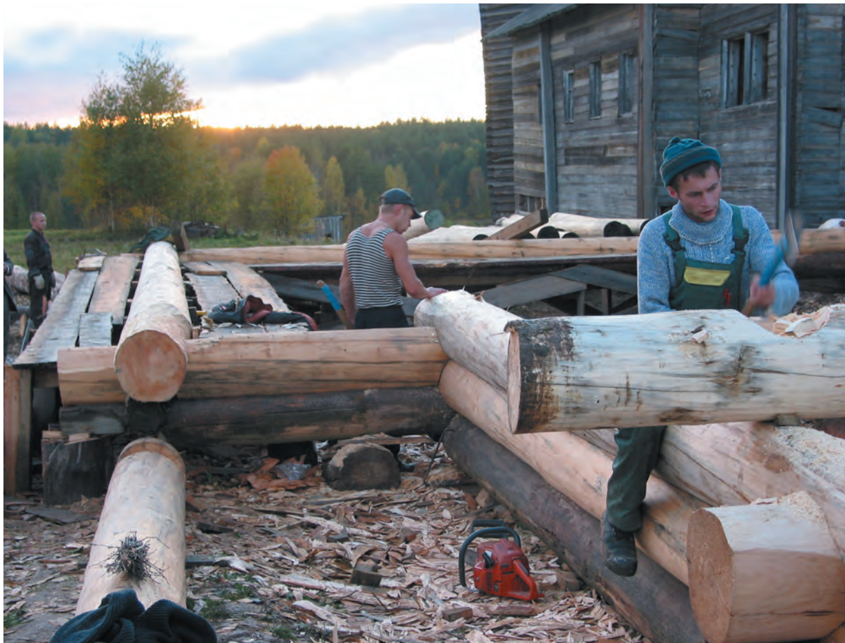
Russian logbuilders preparing corner notches for replacement logs at the Church of Christ's Holy Tree in Filipovskaya. Axe is used to remove nearly all the waste after kerfing with chainsaw. In a separate operation, logs are full-scribed in length on their lower surfaces.
