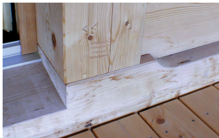
Door header labeled as fitting ninth post, first wallframe, first story (second floor US). Below, second story post number 4, crossframe location indicated by just-visible single flag near center of uppermost stroke.
