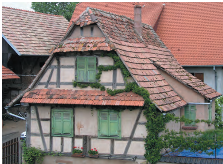
Small traditional Alsace house, half timbered, with tiled, jerkin-head gable roof and pendants over the gable windows, at the Ecomusée d'Alsace in Ungersheim.
