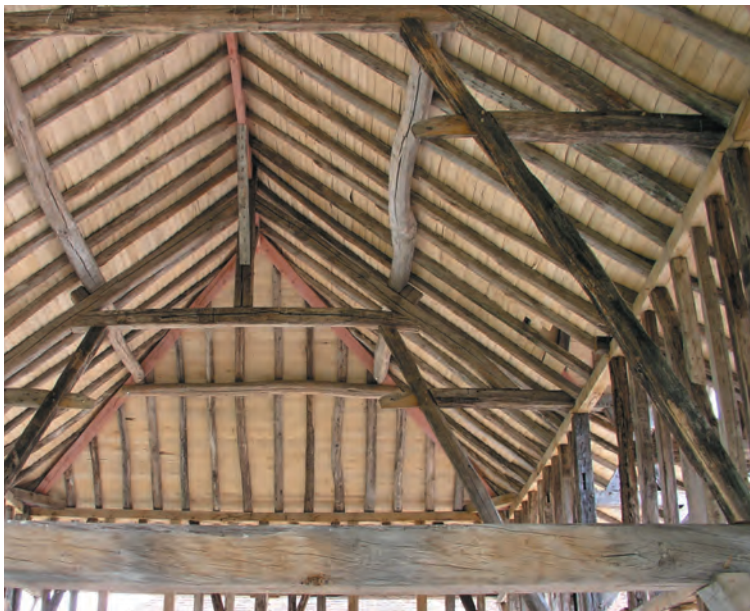
Newly framed structure, Montreuil, using old and new timbers, the latter painted for yet more contrast. Note legs of strength to carry roof loads down from collars to tie beams, thus dissipating much rafter action.
