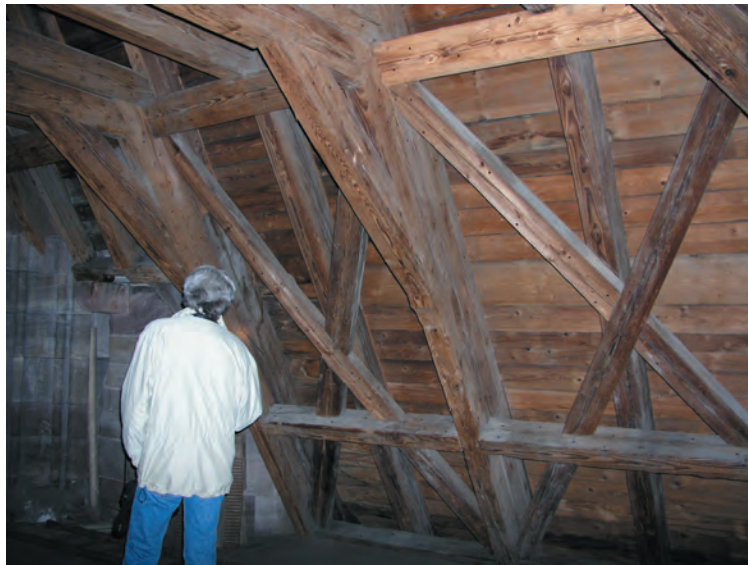
Softwood Liegenderstuhl (lying chair) trusses and heavy longitudinal X-bracing support the framing of the weather roof of Strasbourg Cathedral. Such German-style framing prevails in Alsace.
