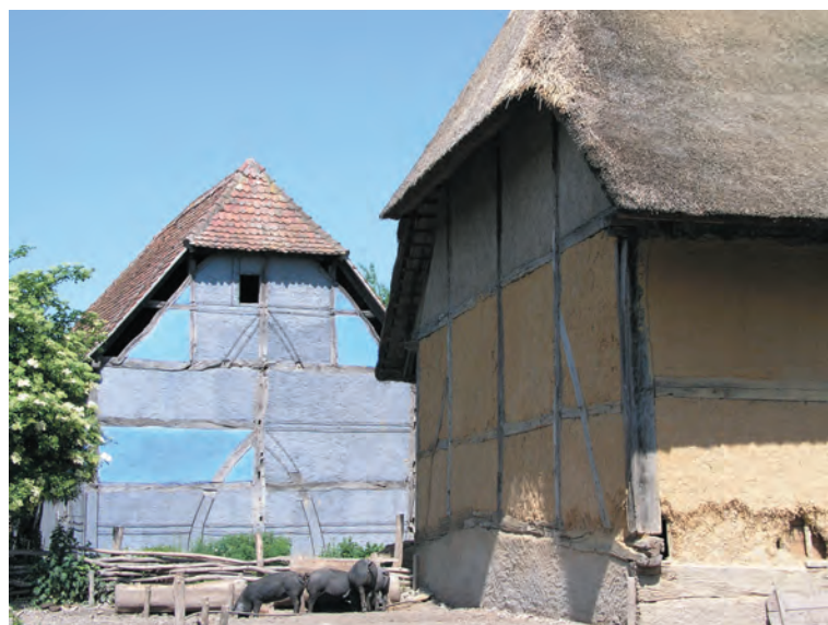
Parti-colored wattled-and-daubed barns at the Ecomusée d'Alsace, with outlined timbers. Note typical jerkin-head roof, with truncated ridge to allow a short hip that gives some protection to the gable end.
