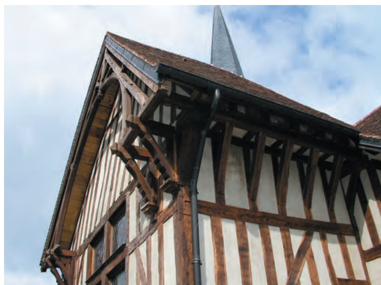
Church of St. Julien and St. Blaise, Longsols, originally 15th century, recently restored. The framed gable end overhang with carved double brackets and arch braces shows the possibilities of the framer's art before structure and decoration were disconnected by the Renaissance. Interior shown overleaf.
