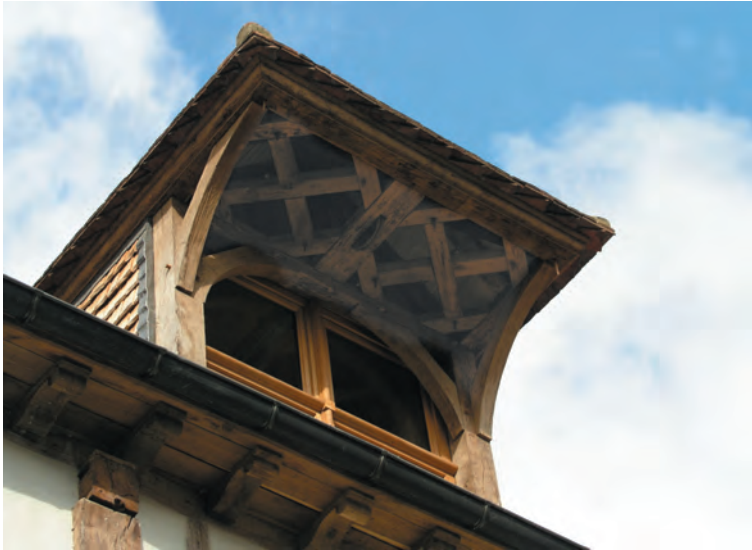
Substantial dormer at Troyes, so heavily framed perhaps to support loads brought up on the pulley just visible at the center of the overhang. Lead flashing shields the thick edge of the tile siding.
