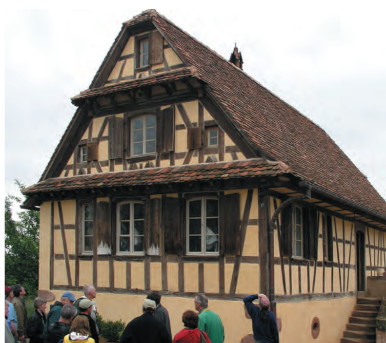
New Alsatian house in Ochfelden built in traditional style but using straw-clay brick infill and straw batt insulation, demoed below by a delighted Dave Carlon.
