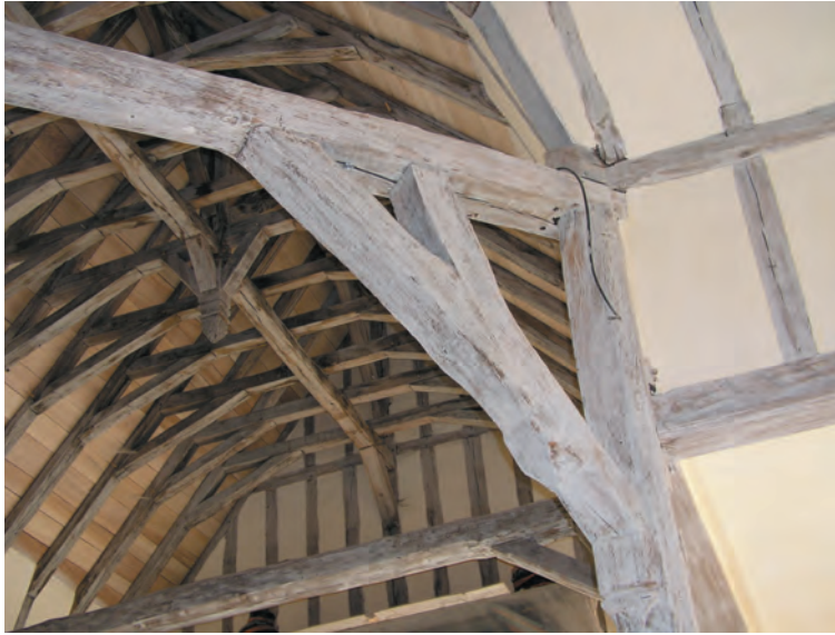
St. Julien et St. Blaise, Longsols, 15th century, restored. Some of these old timbers are newly placed.
