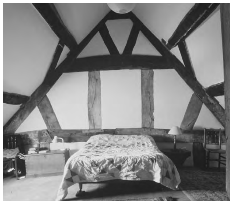
FIG. 24. ROOF TRUSS BRACING AND TIMBER PLACEMENT.
