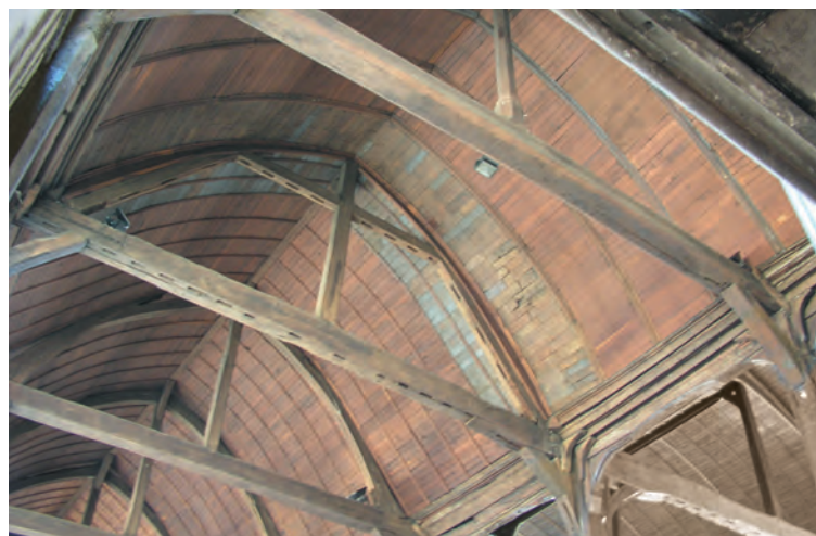
Fig. 12. One of two vaults at Ste. Catherine's. Empty mortises, patched lambrissée and change in rib centers indicate historic alteration.
