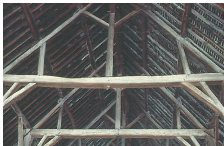
Fig. 3. Market hall, Milly-la-Forêt, 1479, with three-aisle basilican layout and double-framed "Latin Truss" roof with multiple purlins.
