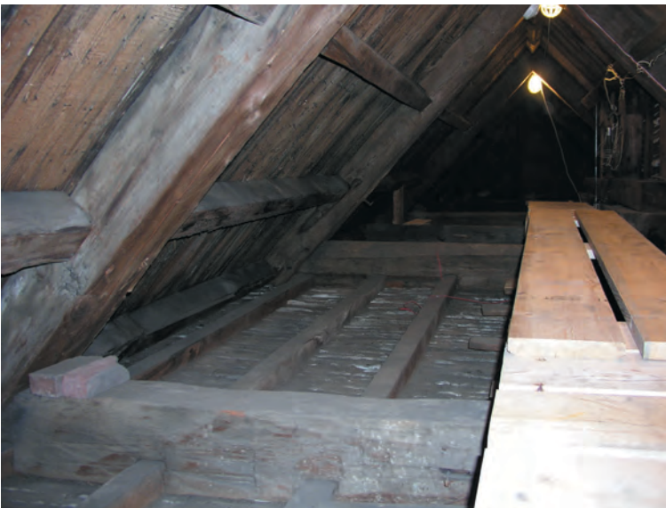
View under one side of the M-roof, with heavy collar beams carrying ceiling joists for the chambers below. Catwalk gives access to area seen in photo below.
