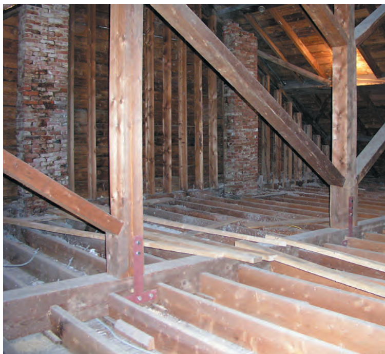
Lower part of truss. Toe-nailed 2x8 joists pass under the tie beams to set lath 2 in. below ties. Long-serving tension joints have been reinforced.
