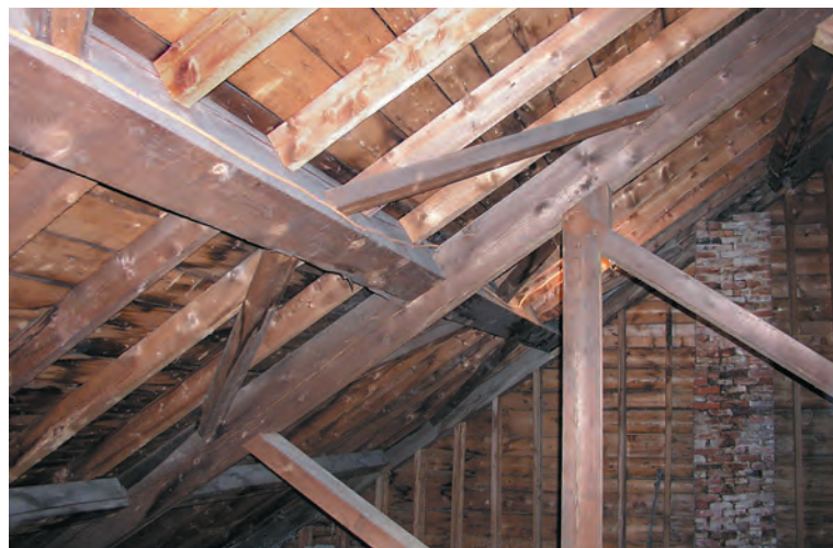
Huntington, upper part of truss with struted princepost. Wind-braced principal purlins overlap the upper chords and connect the trusses.
