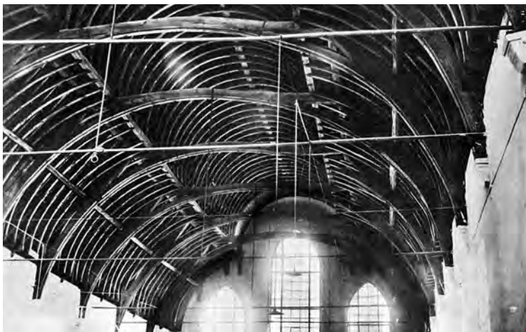
Fig. 8. Trefoil roof design of the main ward of the Cistercian hospital of Byloke in Ghent, dated by dendrochronology to 1255. The roof type is an aisled-hall derivative composed of "short principals" and resembles base crucks that developed in England and the Low Countries during the 13th century. The east end retains some of its original paneling or lambris; the tie-rods and corbels date to the 17th century.
