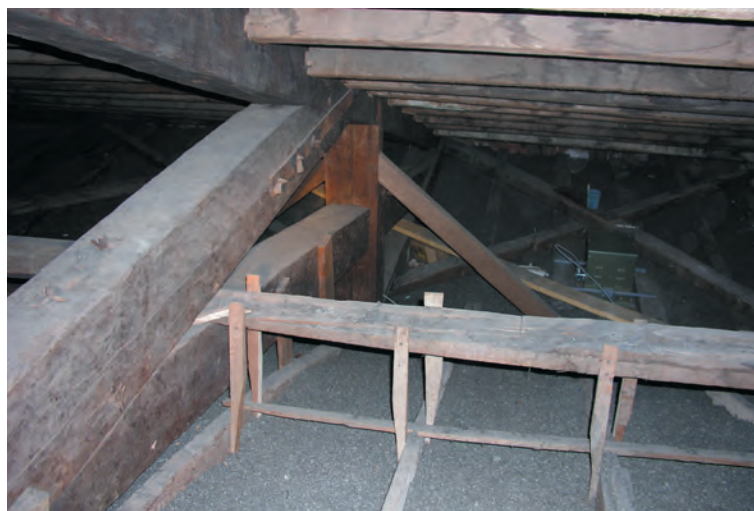
Under the roof at St. John's, curved ceiling joists are hung by wooden staves. Note forelock-bolted iron strap binding collar beam to rafter.
