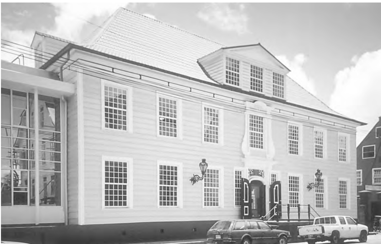
The Cellier house restored to its old glory. Modern fireproof structure to left replaces wood-framed infill.
