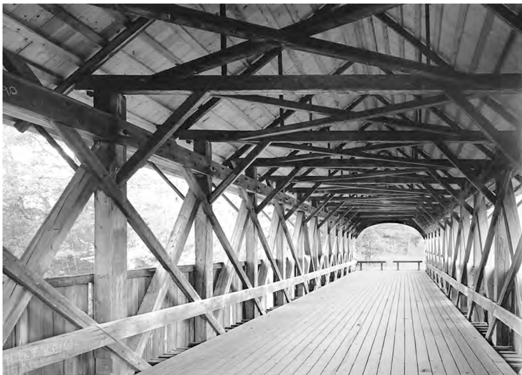
Fig. 2. The Paddleford truss. Sunday River Bridge, Newry, Maine, built by Hiram York, 1872. Note substantial guard rail, not functionally part of the truss. Photo 2004.
