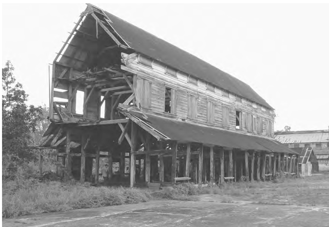
1808 coffee barn at Peperpot estate. Three aisles, closely spaced crossframes, no joists between the ties.
