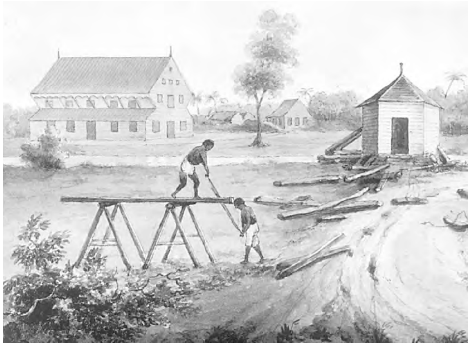
Resawing timber at a building site, ca. 1850 (detail of drawing by Huygens, ca. 1850).
