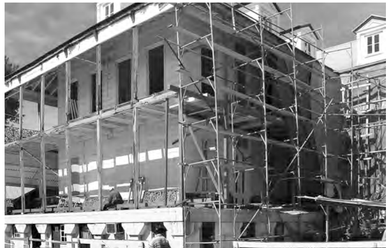
Repair and replacement of galleries on the 1865 hospital building. A projecting canopy will be added to provide further protection.
