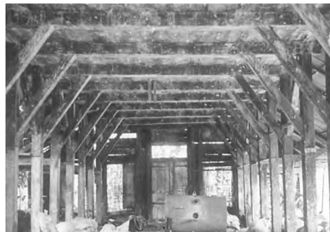
Floorboards are applied directly to crossframes of coffee barn.
