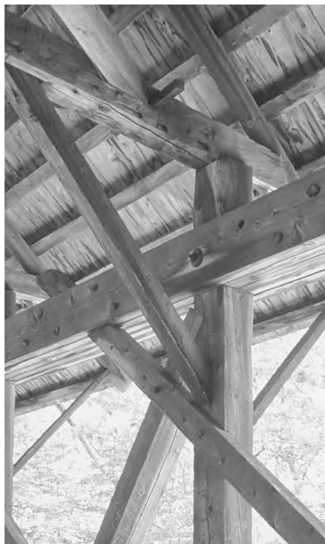
Fig. 3. Paddleford bridge at Groveton, New Hampshire, built by Captain Charles Richardson in 1852, showing typical framing details in the system. This bridge is somewhat the worse for wear, having served heavy traffic on US Route 3 until 1939. It was stabilized by Milton S. Graton in the 1960s and has outlasted its steel replacement. Note the four-part top chord with a space in the middle and the truss ties lapped through each face of the inboard chord laminae. Where the chord passes a post, the bearing shoulder is hidden because the second lamina in has been reduced in height. Note also the lock notch at the end of the tie beam to keep the rafter from slipping off. Photo 2004.
