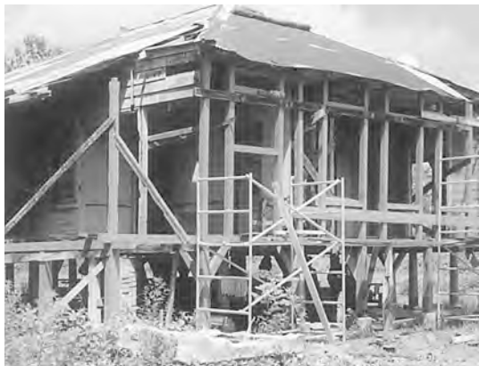
At work in 2001 on the 19th-century frame of the Frederiksdorp doctor's house, stripped of overhangs and gallery. At right, house fully restored in 2003.
