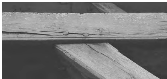
So-called toognagel joint between brace and beam. One pinhole is bored straight across, the other strongly draw-bored.
