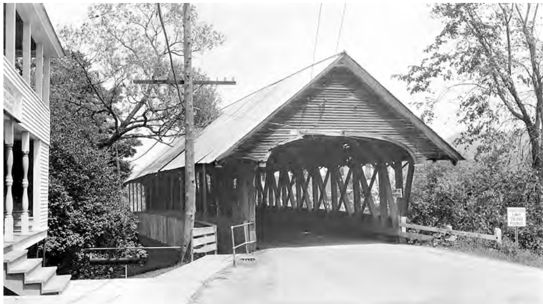
Fig. 5. Typical Paddleford style portal on the former Stevens Village Bridge, Barnet, Vermont. Photo by Henry A. Gibson, 1948, from the archives of the National Society for the Preservation of Covered Bridges.
