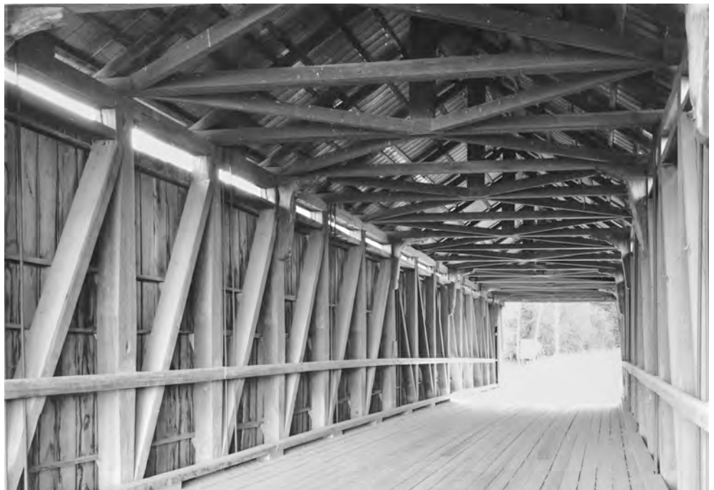
Fig. 1. Multiple kingpost truss bridge at Eaton, Quebec. Vertical rods are later additions. Guard rail (or strake) about a third of the way above the floor is not part of the truss. Photo 1994.
