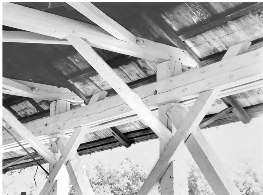
Fig. 3. Paddleford bridge at Groveton, New Hampshire, built by Captain Charles Richardson in 1852, showing typical framing details in the system. This bridge is somewhat the worse for wear, having served heavy traffic on US Route 3 until 1939. It was stabilized by Milton S. Graton in the 1960s and has outlasted its steel replacement. Note the four-part top chord with a space in the middle and the truss ties lapped through each face of the inboard chord laminae. Where the chord passes a post, the bearing shoulder is hidden because the second lamina in has been reduced in height. Note also the lock notch at the end of the tie beam to keep the rafter from slipping off. Photo 2004.
