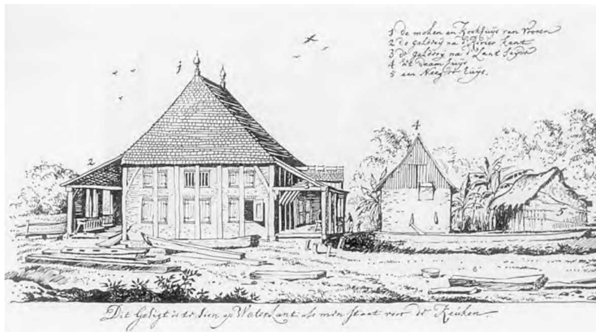
Early sugarmill (1707) at Waterland estate, with high hip roof, exposed frame and long corner braces. Drawing by Jean-Louis Volders after the original by Dirck Valkenburg.
