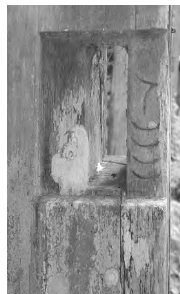
Assembly mark within joint.
