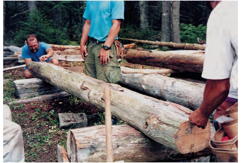
Fig. 6. Striking centerlines joining plumb and level lines on log-ends. Bumps in surface can sometimes require segmental striking.
