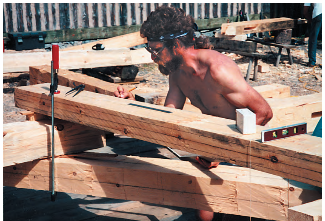
Fig. 4. Marking for joints in multiple member assembly. Timbers have been stacked in the proper orientation and carefully leveled with shims, then clamped to keep them from shifting. Upper member has been both centerlined and joint lined, lowest timber centerlined only.
