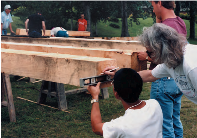
Fig. 5. Level-lining square timbers at the ends preparatory to striking connecting lines on faces. Objective is to describe a true plane.
