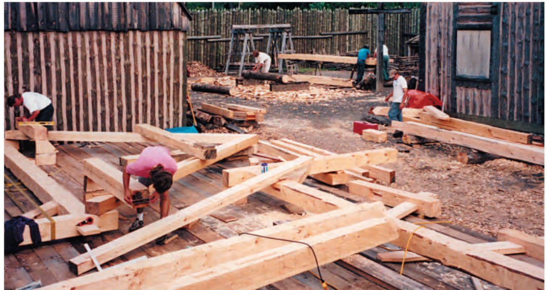
Fig. 2. Square rule assemblies (above left) show abrupt gains and reductions at many joints. Scribe rule assemblies (right) appear to flow together.
