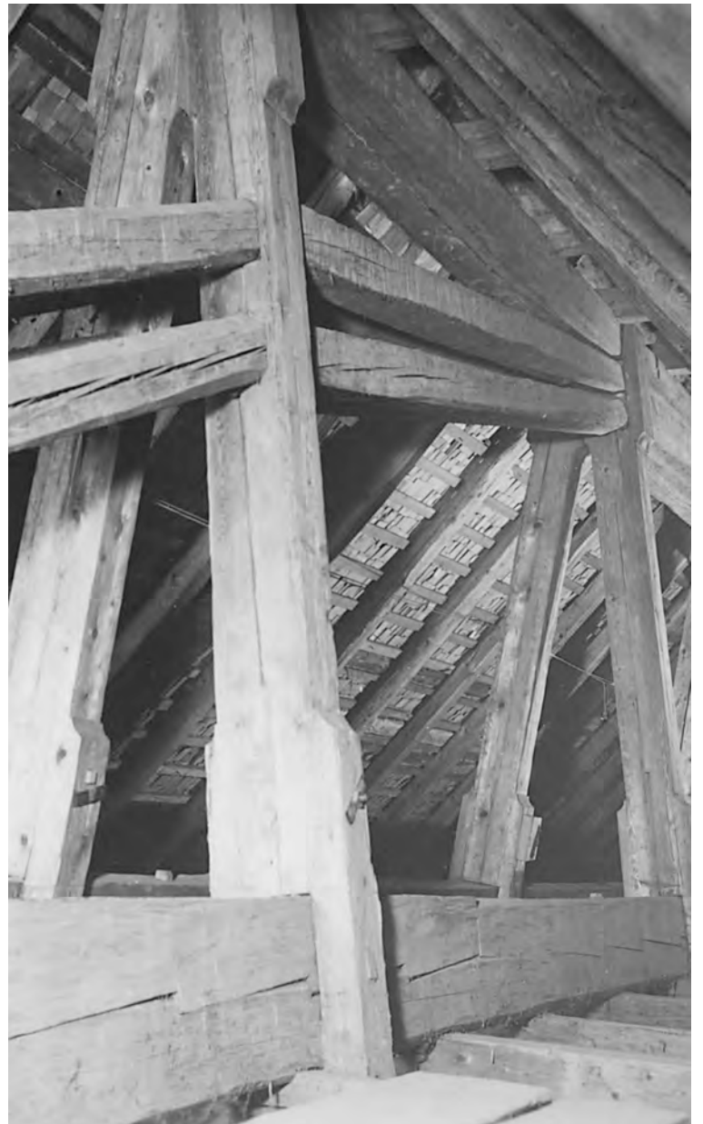
Fig. 2. Lengthwise truss, Reformed Church at Grub, Switzerland, 1752.
