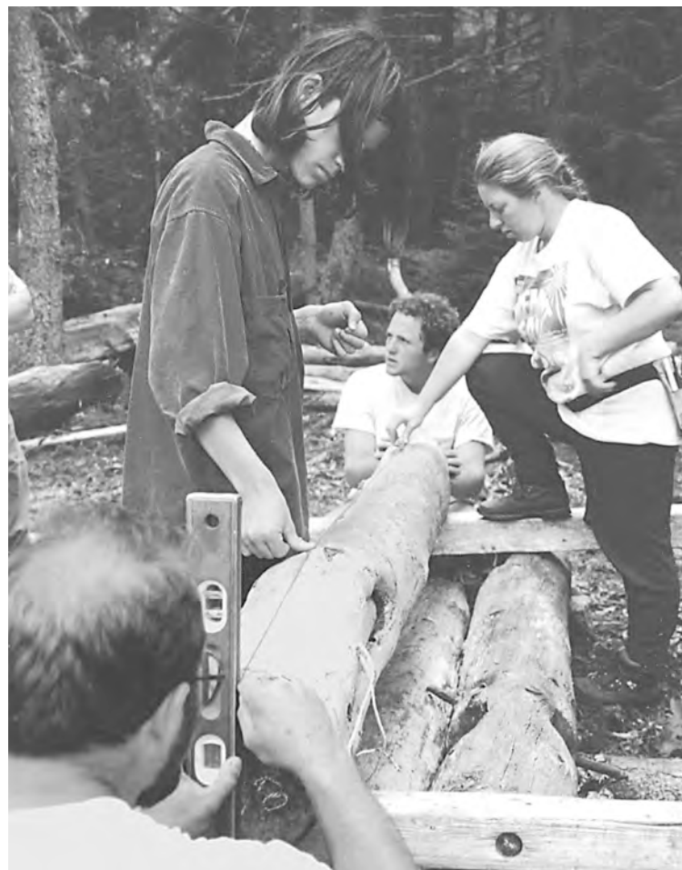
Fig. 13. Snapping a chalk line in segments on a bumpy surface.
