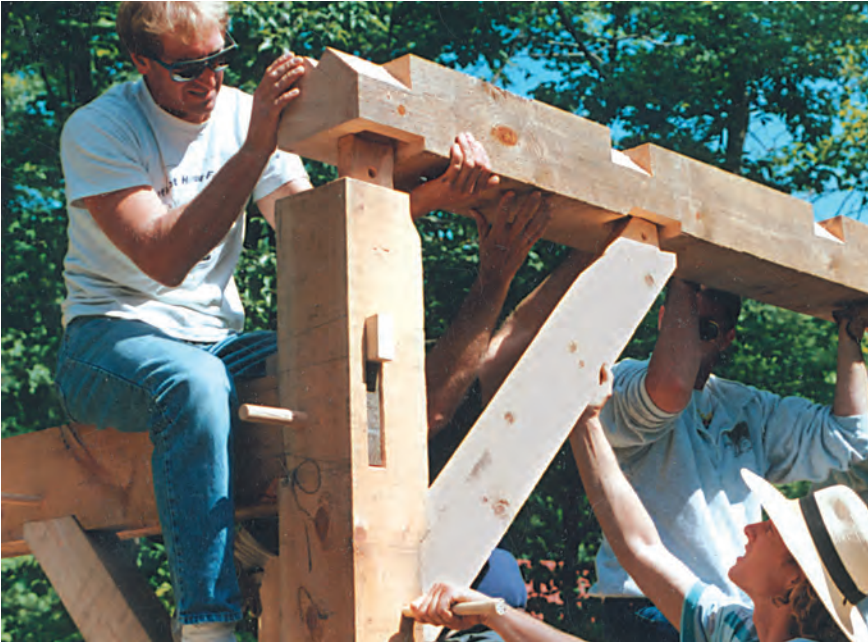
Fig. 2. Square rule assemblies (above left) show abrupt gains and reductions at many joints. Scribe rule assemblies (right) appear to flow together.
