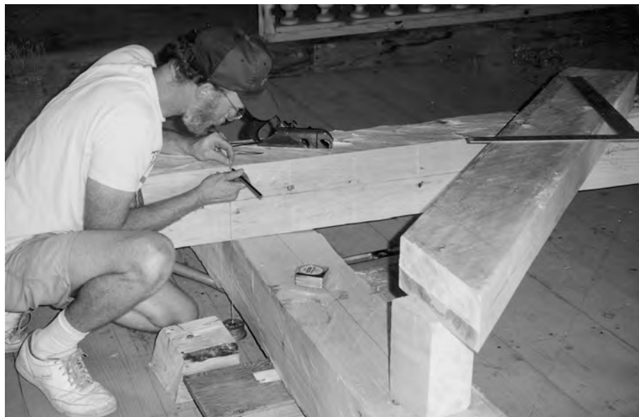
Fig. 18. Scribing assembly for post, beam and brace at St. Marie-among-the-Iroquois. Main timbers are lined. French method includes floor layout lines and cast plumb bob with flat bottom. Small rabbit plane cuts flats across the grain of hewn timber to produce level reference stations or "feather marks."
