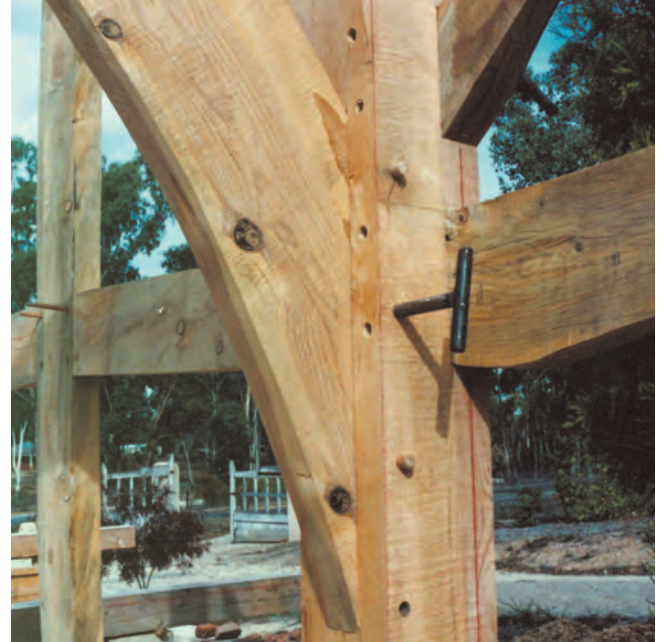
Fig. 2. Square rule assemblies (above left) show abrupt gains and reductions at many joints. Scribe rule assemblies (right) appear to flow together.
