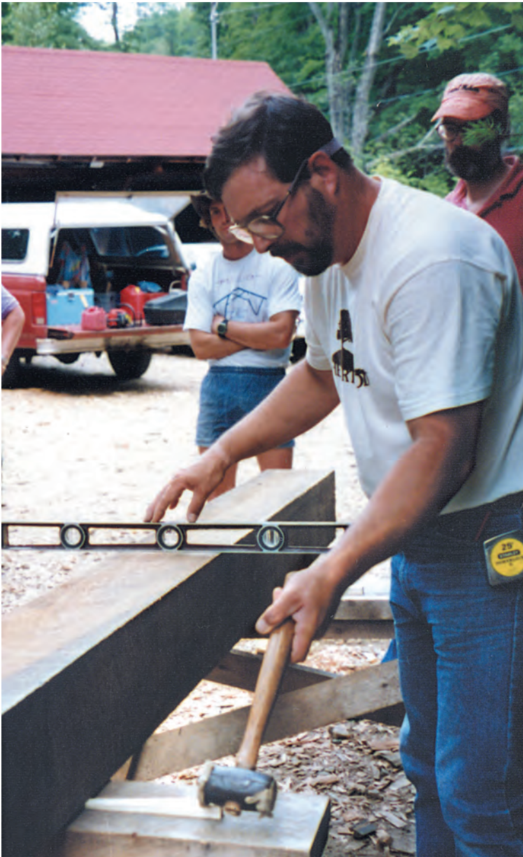
Fig. 9. Dave Carlon tapping up the wedge to tilt a timber surface into level. Area under level will be hatched for later reference.
