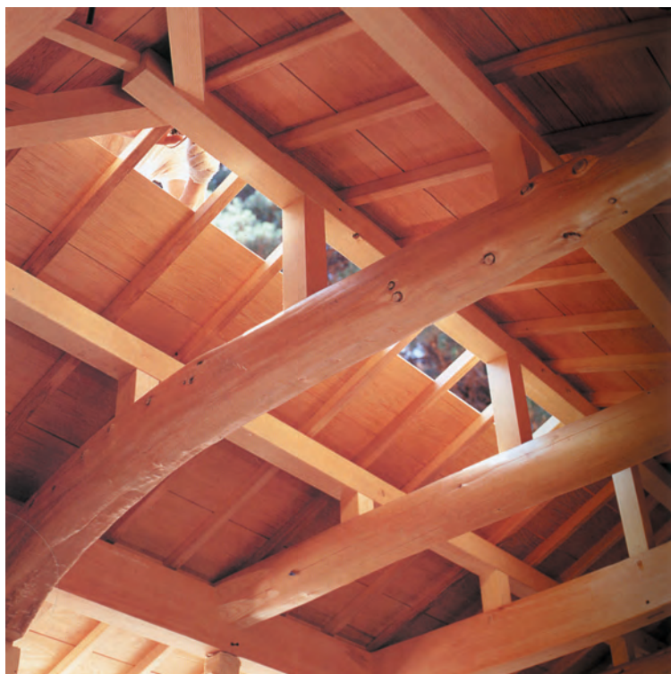
Guesthouse roof framing, a mix of cedars, with Western red cedar boarding not quite complete.
