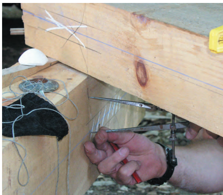
Fig. 7. Using dividers to transfer the brace half-width to the face of the post. End lines have already been established by string.
