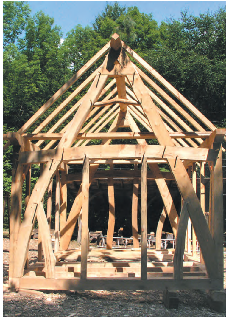
Fig. 19. Cruck frame built at the Heartwood School in Washington, Massachusetts, in a two-week workshop this summer, during which photos for this article were taken. All pieces in the 12x14-ft. frame were scribed except the rafters, which were square-ruled. Floor members were scribed using tumbling (see previous article in this series), wall and bent members, including cruck blades, were plumb-bob scribed, while the round-to-square connections in the upper part of the cruck were bubble scribed (the subject of the next article). Frame was a mix of hardwoods (mostly cherry) and softwoods; booked-matched cruck blades furthest from camera are Eastern white pine; blades nearest camera are spruce and aspen. Jack Sobon, who taught the workshop along with Dave Carlon, Josh Jackson and the author, designed the frame.
