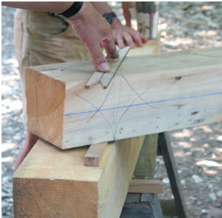
Fig. 16. Connecting the points representing the post-face line. Straight-edge happens to be a French-style homemade mortise and tenon gauge. In use, centerline marked by v-cuts registers on joinery centerlines.
