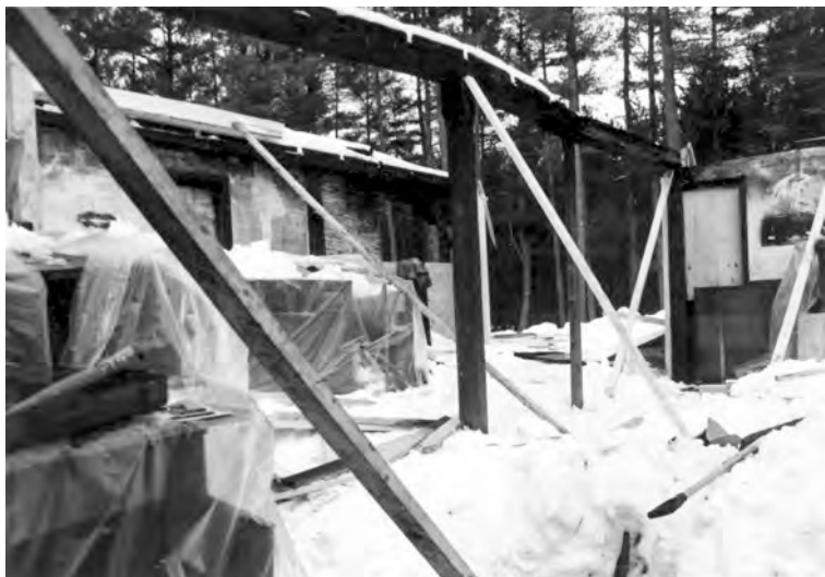
Tie beams over octagonal posts appear to have been set flush with the bottoms of the long plates, the latter burned away in this view.
