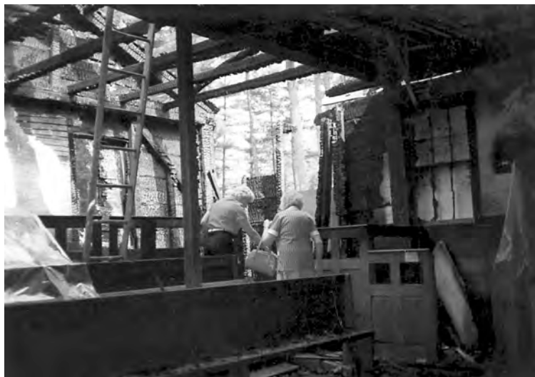
Two citizens inspect the remains of the meetinghouse. Intact end wall, ceiling joists and one tie beam visible. Box and bench pews survived.
