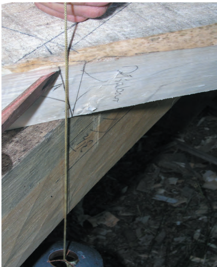
Fig. 13. Pencil indicating post-face line on brace is offset the distance from post face to string at housing location below, as measured along plane of lower face of brace. Mortise is already laid out.
