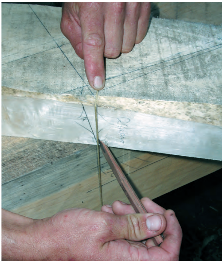
Fig. 14. Plumb bob string has been moved up brace arris from its position in Fig. 13 until lines don't cross. All lines shown in Figs. 13 and 14 have been laid out previously.
