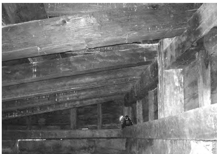
At upper end, joists rest on ledger, a kind of second sill on short posts.
