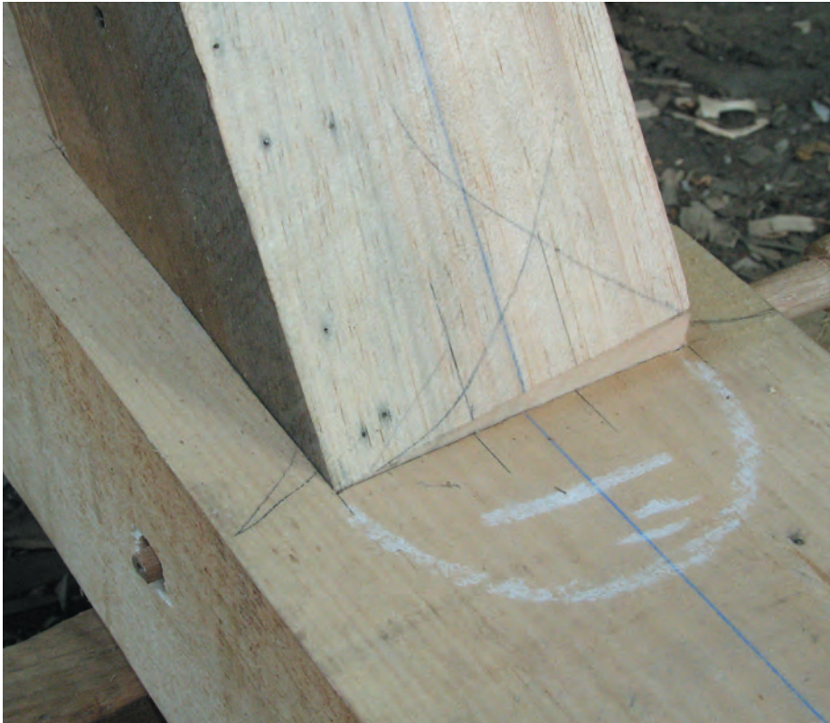
Fig. 1. Centered housed brace in irregular timber neatly achieved with scribe layout. Projection of brace nose above surface of meeting timber is called by its French name, “désabout.” Diminished housing is 1 in. deep at the bearing end, tapers to zero at the surface.
