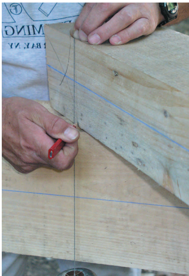
Fig. 9. Marking brace for bearing end of tenon. Pencil must be perpendicular to face of post since bearing housing is plumb to surface.
