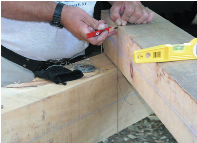
Fig. 15. Marking the upper side (or inside corner) of the brace.
