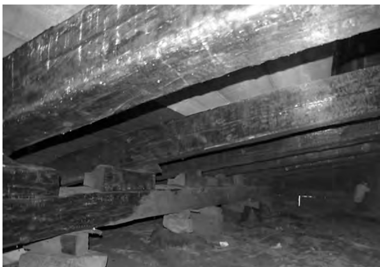
Heavy sloping joists rise from girders under central aisle.
