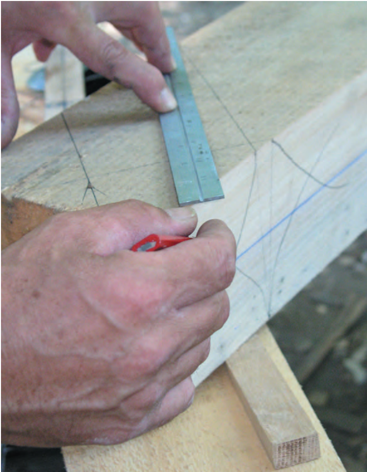
Fig. 18. Straightedge 1 in. wide laid along line of diminished shoulder after use as gauge to measure back 1 in. along bearing shoulder line from the post-face line, then pivoting to connect this new point with top point. This is the cut line for the tenon shoulder. During assembly of centered (blind-housed) brace, you can tell brace is fully seated when penciled post-face line meets post face.
