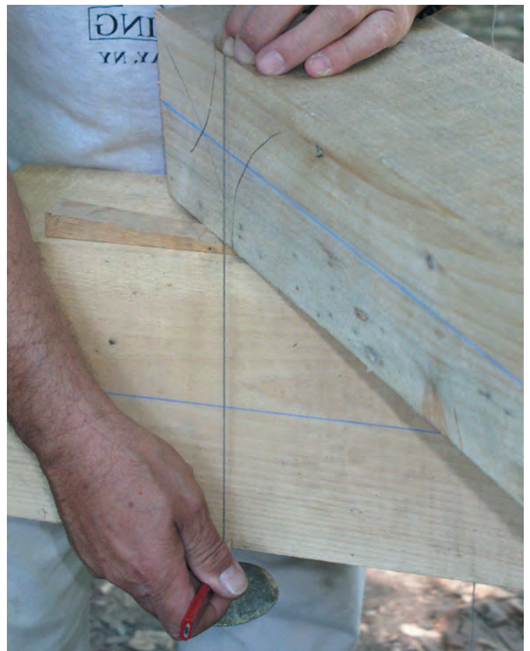
Fig. 5. Marking the post for the housing for bearing end of brace. Pencil is held perpendicular since bearing will be square to the surface. Housing mark is temporary; brace may have to be clipped farther up to make sure bearing face begins before brace enters post, and housing shifted as well.
