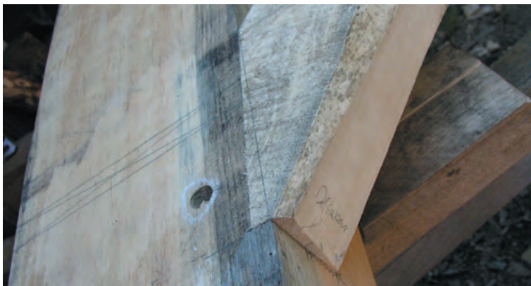
Fig. 12. Flush brace joint with désabout and diminished housing.
