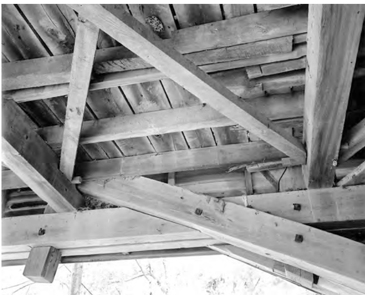
Fig. 3. Bottom chord is notched to let arch pass. Huffman Mills Bridge, Perry-Spencer counties, Indiana (W. T. Washer, 1864). Bottom chords accumulate dust and debris; this one needs cleaning.
