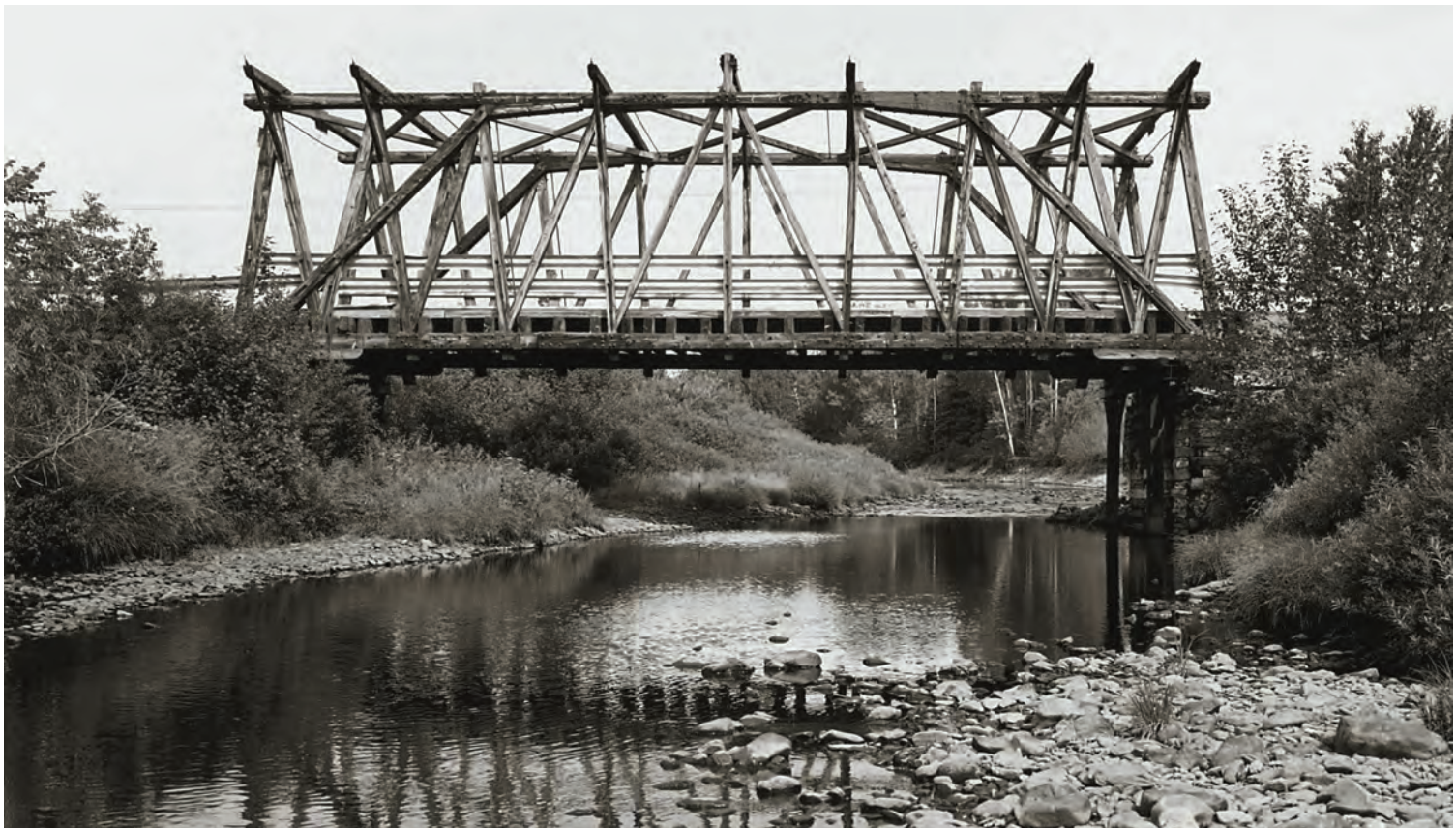
Fig. 11. New Brunswick struted Burr truss. McElwaine Bridge, at Temperance Vale (1955).
