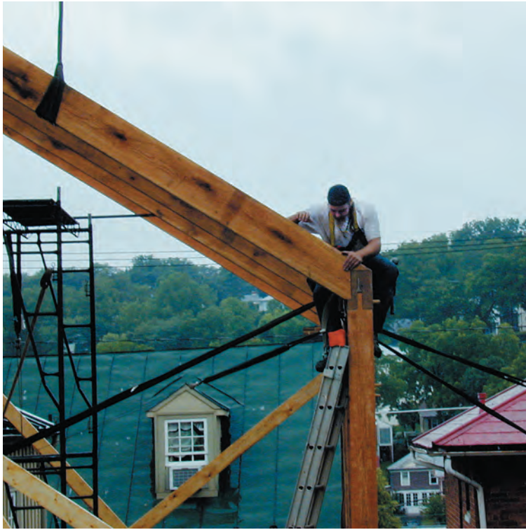
Fig. 3. Fitting the white oak rafters. Support is at ledge in plate and combines with support at underslung ridge to eliminate rafter thrust.
