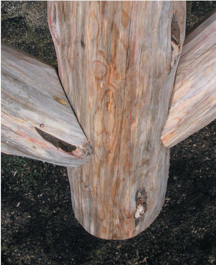
Fig. 12. Kingpost with two mitered struts, an instance when expected loading indicates unequal bearing shoulders and thus asymmetry in the miter.
