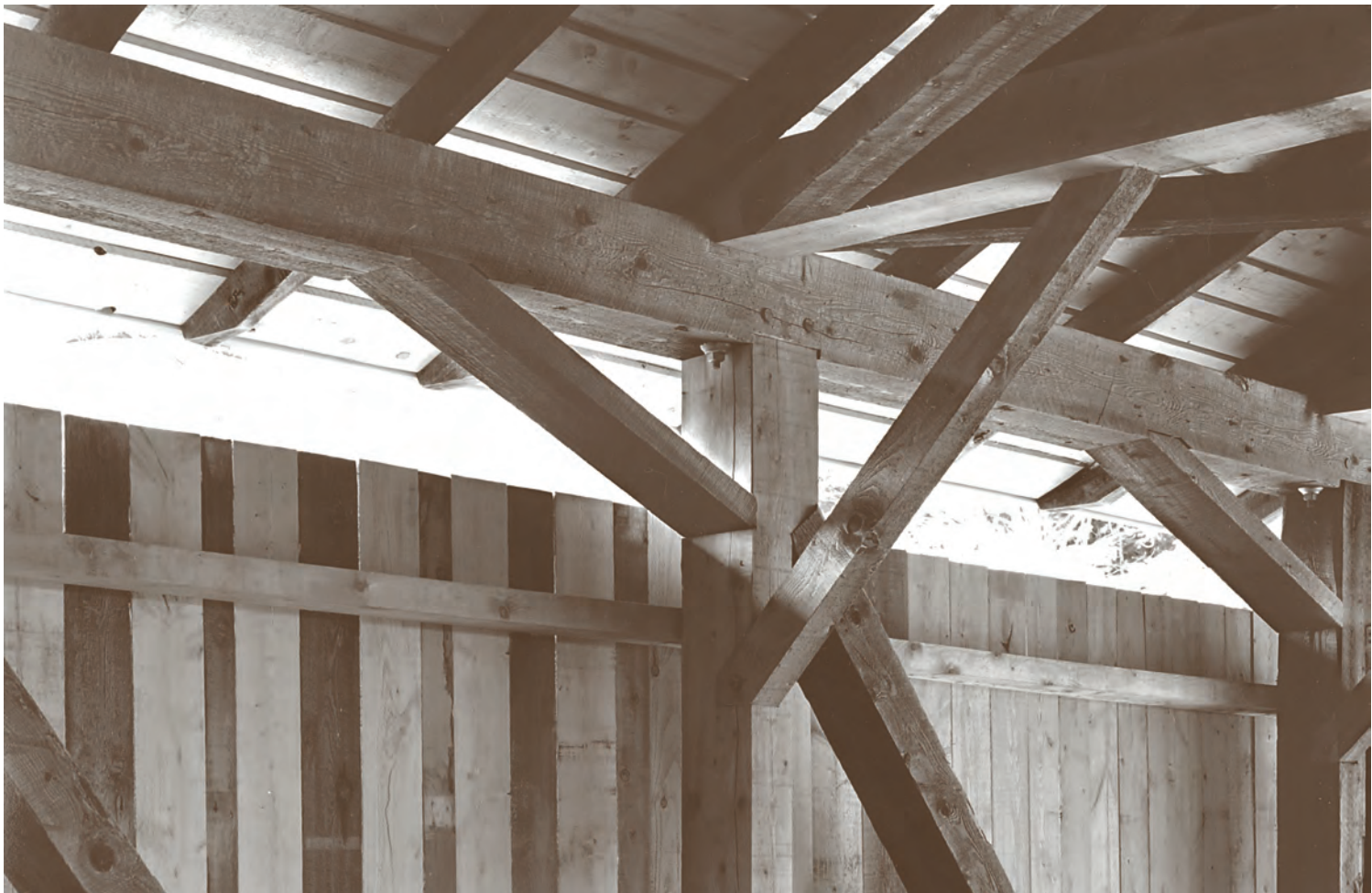
Fig. 6. Post-top chord joint, with check brace. Canyon Bridge, Jeffersonville, Vt. (builder and date unknown). Tie beam offset from its usual position over the post requires sway brace to be joined asymmetrically.
