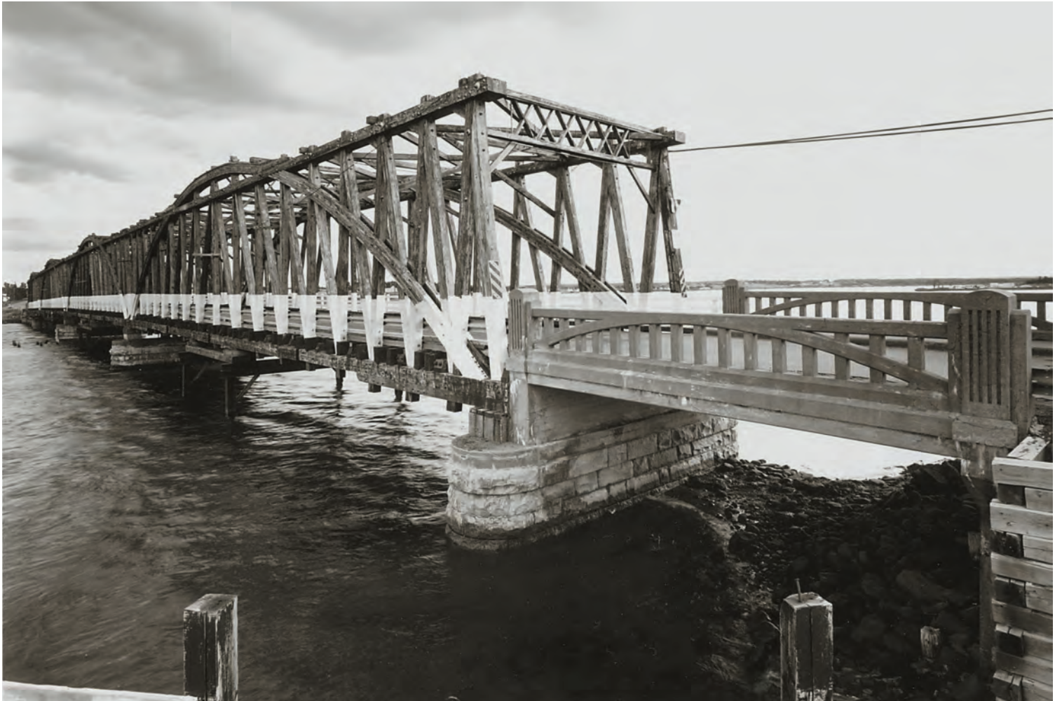
Fig. 10. New Brunswick arched Burr truss, at Cocagne (1941). Concrete approach railing mimicking the arch is an unusually fine touch and found on other bridges of this design from the Public Works Office.
