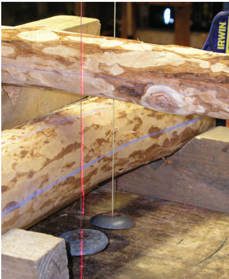
Fig. 13. A laser level can project a beam of light to aid in marking a projected plane on intersecting timbers.
