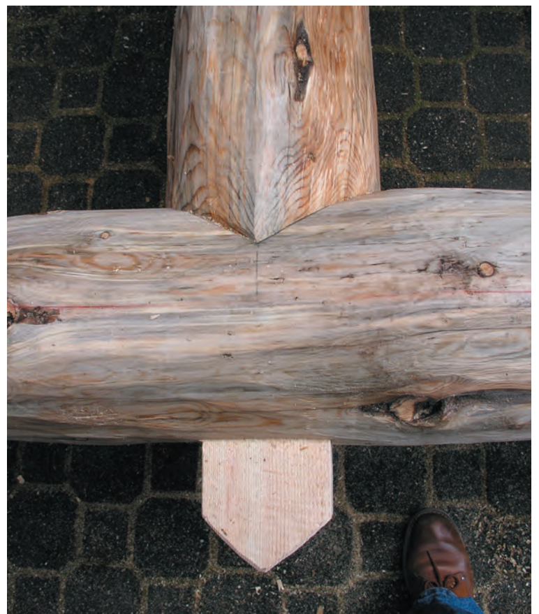
Figs. 7-8. Round-to-round mitered joint offers excellent bearing and neat appearance. Diameter of tenoned member will equal chord length of mortised member at joint. Example below has been artfully reshaped.
