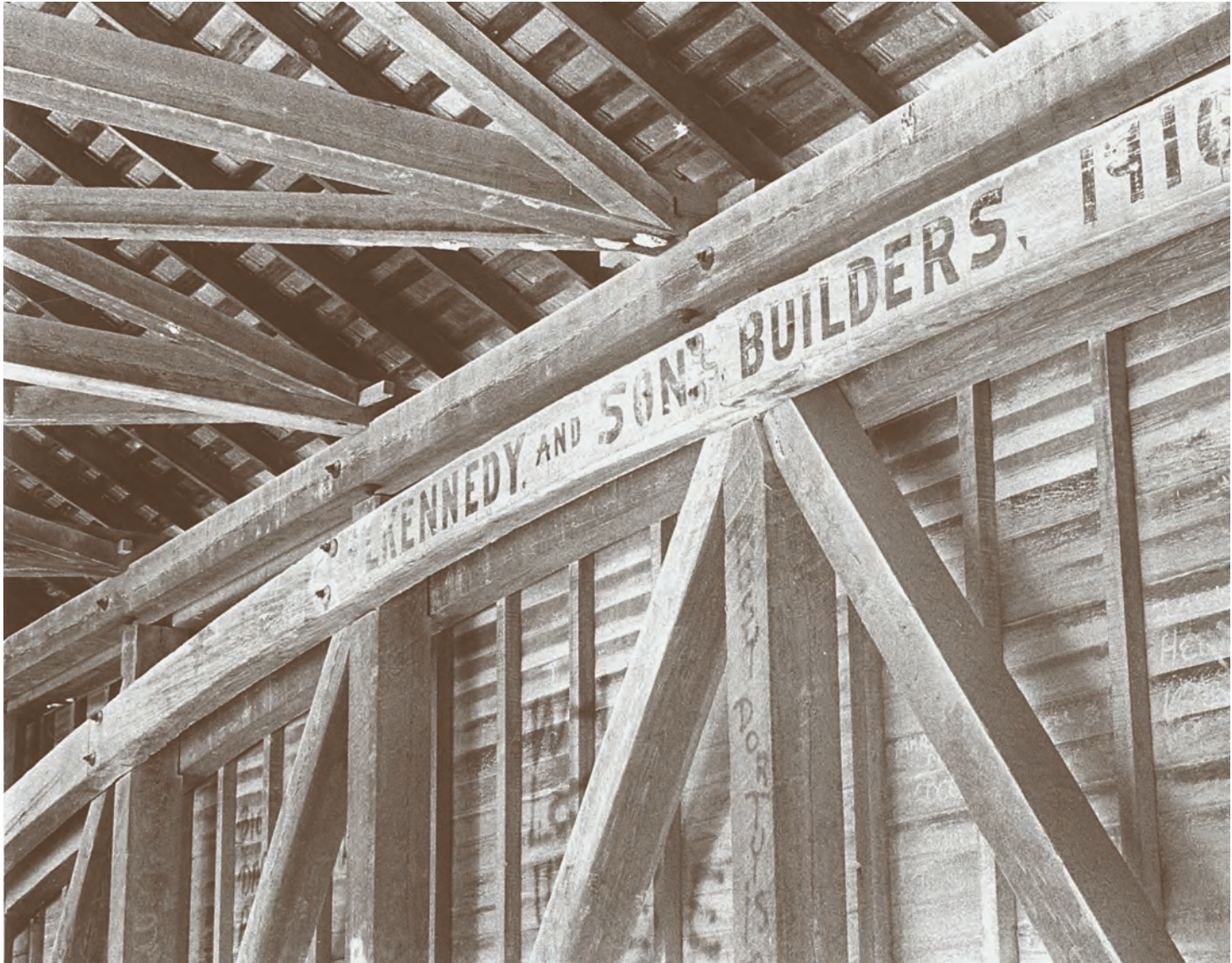
Fig. 7. Kennedy family bridge details from Indiana. Norris Ford Bridge, Rush County (1916). Note double top chord, tie beams slightly offset from panel points because of relish on post tops, arches slightly notched into posts. Many Indiana bridges display the builder's name, but more often on the portal.
