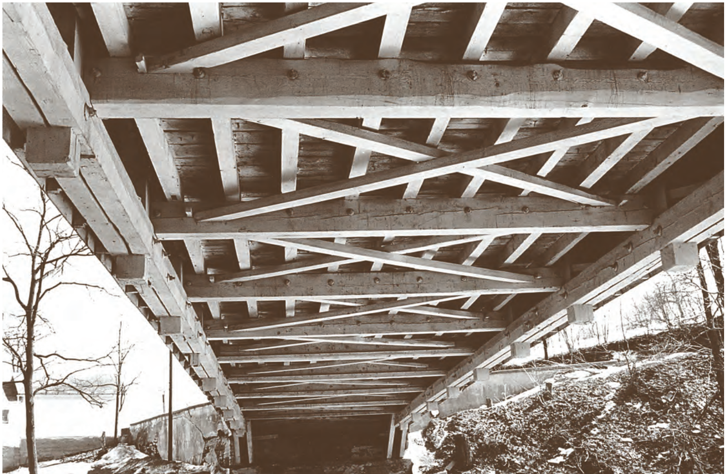
Fig. 5. Underneath Rex's Bridge, Lehigh County, Pa. (builder unknown, 1858). Floor beams are on same side of posts as main braces because check braces are on the other side; bolts in solid beams are likewise unusual. It is difficult to find one Burr truss bridge typical in all details.
