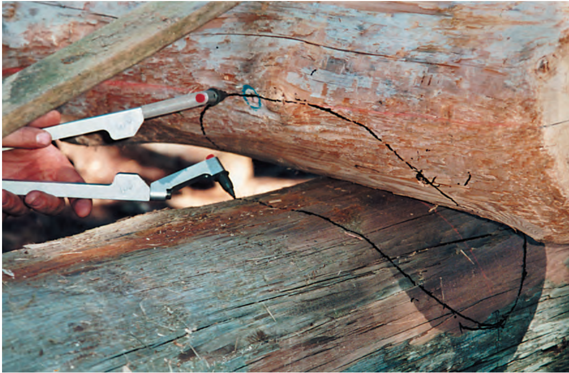
Fig. 1. Log-builder's scribe technique used here at a crossing of two round timbers is equally applicable to lengthwise joints and combinations of square and round timber. Cavity is severely undercut in upper member to clear all possible projections of lower member at the joint and produce a seamless appearance.
