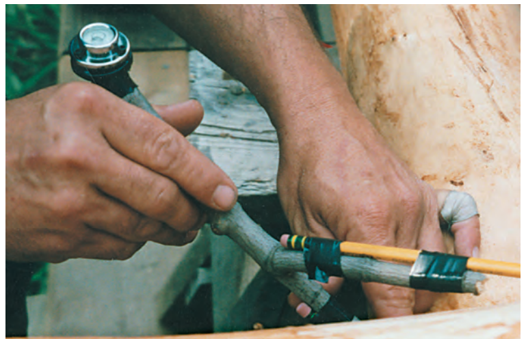
Fig. 5. Homemade scriber can be improvised with forked stick, pencils and bubble level.
