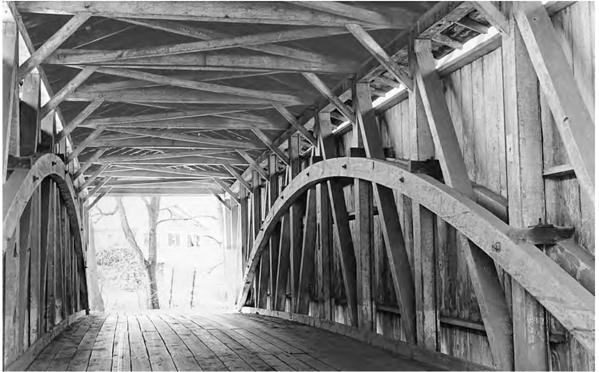
Fig. 2. The typical Burr truss. Kauffman's Distillery Bridge, Lancaster County, Pa. (built by Elias McMellen in 1874). Blocks on top of arches, with steel rods to the bottom chord, are later additions.
