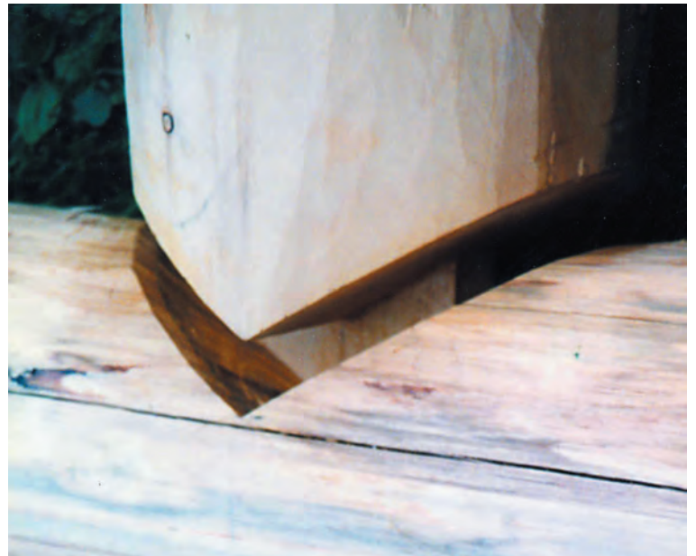
Figs. 7-8. Round-to-round mitered joint offers excellent bearing and neat appearance. Diameter of tenoned member will equal chord length of mortised member at joint. Example below has been artfully reshaped.
