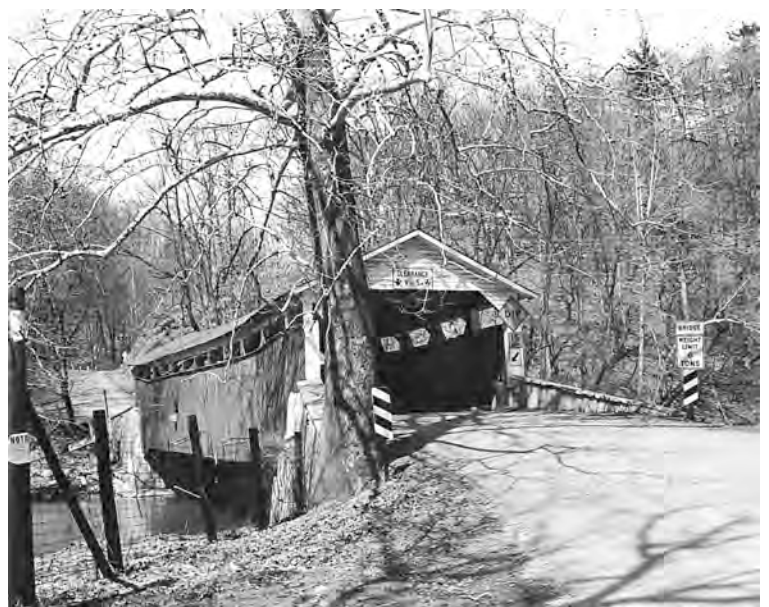
Fig. 4. A problem with the arch ends of this bridge is affecting the bottom chord and the entire truss. Schlicher's Bridge, Lehigh County, Pa. (builder unknown, 1882).
