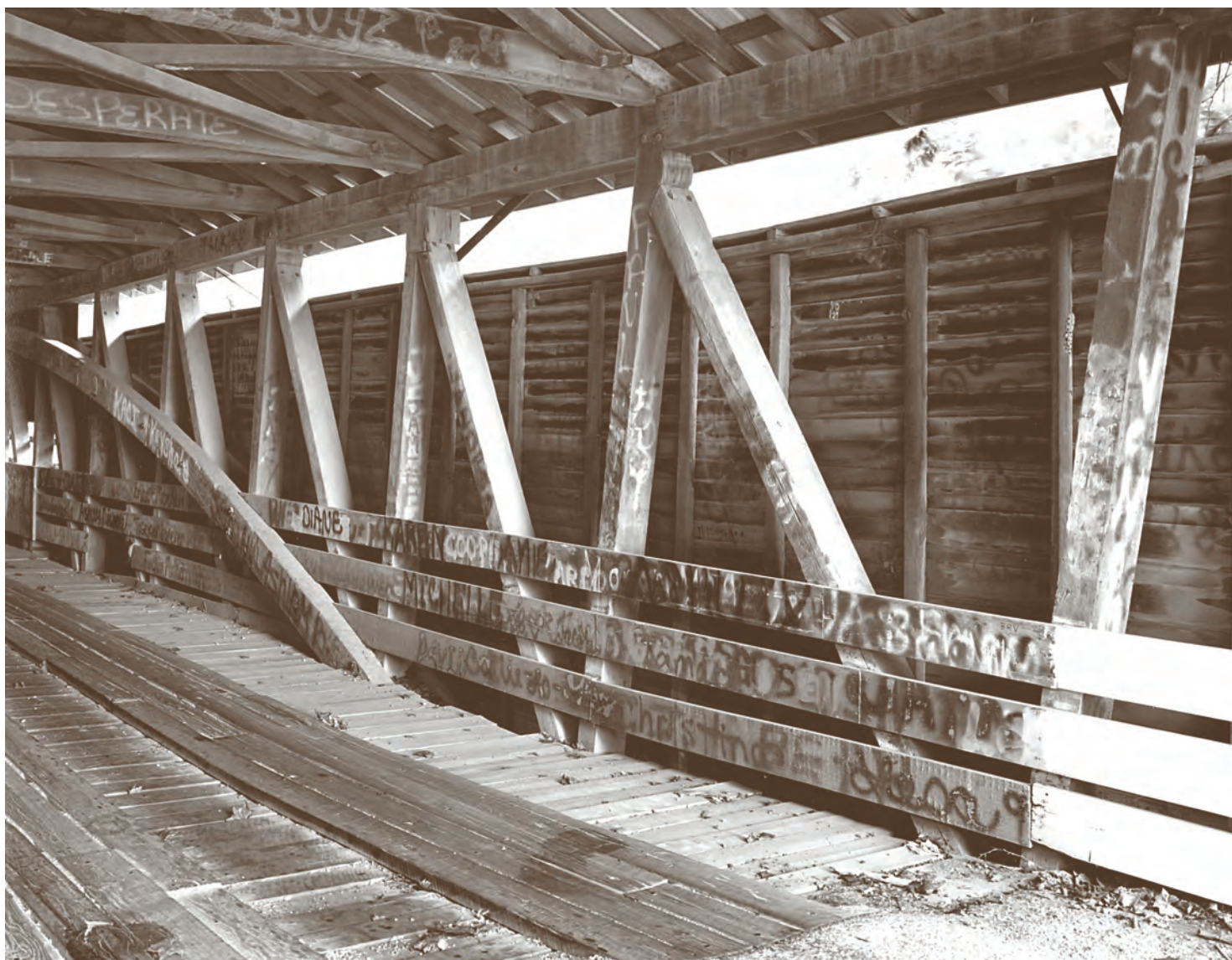
Fig. 8. Flared posts. Huffman Mills Bridge, Perry-Spencer counties, Indiana (W. T. Washer, 1864). Note skewed joints at tops of posts and curious surface shape between brace joint and chord joint. Graffiti, common enough in covered bridges, have flourished here.
