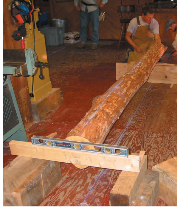
Fig. 3. Strategy for holding log level. With appropriate depth, stick can provide correct offset for scribing.
