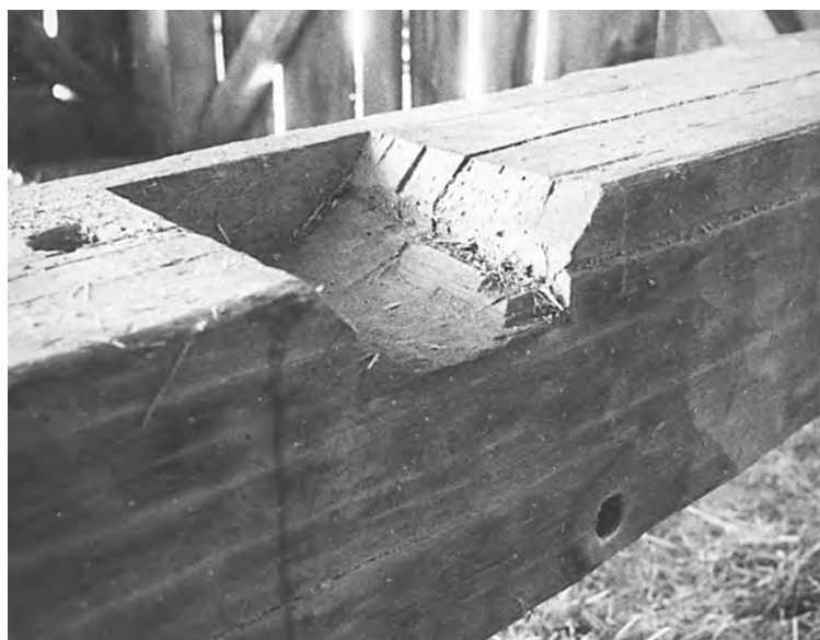
Figs. 8, 9. At top, the end of a "beef roll" salvaged from a collapsed barn. The roughly shaped 6-in.-dia. sugar maple log is reduced to 4 in. at the end and has two 2-in.-dia. holes bored through at right angles to each other, one at 5½ in. from the end, the other at 13 in. Fig. 9 above shows curved bearing notch in a tie beam from an 18th-century English barn in Adams, Massachusetts, that held one end of a beef roll just inside the south doorway.
