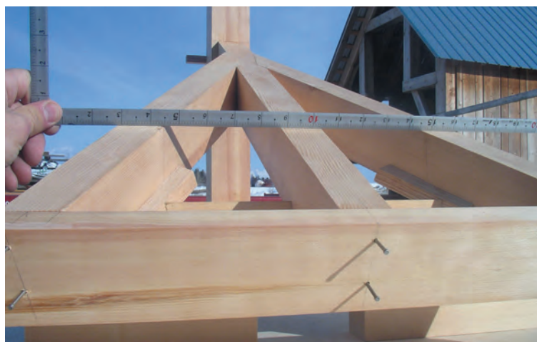
Fig. 3. Top surfaces of common and askew rafters form roof plane.
