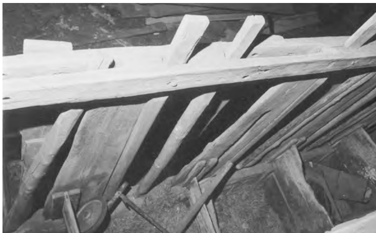
Fig. 6. Rare original cow stanchions in 32x42 Savoy, Massachusetts, barn, destroyed 1997 in a local fire department exercise. Two upright poles, one sliding, one fixed, are mortised into a 32-ft. hewn 4x5 at the top and a hewn 7x14 (on edge) at the bottom.
