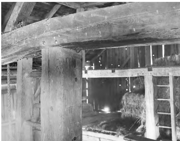
Fig. 7. Ladders on both sides of threshing floor in the extant 30x40 Savoy barn looking toward loft over the cows. Ladders could also be made by cantilevering the shaved rungs out from each side of a post.
