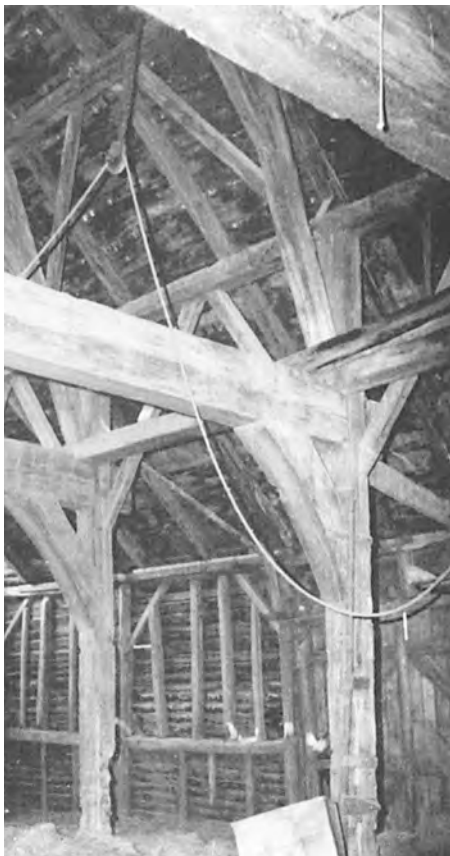
Van Bergen-Vedder barn, traditionally dated to 1680s, possibly post-1700, formerly at Leeds, Greene County, N.Y. Canted roof strutting is 19th century.
