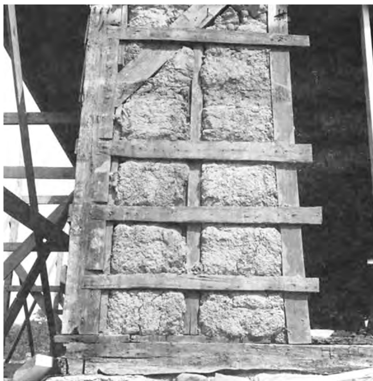
Photos and drawings John R. Stevens Framing of the Minne Schenck House, ca. 1730. Shingle lath passes over studs and brace but is let in to corner post.
