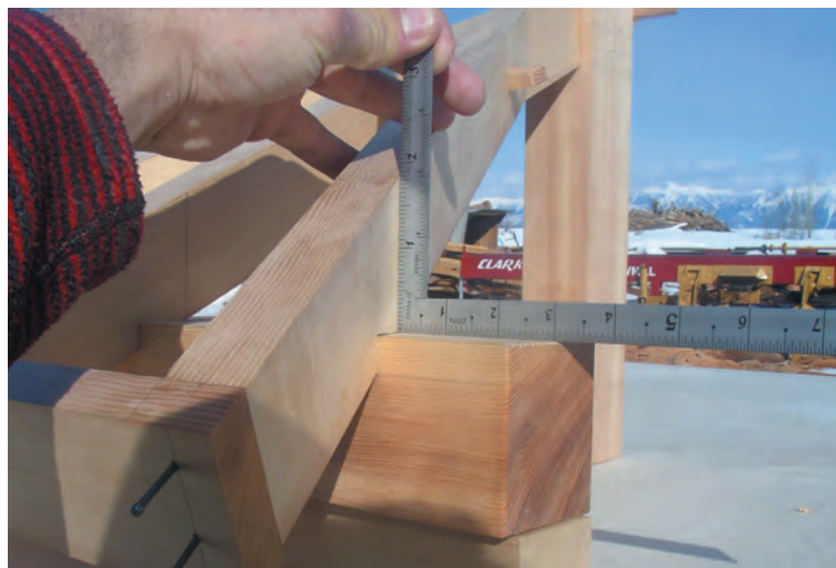
Fig. 2. Askew rafters are reshaped top and bottom; sides are held plumb.
