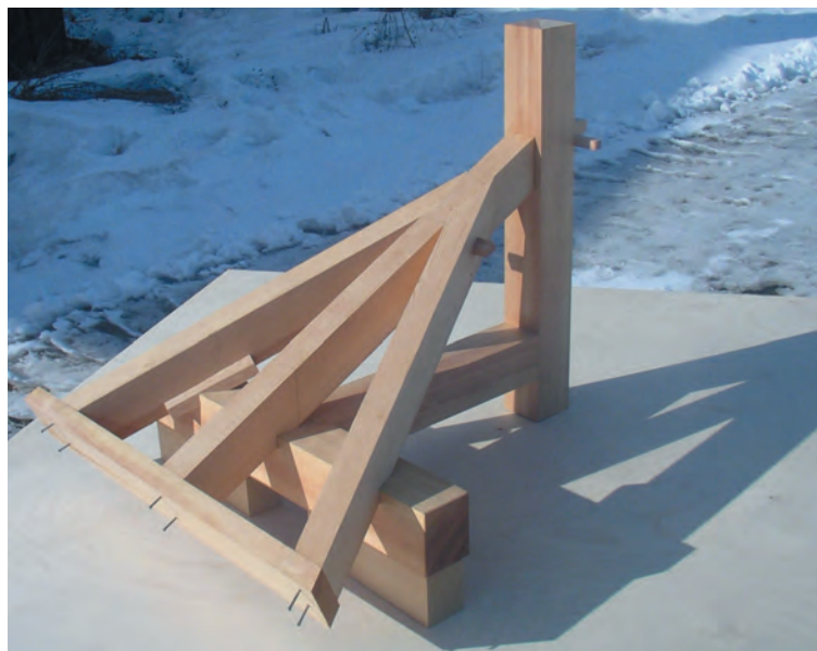
Fig. 1. The model demonstrates various joints as well as geometry.
