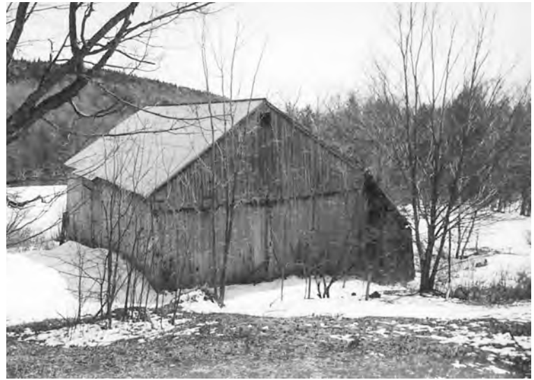
Fig. 4. Extant English barn, 30x40 ft., Savoy, Massachusetts, built before 1840. Use of square-rule layout dates it after 1812 in this area.
