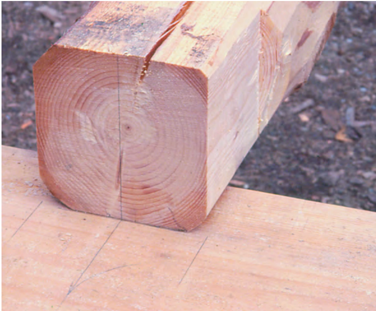
Fig. 12. Joist end reduced in width and projected on sill preparatory to cutting pocket. This work is all done to centerlines.
