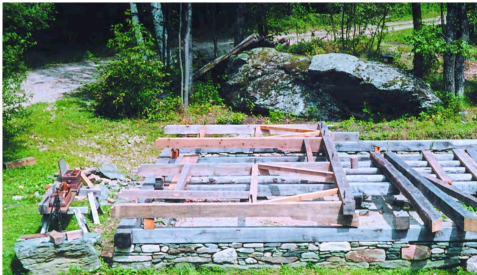
Fig. 18. Stone foundation with square and level floor frame makes an excellent platform on which to scribe the rest of the frame.
