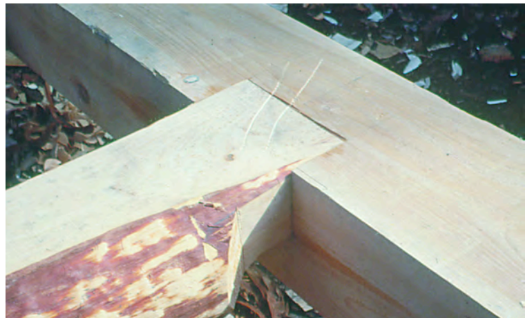
Fig. 16. True marriage marks indicating joint number 2.
