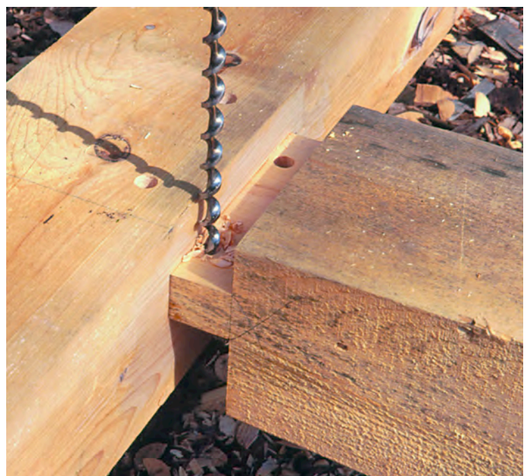
Fig. 8. Drawboring the mortise and tenon joint. After using the drill-bit to prick through the pinholes in the mortise with the joint closed, the tenon is withdrawn far enough to offset the marks toward the shoulder and bore the holes.
