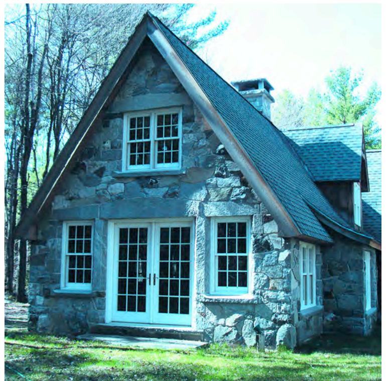
Fig. 2. Heavy rock-pitched faces and substantial lintels in stone veneer on a timber-framed house in western Massachusetts.
