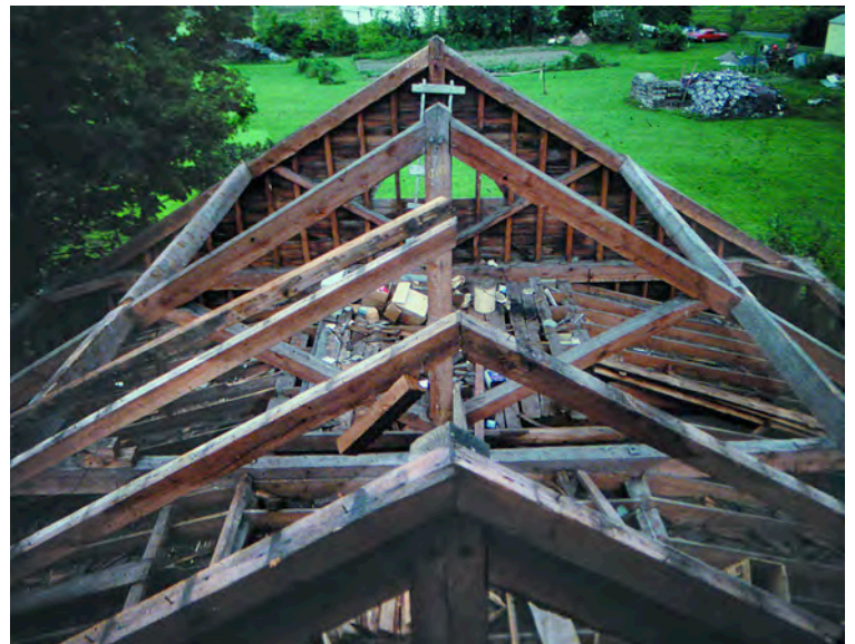
Dismantling the kingpost truss roof frame, as seen from the steeple. Steeple truss was queenposted.
