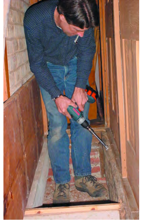
Above, Sheldon house, Deerfield. Main house (front) redated from 1735 to 1755 with confirmation of dendro. Above right, Bill Flynt coring chimney girt in the 1735 Col. Ashley house, Ashley Falls, Massachusetts. In the latter house, dendro confirmed documentary date.
