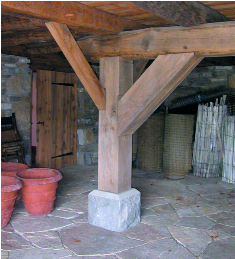
Fig. 4. Impermeable stone plinths raise posts out of ground and block rising damp. Paving with stone keeps storage areas drier.
