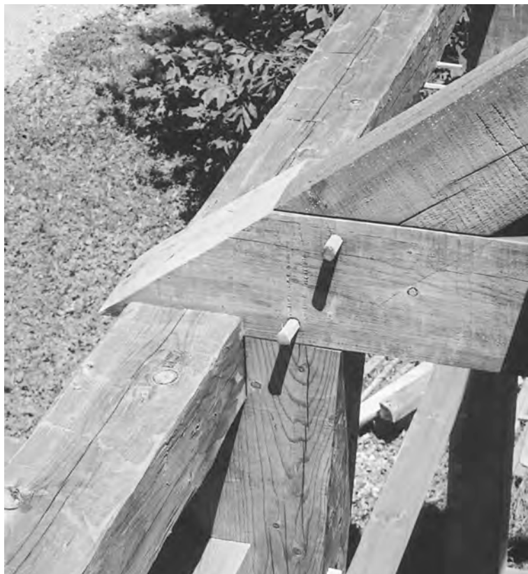
Fig. 1. English tying joint in author's barn. Post jowl, center, is joined to tie beam via teazel tenon; post is tenoned separately to continuous plate, left, which also passes under tie while capturing it in a shallow dovetail housing, unseen. Rafters are tenoned into tie for base-tied truss.
