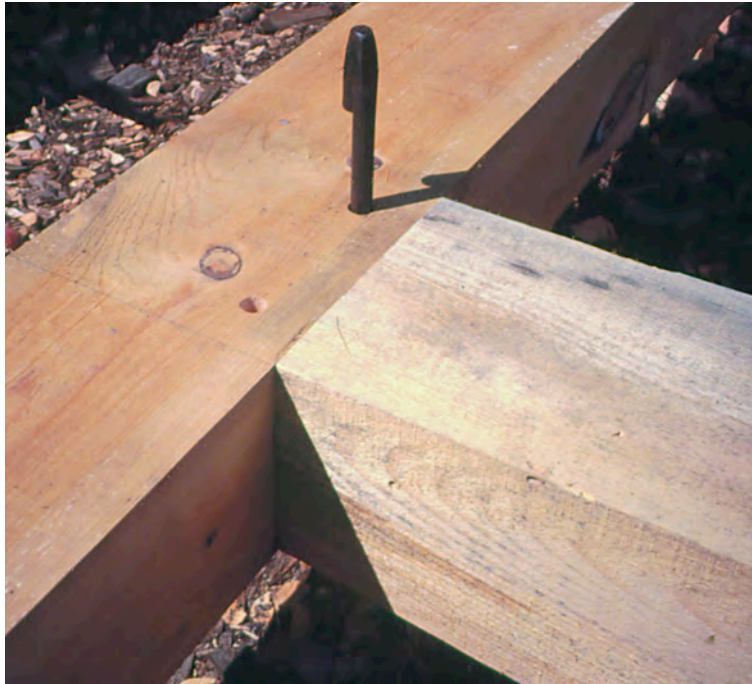
Fig. 9. Sill joint assembled and held temporarily with a tapered drift or hookpin, which can be levered out. Pins that can be conveniently turned while being withdrawn are easier to use.
