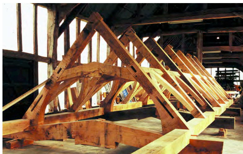
Above, upper cruck roof frame fully assembled in the workshop. At top, frame in place over Pilton barn, with one side lathed and tiled over.
