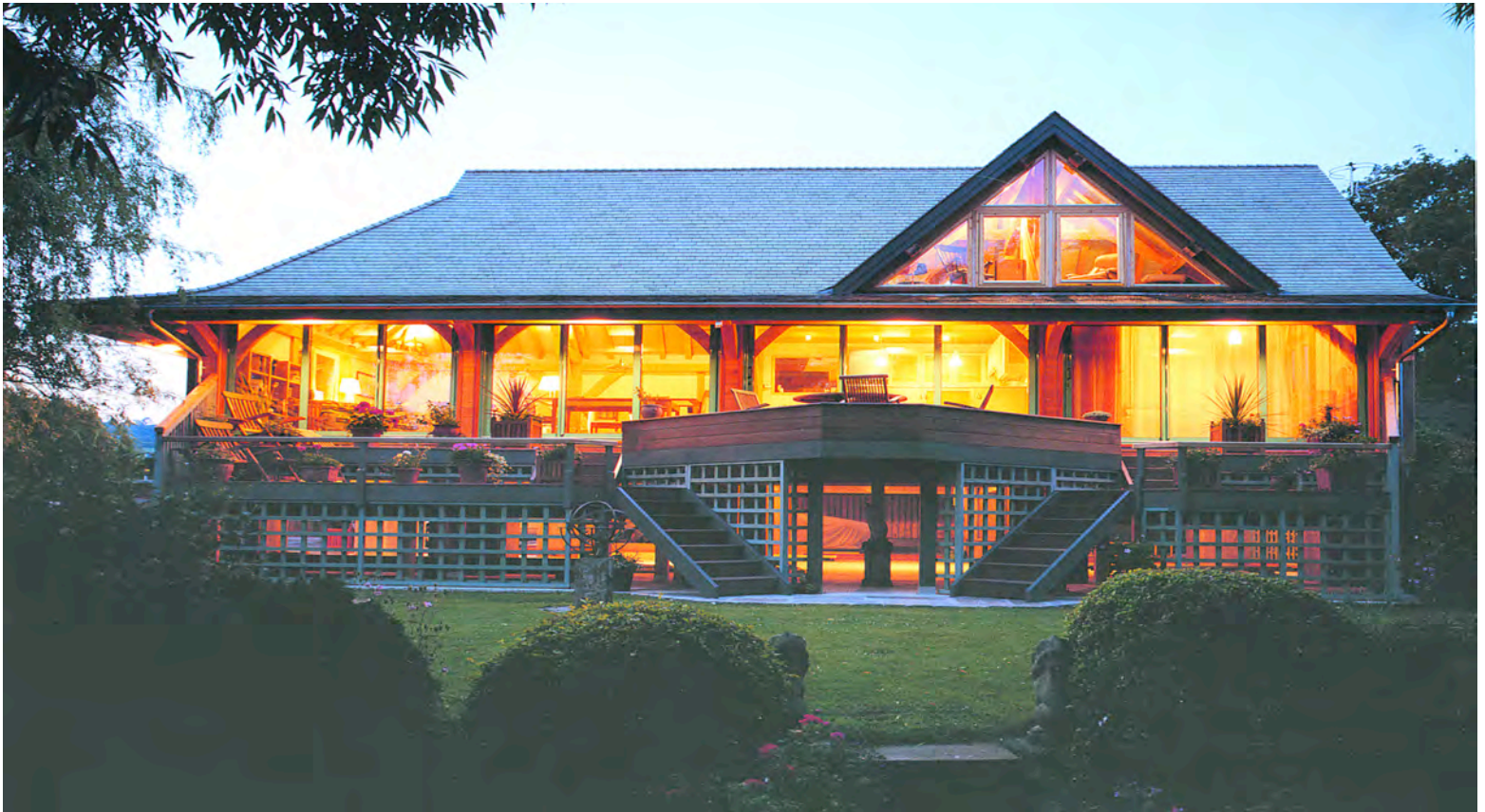
Fig. 4. Raised house for site prone to occasional flooding, designed by Wilfred Burton, a bold combination of traditional framing with modern fenestration and an open plan.
