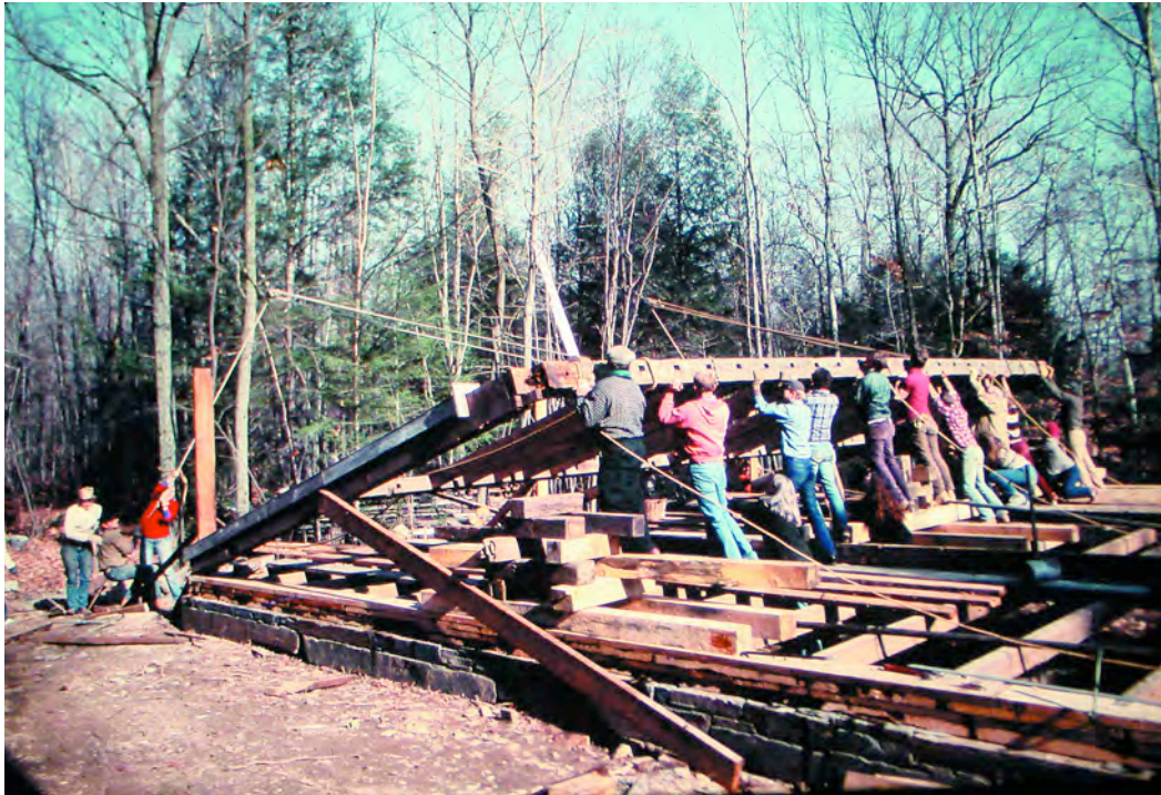
Raising the first wall of the relocated church at Eastfield on Guy Fawkes Day, 1982.
