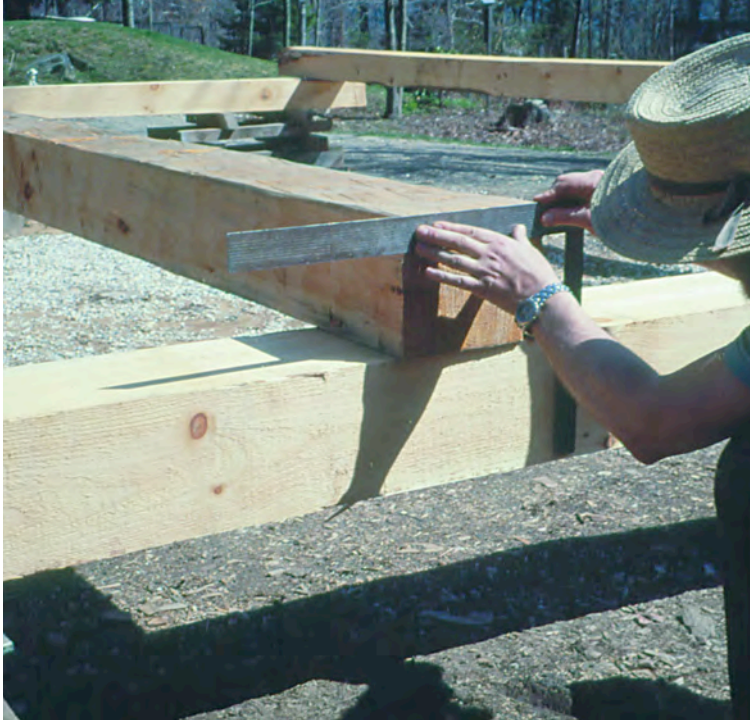
Fig. 3. Sighting across the top of the blade of a square to make it flush with the high spots on a hewn sill. A line is then drawn along the underside of the blade to describe the 2-in. joinery line.
