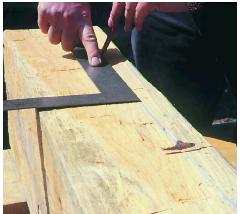
Fig. 7. Laying out a sill tenon. On lined timber, the square is set flush to the chalk line and a line scratched on both sides.
