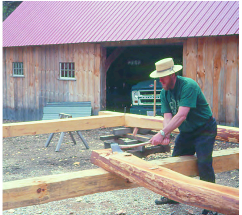
Fig. 10. Hewing the notches in the sleeper to allow it to come flush with the bottoms of the joists, which are 2 in. shallower than the intermediate sills. Notches also locate and stabilize the latter.
