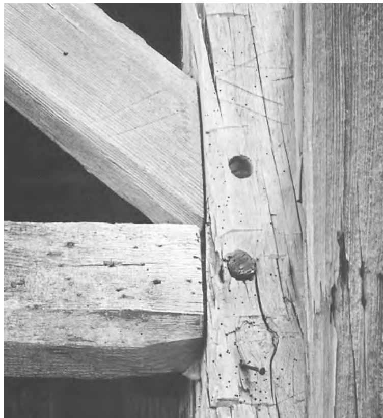
Fig. 2. Shared mortise in barn in Plainfield, Massachusetts. A scribe line seen crossing the V mark shows the brace mortise layout; the girt's underside has been reduced to fit the mortise, which has been precut to a standard length.
