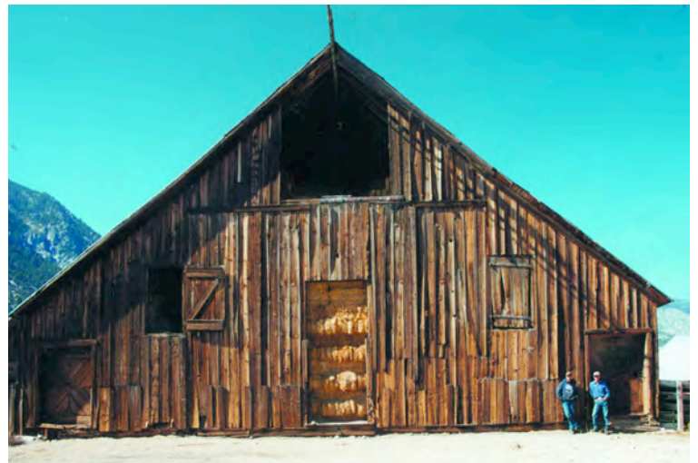
Scossa barn, Minden, Nevada, 1908, a good example of Carson Valley barns, in original condition and equipped with Jackson hayfork. Note unhappy grandsons. The softwood frame has three bays 18 ft. on center and measures 60 ft. wide by 54 ft. long. Central aisle appears full of hay.
