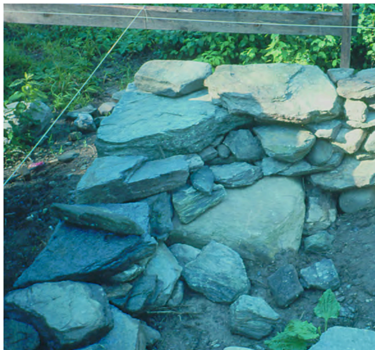
Fig. 17. The stonework is faced only on the outside. Note the large cornerstone, original batter board and stretched level lines.
