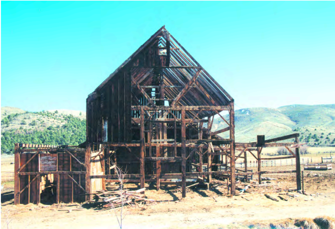
Palmer-Barber Bruns barn, Diamond Valley, California, about 1860. Apparently Dutch influences include tapered rafters and through tenons, though ethnicity of builders is unknown.
