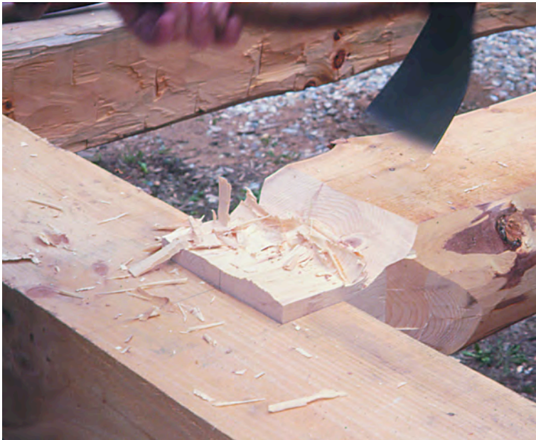
Fig. 13. Joist is inserted upside down and tenon shaped with axe and adze until flush with top of sill.
