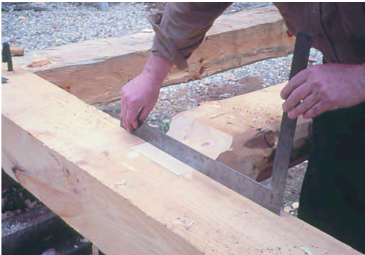
Fig. 14. Work is checked with a square for flush. Joist is then inverted.
