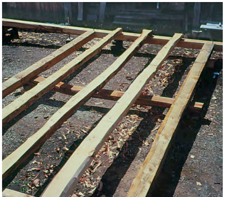
Fig. 11. The threshing-floor joists are positioned on blocking, ready to have their end tenons cut. Note sleeper beneath.
