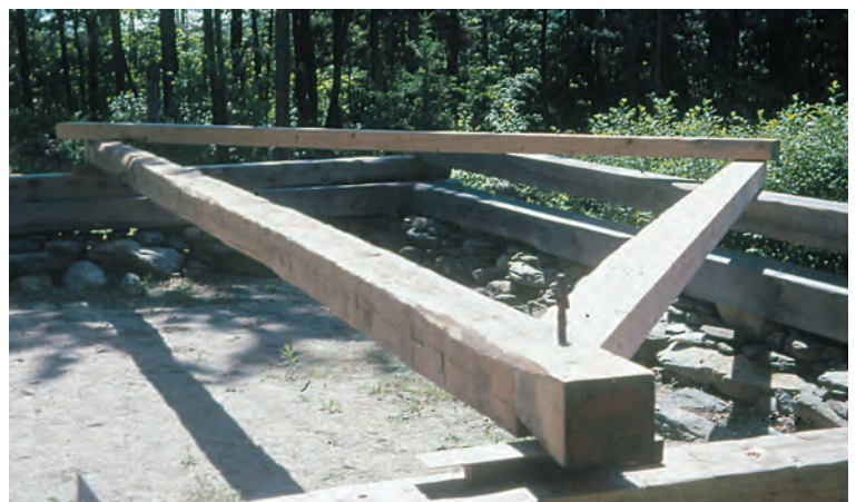
Fig. 8. Scribing rafter to tie beam. The roof triangle, face up, lies flat, supported by the next tie beam. One rafter has been scribed and fitted; the second is in process.
