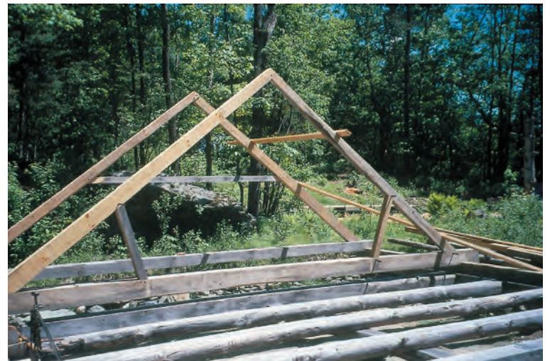
Fig. 11. In this view of a test assembly, end rafters are collared to support siding, intermediate rafters strutted to help bear roof load.
