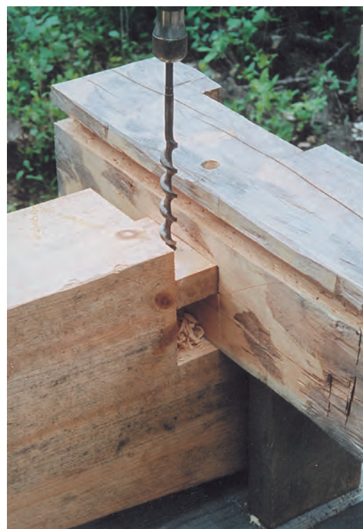
Figs. 21–23. Sequence for joining plate to post. Tenon shoulders are cut strong, then recut after scribing of waney mortise face. The joint brought home, pinhole center is pricked through previously drilled hole across mortise. Plate is then withdrawn sufficiently to recenter the pinhole mark closer to the tenon shoulder for the draw, and the hole is drilled through the tenon and (if the bit allows) the rest of the post.
