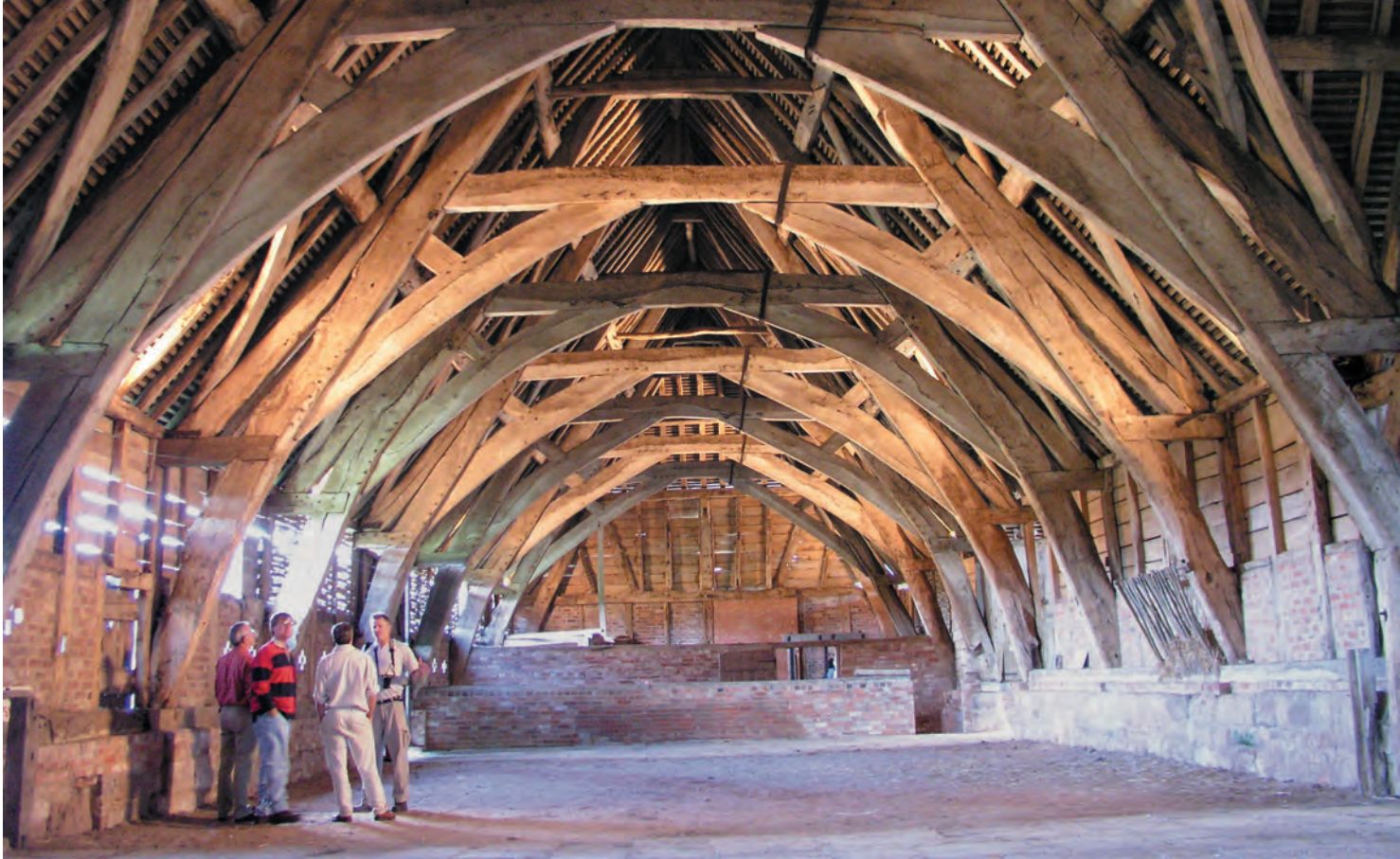
Late 13th-century tithe barn at Leigh Court, Worcestershire, reputed to be the largest full cruck frame in Britain, 150 ft. long, 33 ft. 6 in. wide, 34 ft. high.
