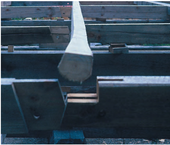
Figs. 12–14. Above, small ridgepole sitting over rafter peaks (peaks no longer over struck centerline); tenoned side of joint will be notched later at raising. At right, 13, purlins are already joined to the rafters. Below, 14, closeup of half lap joints and 8-in. purlin overhang.
