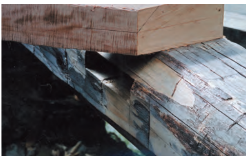
Figs. 15–17. Sequence of scribing brace shoulder to waney timber. Truing wane parallel to mortise side simplifies procedure.
