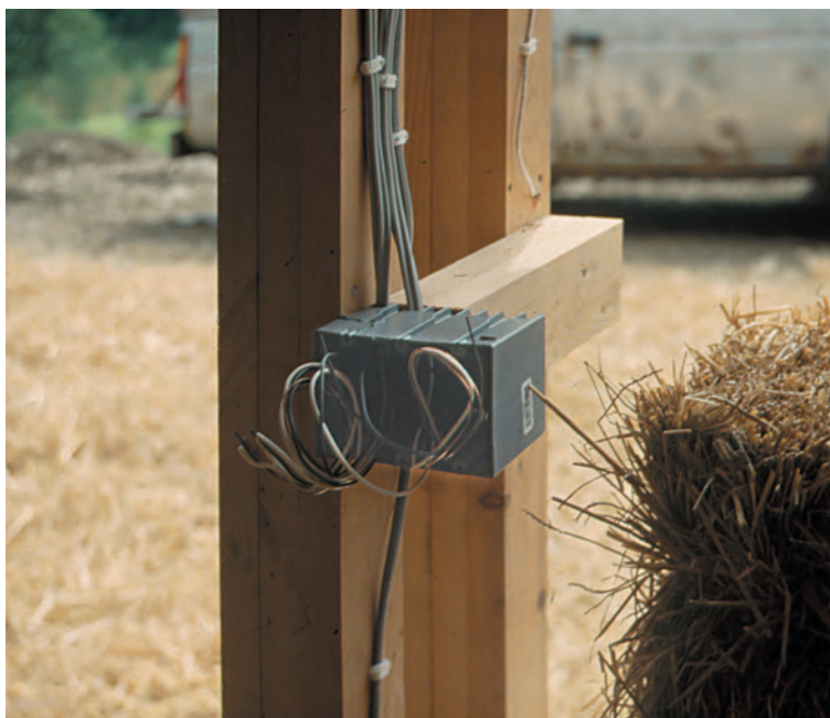
Figs. 5–6. Bales are notched at bottom for sturdy wiring chase. Below, switches are wired before bales are installed.
