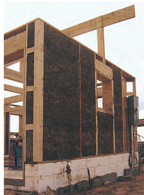
Fig. 4. A finished clay-straw wall, ladder (Larsen) truss visible at corner. Clay-straw is lifted high off ground on ICF stem wall.
