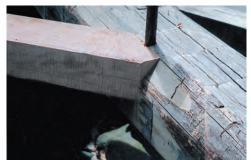
Figs. 15–17. Sequence of scribing brace shoulder to waney timber. Truing wane parallel to mortise side simplifies procedure.
