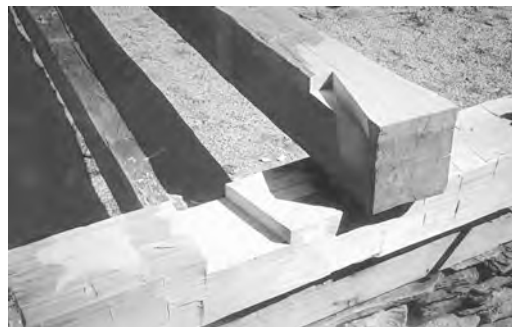
Figs. 5–6. Lapped half-dovetail joint at plate. Mating surfaces have been corrected.
