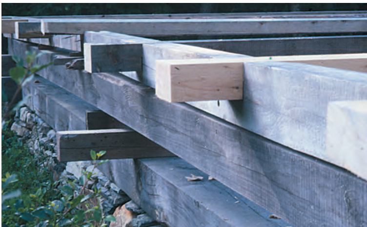
Figs. 12–14. Above, small ridgepole sitting over rafter peaks (peaks no longer over struck centerline); tenoned side of joint will be notched later at raising. At right, 13, purlins are already joined to the rafters. Below, 14, closeup of half lap joints and 8-in. purlin overhang.
