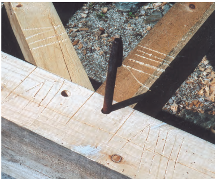
Fig. 25. Brace and girt mortises (or mortises for opposed braces) can be shared advantageously, easing and speeding the work. When numbering, Vs are inverted to suit action of race knife, which cuts most controllably if pulled from point of V.
