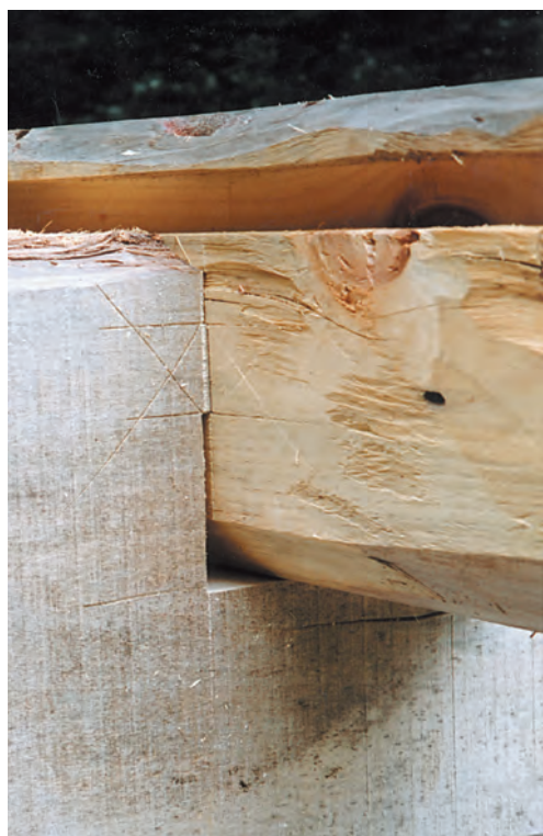
Figs. 21–23. Sequence for joining plate to post. Tenon shoulders are cut strong, then recut after scribing of waney mortise face. The joint brought home, pinhole center is pricked through previously drilled hole across mortise. Plate is then withdrawn sufficiently to recenter the pinhole mark closer to the tenon shoulder for the draw, and the hole is drilled through the tenon and (if the bit allows) the rest of the post.
