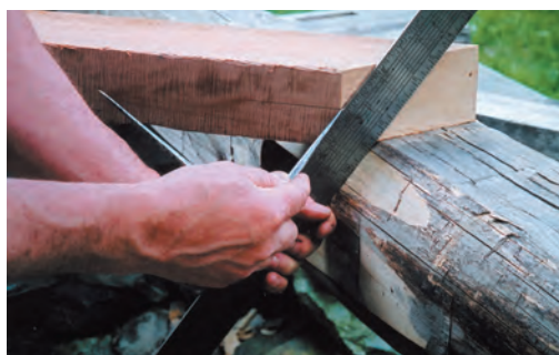
Figs. 15–17. Sequence of scribing brace shoulder to waney timber. Truing wane parallel to mortise side simplifies procedure.
