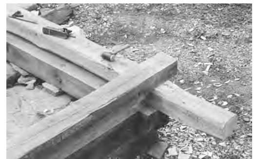
Fig. 7. Scribing end tie over plate.
