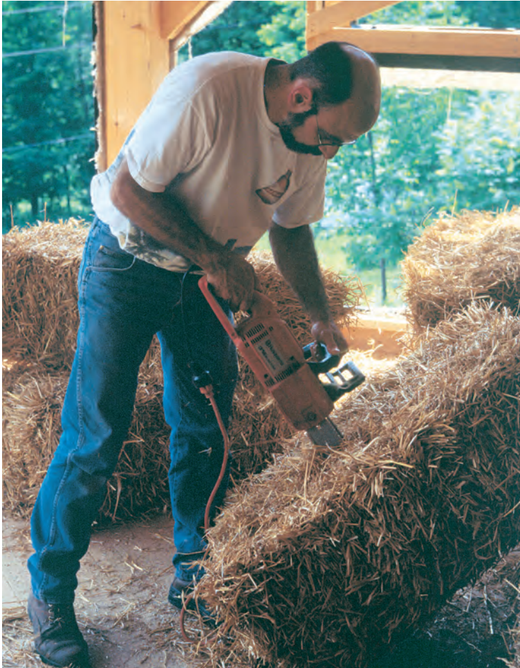
Fig. 9. Mike Basile chainsaws a bale to custom width.
