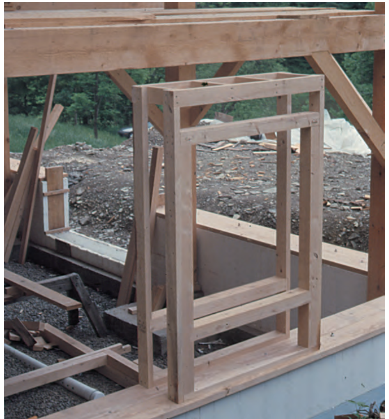
Fig. 3. Standing window buck on high foundation wall.
