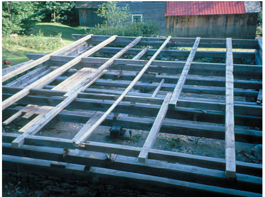
Figs. 12–14. Above, small ridgepole sitting over rafter peaks (peaks no longer over struck centerline); tenoned side of joint will be notched later at raising. At right, 13, purlins are already joined to the rafters. Below, 14, closeup of half lap joints and 8-in. purlin overhang.
