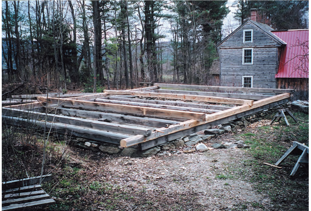
Fig. 4. Deck assembled, the eaves-level frame (plates and ties) superimposed for scribing. Plates lie outside long sills to account for siding groove. Interior ties are on edge, end ties flatwise. Sufficient trim is left to allow some adjustment at joints to avoid timber defects. Plates will ultimately be trimmed for an 8-in. overhang at the gable ends.
