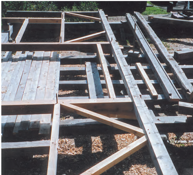
Fig. 24. Front long wall assembly completed, with braces, door headers and nailers scribed and fitted. Note detached inverted end tie at right with boarding groove showing on underside.
