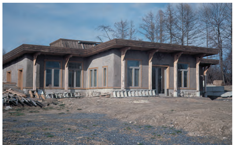
Figs. 11–12. Timber-framed house, Lansingville, N.Y. At left, baling almost complete, with window and door bucks ready for trim. At right, plastered and trimmed. Broad overhang is desirable to keep walls dry. Roof brackets are independent of frame.
