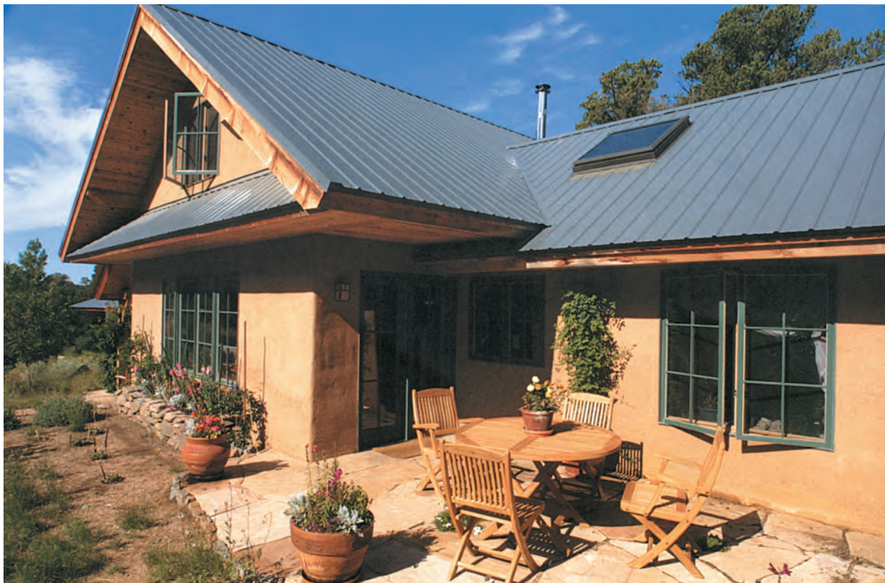
Fig. 5. In the Southwest, the authors often use clay-based plasters for exterior finish on their designs. La Barbara Canyon, New Mexico.
