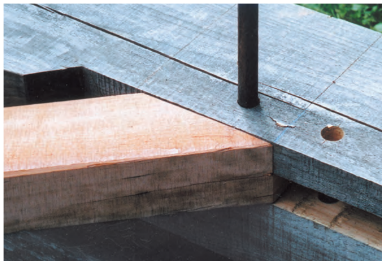
Fig. 19. Stop at base of jowl lies just above transverse brace mortise, lengthened here to accept loft floor beam.
