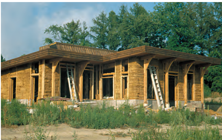
Figs. 11–12. Timber-framed house, Lansingville, N.Y. At left, baling almost complete, with window and door bucks ready for trim. At right, plastered and trimmed. Broad overhang is desirable to keep walls dry. Roof brackets are independent of frame.
