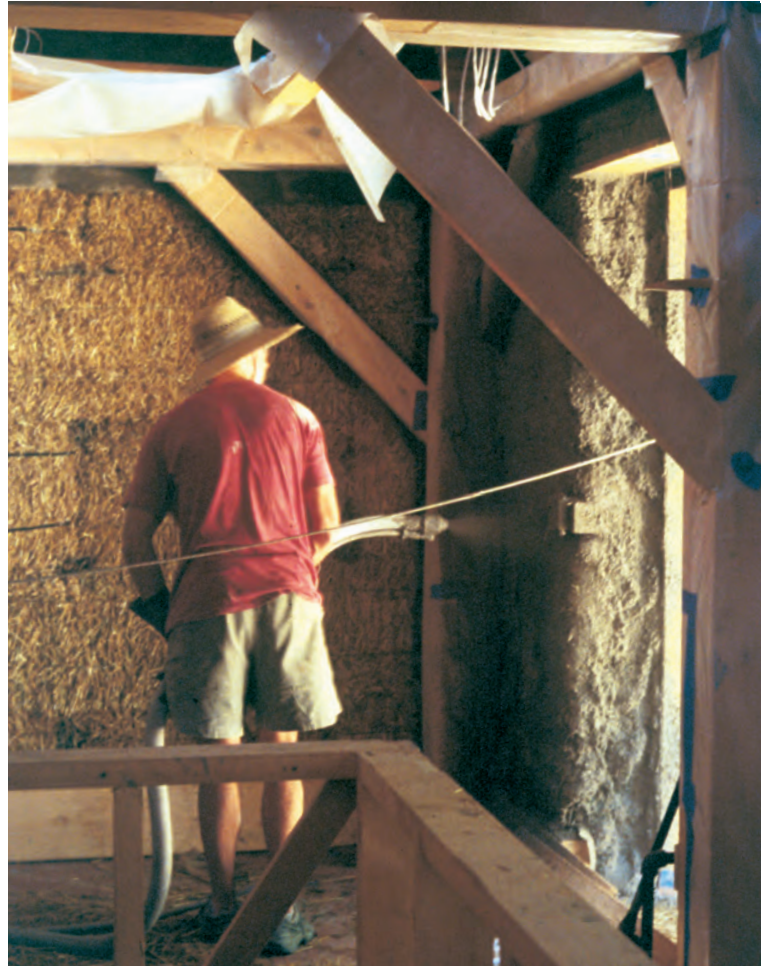
Fig. 10. A plaster pump is practical for large jobs.
