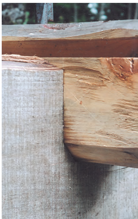
Figs. 21–23. Sequence for joining plate to post. Tenon shoulders are cut strong, then recut after scribing of waney mortise face. The joint brought home, pinhole center is pricked through previously drilled hole across mortise. Plate is then withdrawn sufficiently to recenter the pinhole mark closer to the tenon shoulder for the draw, and the hole is drilled through the tenon and (if the bit allows) the rest of the post.
