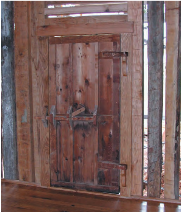
Fig. 4. Plank door swings on wooden pintle hinges.
