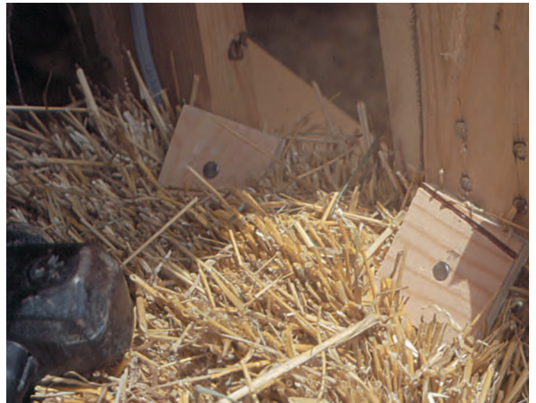
Figs. 7–8. Bale nails fasten straw to window framing. Below, bale spikes fasten bales to timbers.
