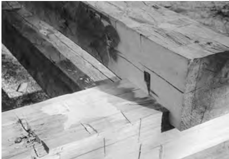
Figs. 5–6. Lapped half-dovetail joint at plate. Mating surfaces have been corrected.
