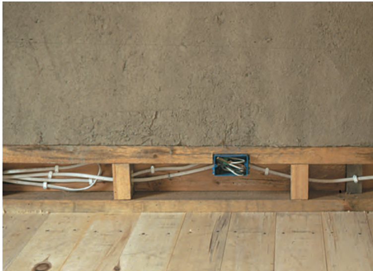
Figs. 5–6. Bales are notched at bottom for sturdy wiring chase. Below, switches are wired before bales are installed.
