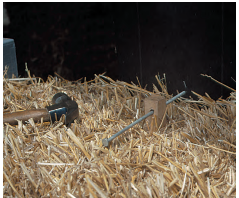
Figs. 7–8. Bale nails fasten straw to window framing. Below, bale spikes fasten bales to timbers.
