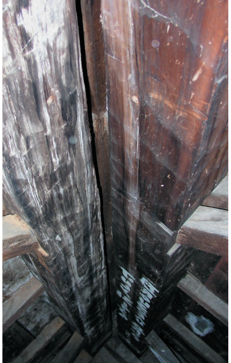
Fig. 21. Eight 12x12x28 posts in cater-corner pairs rise from the belfry roof to the top of the clock stage. Plan views in Figs. 5–6.
