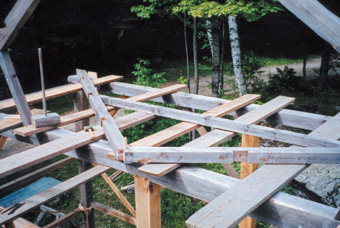
Fig. 10. Gable rafter pair with collar assembled over spaced planks on tie beams. Already erect, one intermediate rafter pair with raking struts was assembled piecemeal in position. Note notches for ridge and purlins. Detail below, closeup of stop nailed to tie to restrain rafter foot when truss is lifted.
