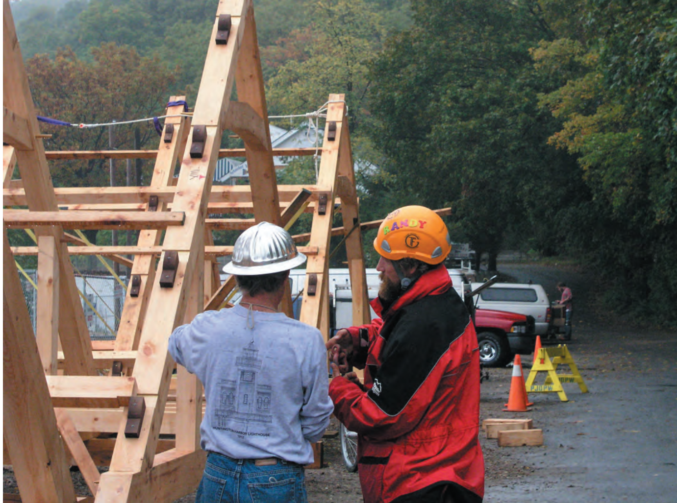
Fig. 1. Hardhats or safety helmets with or without brims are de rigueur at timber frame raisings. Chin straps are definitely useful. Note that stickers on hardhats must be of a compatible material and their numbers should be kept within reason to allow proper inspection of the hat.
