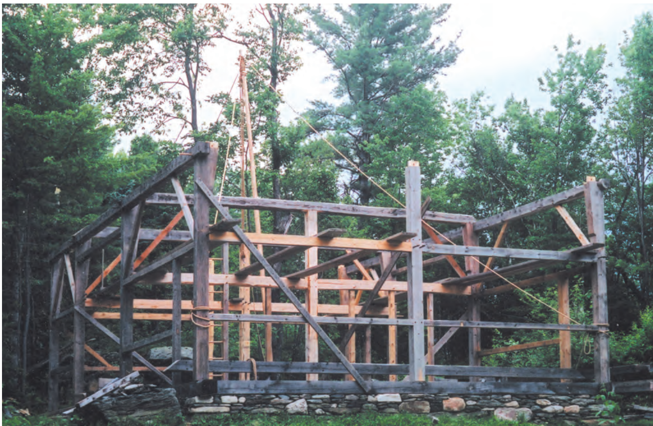
Fig. 8. Gin pole (now inside frame) is placed carefully for load block to hang plumb over destination. Tagline (slack at left) controls load.
