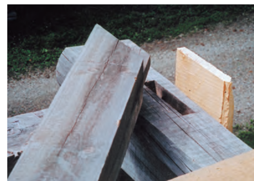
Fig. 10. Gable rafter pair with collar assembled over spaced planks on tie beams. Already erect, one intermediate rafter pair with raking struts was assembled piecemeal in position. Note notches for ridge and purlins. Detail below, closeup of stop nailed to tie to restrain rafter foot when truss is lifted.
