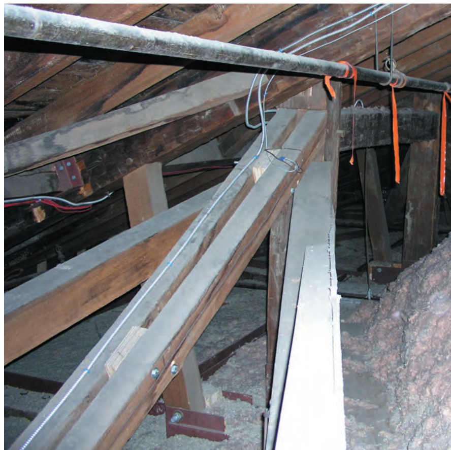
Fig. 25. Multiply braced queenpost trusses run the long way in the attic flanking the dome, to account for absent transverse kingpost truss.
