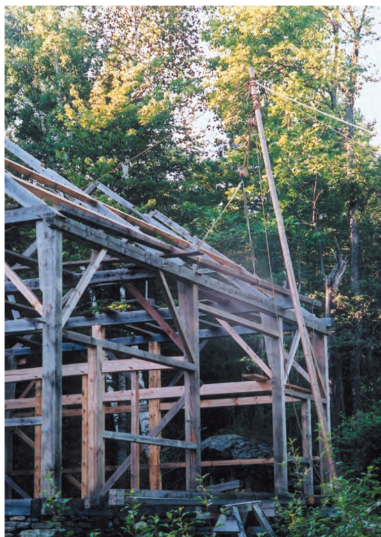
Fig. 12. Raising purlins with the gin pole and staging them on projecting tie beam ends left long for the purpose.
