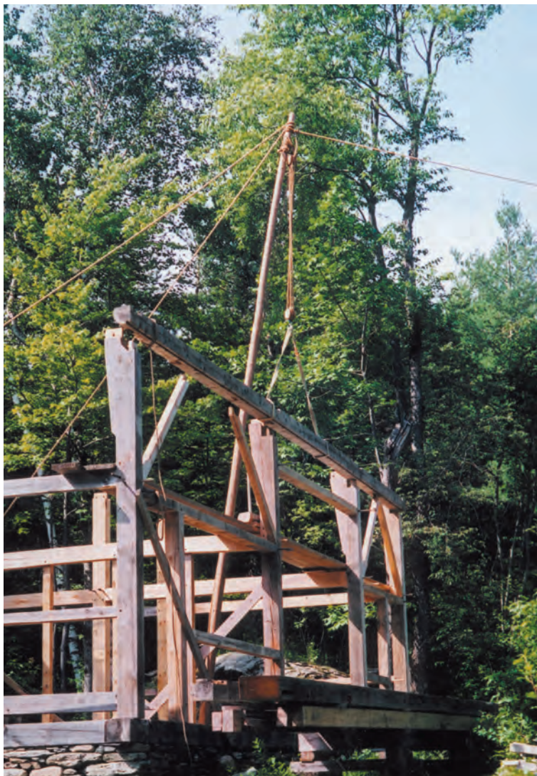
Fig. 8. Gin pole (now inside frame) is placed carefully for load block to hang plumb over destination. Tagline (slack at left) controls load.
