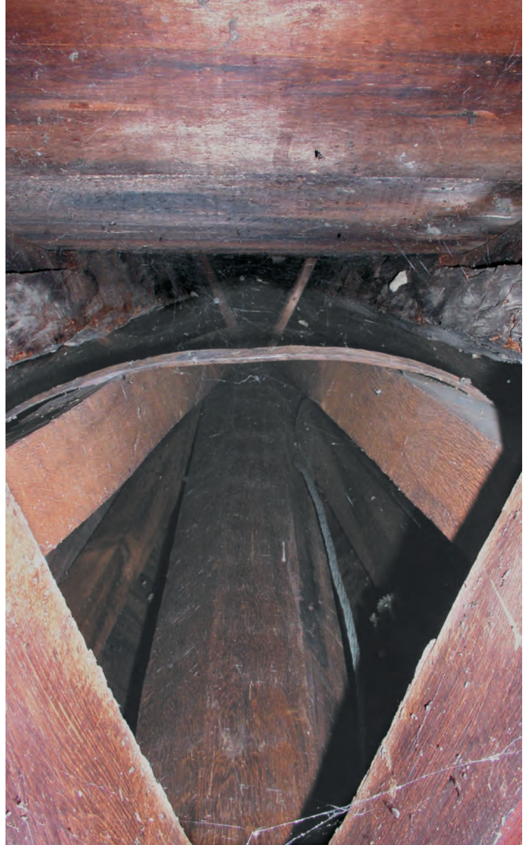
Fig. 23. View straight up into spire. Curved pine roof boards at top, oak mast at center, oak braces and spire rafters at left and right.
