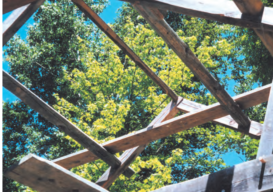
Fig. 14. Plank across purlins allows installation of lightweight ridge.
