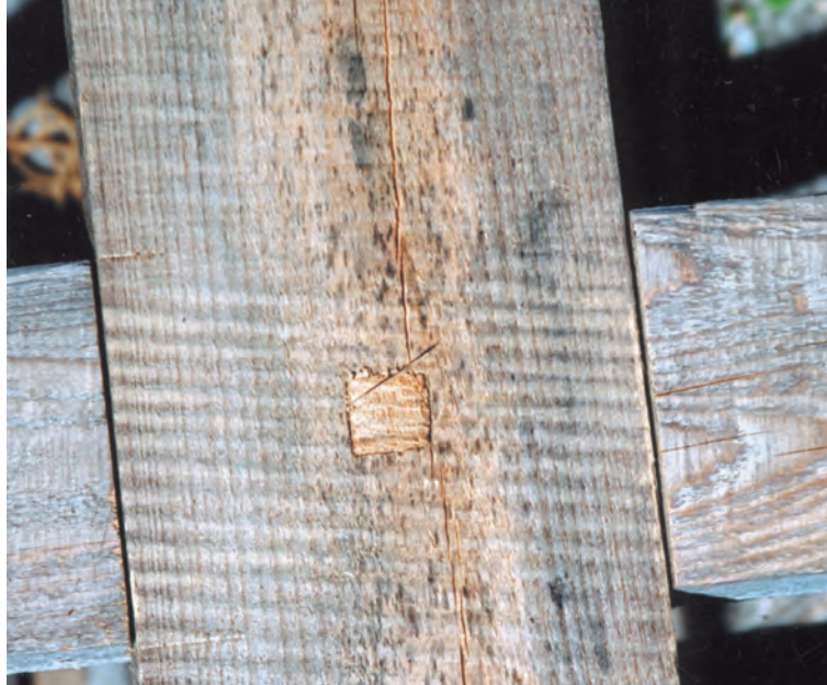
Fig. 13. Square ash pin securely grips pine purlin-to-rafter joint.
