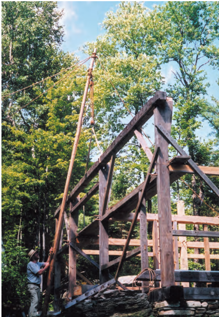
Fig. 6. Gin pole helps lift plate and position one end over a corner-post tenon. Planks give access for adjustments and brace insertion.
