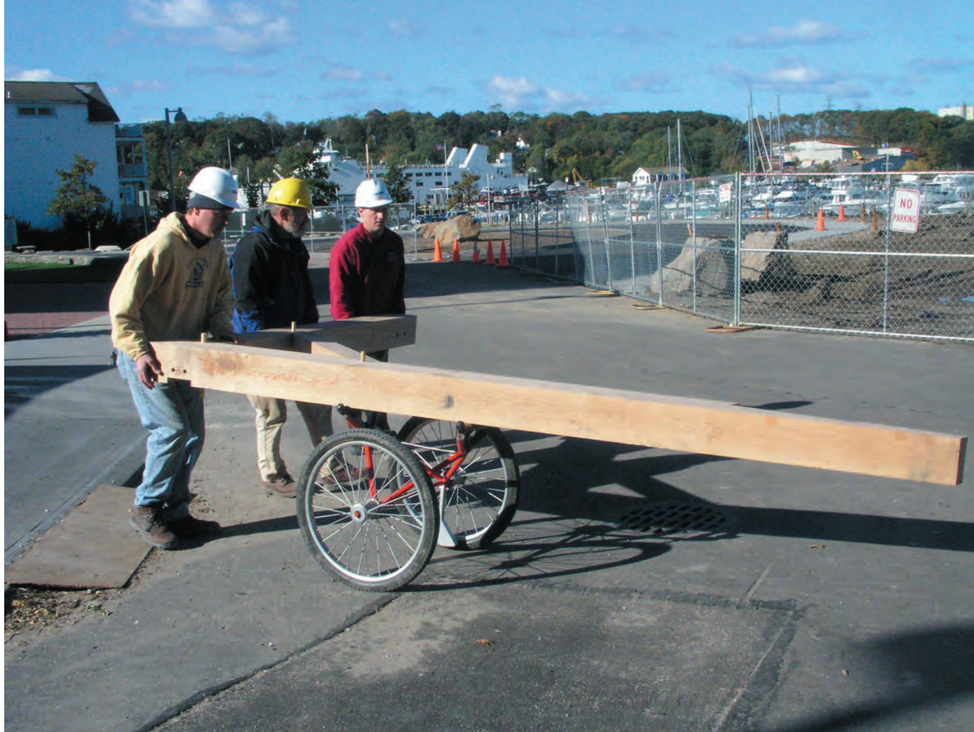
Fig. 8. Carrying an unbalanced load safely and restfully (at least one of the two men on the short beam is loafing). Everyone faces squarely forward and stands nearly upright; the cart takes the brunt of the load as the fulcrum between the long part of the post and the beam-brace assembly on the short part.
