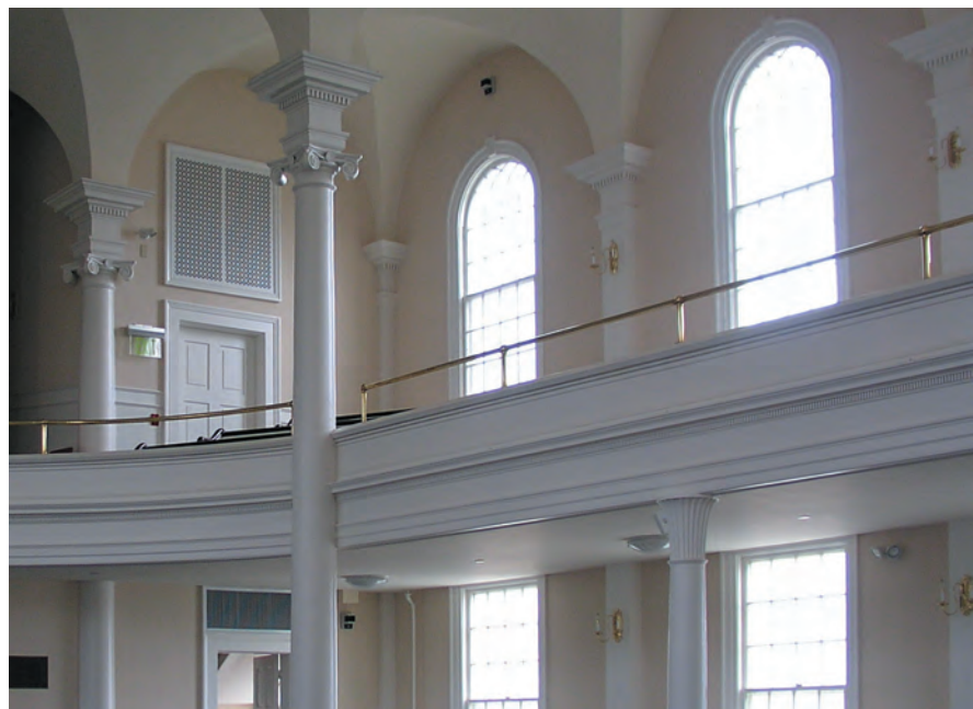
Fig. 1. Middlebury Congregational Church (1806–09), designed by Lavius Fillmore, stands at the top of a hill at an important road junction. Fig. 2, below, post at left rear rises through vaulting to help support a roof truss carrying back wall of steeple.
