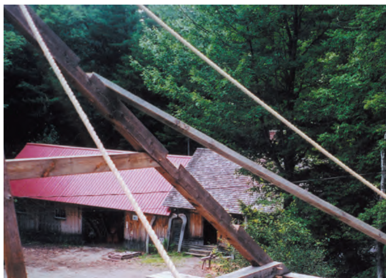
Fig. 11. Stay braces for rafters will keep roof framing plumb. With forethought, they would have been nailed to undersides of rafters.
