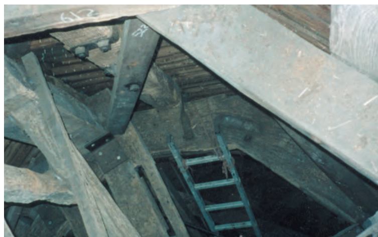
Fig. 15. Crooked timber exploited for octagonal spire framing.
