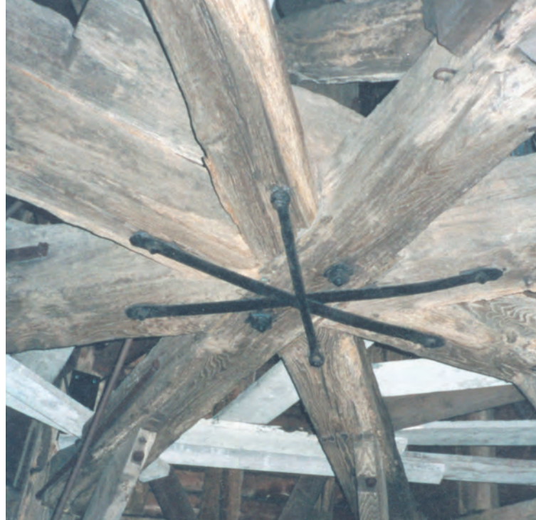
Fig. 14. Mast foot crab at St. Mary the Virgin at Cleobury-Mortimer.
