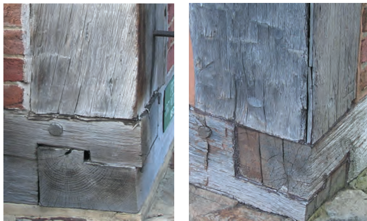
Fig. 4. Sill corner details in Salem, one coggled, one dovetailed.
