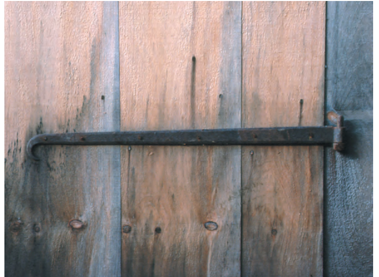
Fig. 8. Hinge straps (32 in. long on the big doors, 24 in. on the smaller doors) with decorative curled tips. Four 18th-century hinges were recycled from an old barn and additional new ones forged to match. Pintle (at right) with square tapered shaft was driven into doorpost.
