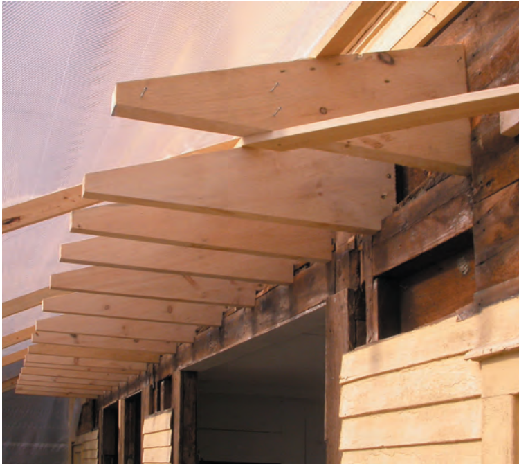
Fig. 3. Reconstruction of pentice roof followed discovery of telltale mortises in building. Temporary roof over work area allowed unhindered progress.
