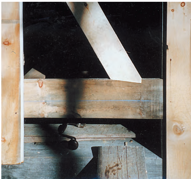
Fig. 7. Gain in lower batten for doorbrace. Sheathing is held back on post for door to make a seal on the hinge edge (at right).
