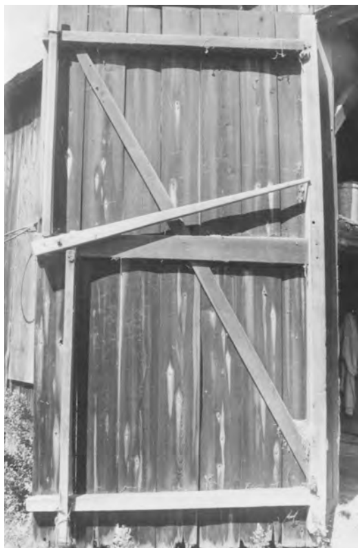
Fig. 3. Framed door in Savoy, Massachusetts, with ingenious lever-operated bolt.
