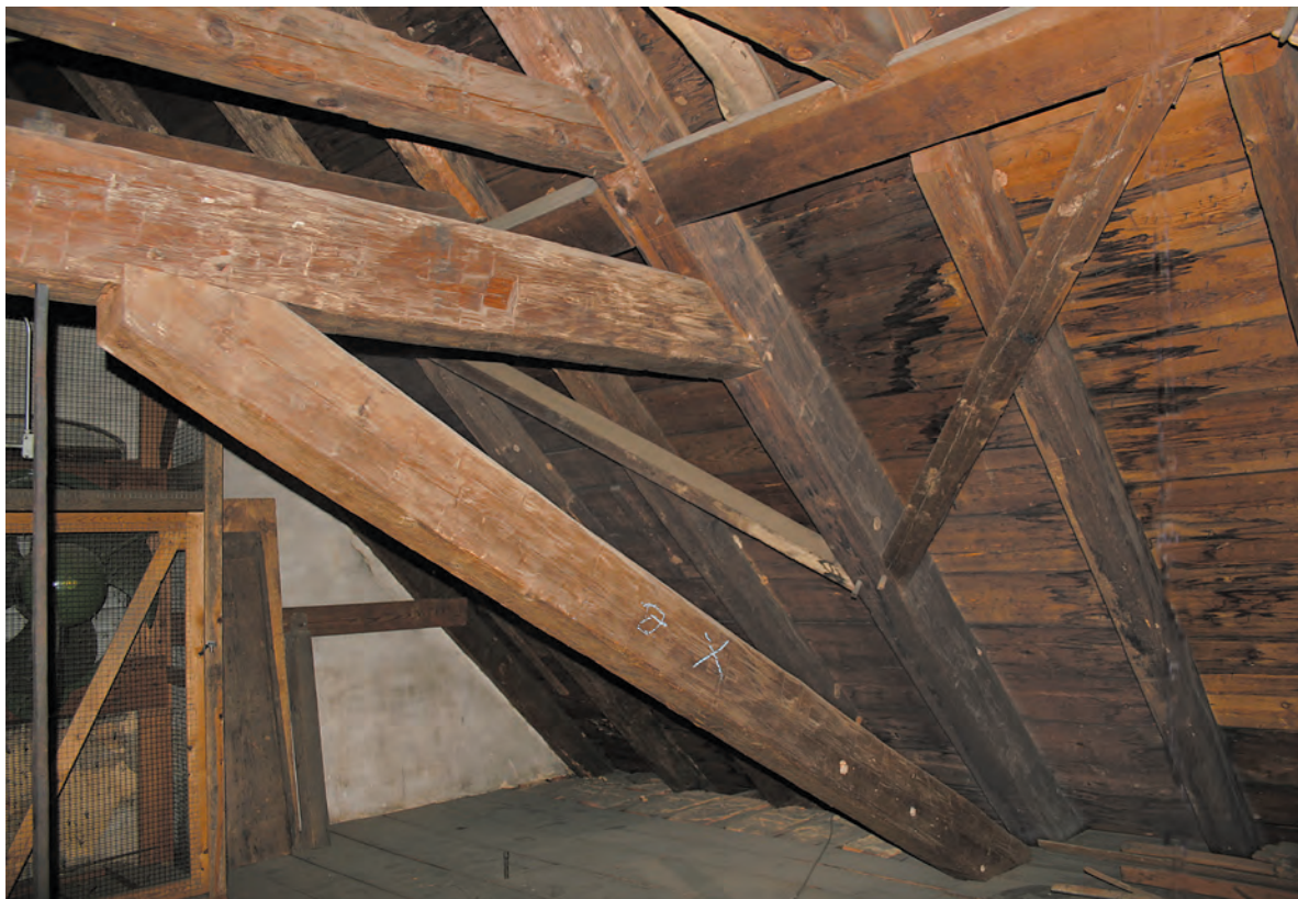
Fig. 10. Home Church principal rafters 8x12 carry tenoned and strutted purlins 5x6. Common rafters 5x7 run on 3-ft. centers. Strut, lower collar and rod at far left form part of truss to help hold up sanctuary ceiling.
