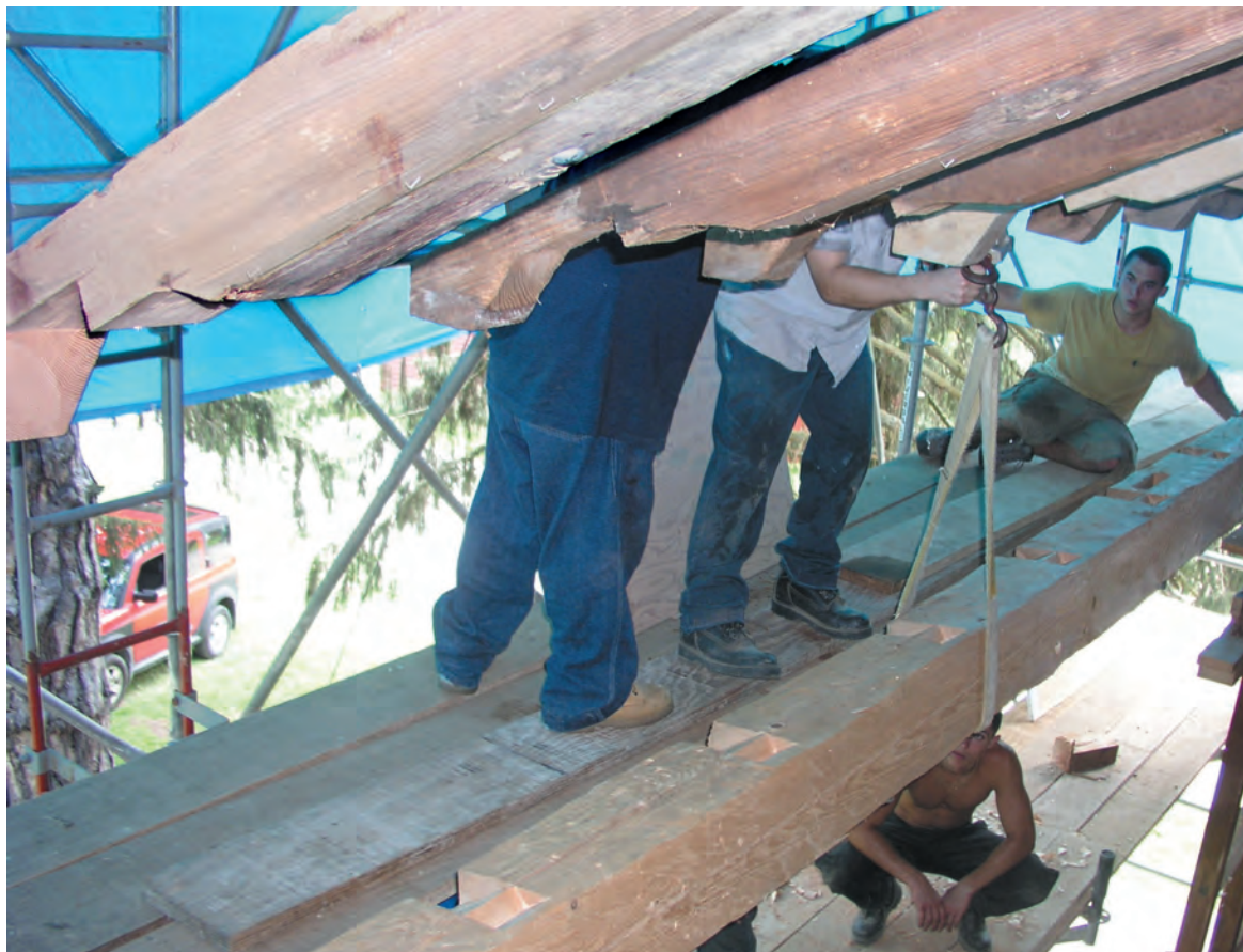
Fig. 5. After scarfing-on of new rafter ends, the repair sequence called for insertion of the new step-lapped plate from below. Plate will be hoisted further and blocked up on cribbing spanning from the attic floor to the staging, then slid outward to engage the rafter feet.
