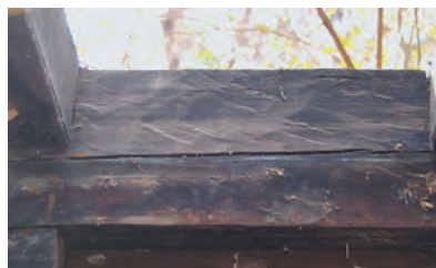
Fig. 3. Dressed and beaded joists in Brown House.
