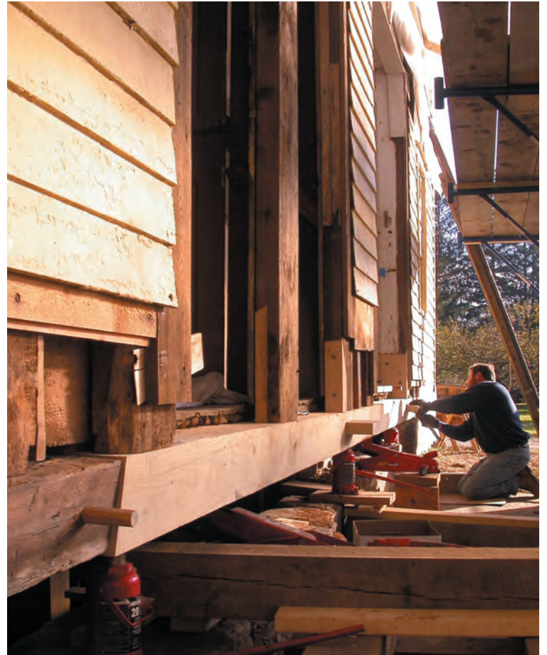
Fig. 5. Scarfed-in sill in place, Matt Duffin drives in free tenon to secure floor beam meeting sill. To his left, a second free tenon remains proud.
