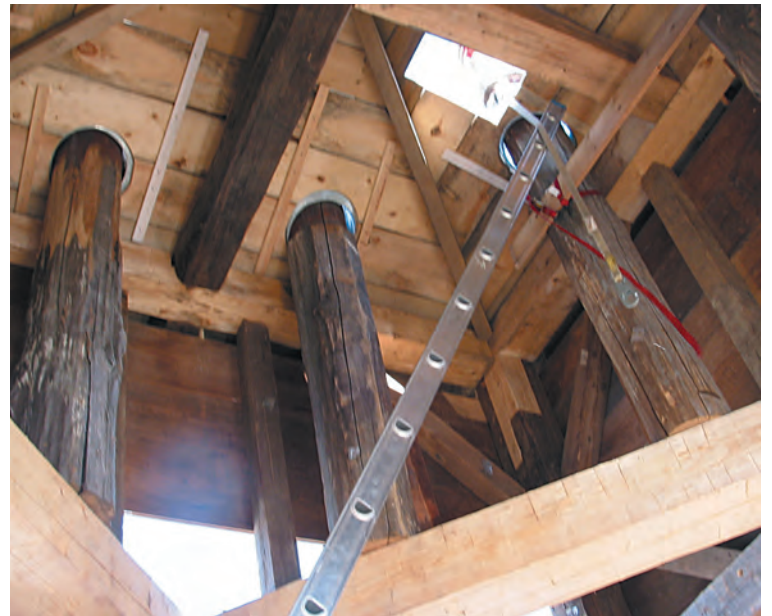
Fig. 1. Steeple columns are turned where they emerge to view, left merely debarked where they remain concealed.
