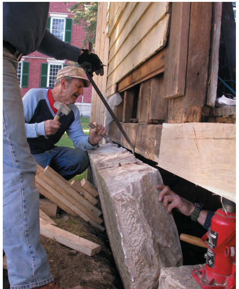
Fig. 6. Persuading a granite foundation stone to enter under the sill. The late Ed Mottarella chamfers the arris to ease the way.
