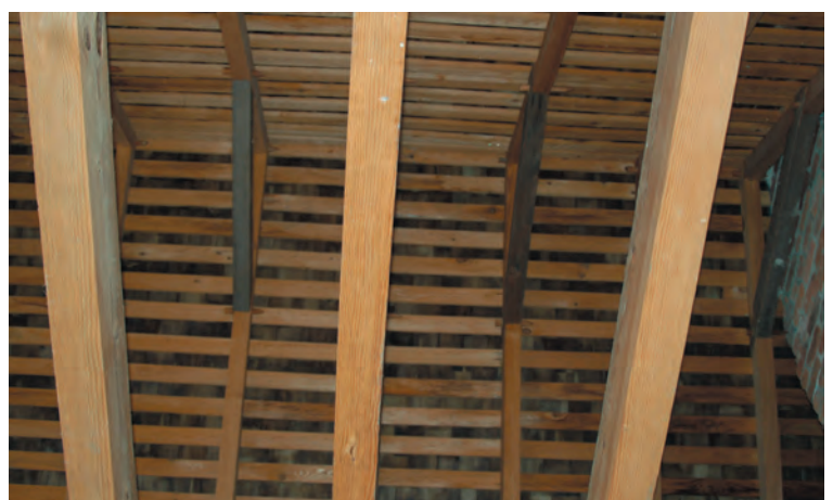
Figs. 8–9. Reconstructed open-ceiling kitchen at Hope Plantation. Ventilation overhead relieved heat of a wood-fired southern kitchen.
