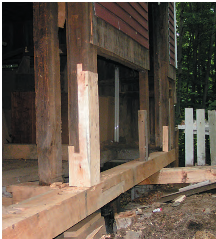
Fig. 2. Repair or replace? Here, one choice for sill, the other for posts.
