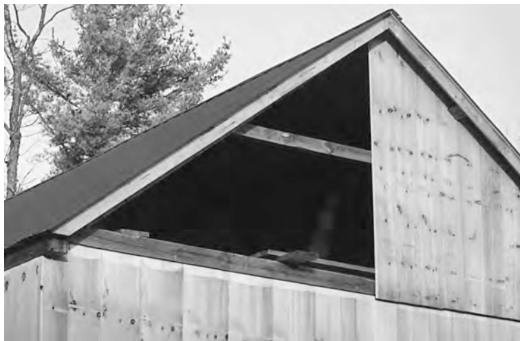
Fig. 2. Most gable boarding could be done from inside while standing on planks. A few last pieces near the eaves went on from a ladder.
