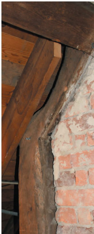
Fig. 8. Crucks post supporting purlin. Rafter is modern.
