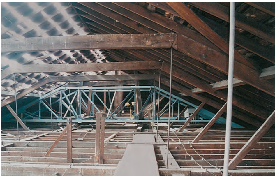
Fig. 3. A pair of light steel trusses now support the steeple in the attic of St. Philip's Moravian Church. Main roof trusses are composite vernacular queenrods.
