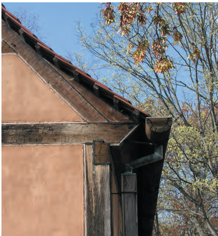
Fig. 2. Miksch House, 1771, a Fachwerk house with the characteristic roof pitch “kick” at the eaves. Note coggled tie beam at front plate.
