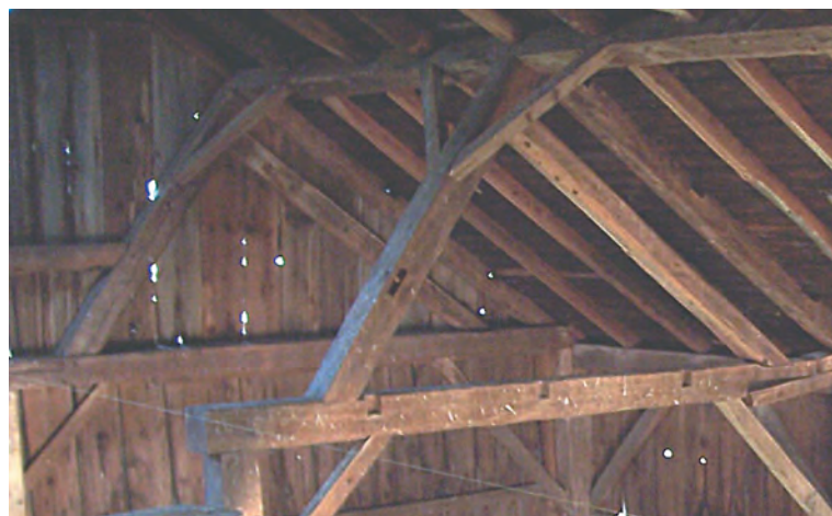
Fig. 2. English barn cut and spread apart, with new roof framing.
