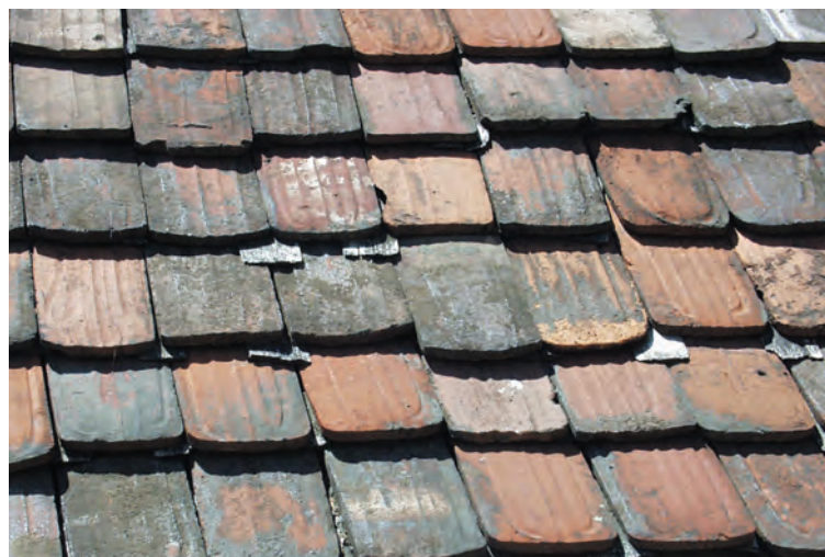
Fig. 3. Roof tiles are laid in straight files without staggering the joints. Instead, thin wooden slips under the joints shed onto one another.
