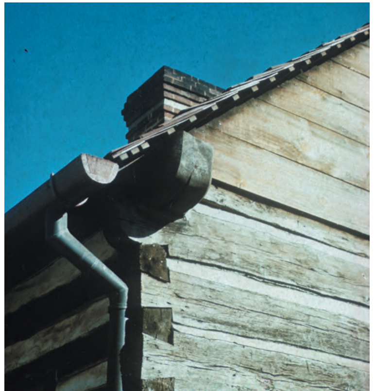
Fig. 1. The Lick-Boner house, 1787, Salem, N.C. Mature chinker log construction with hewn logs and dovetailed corners.
