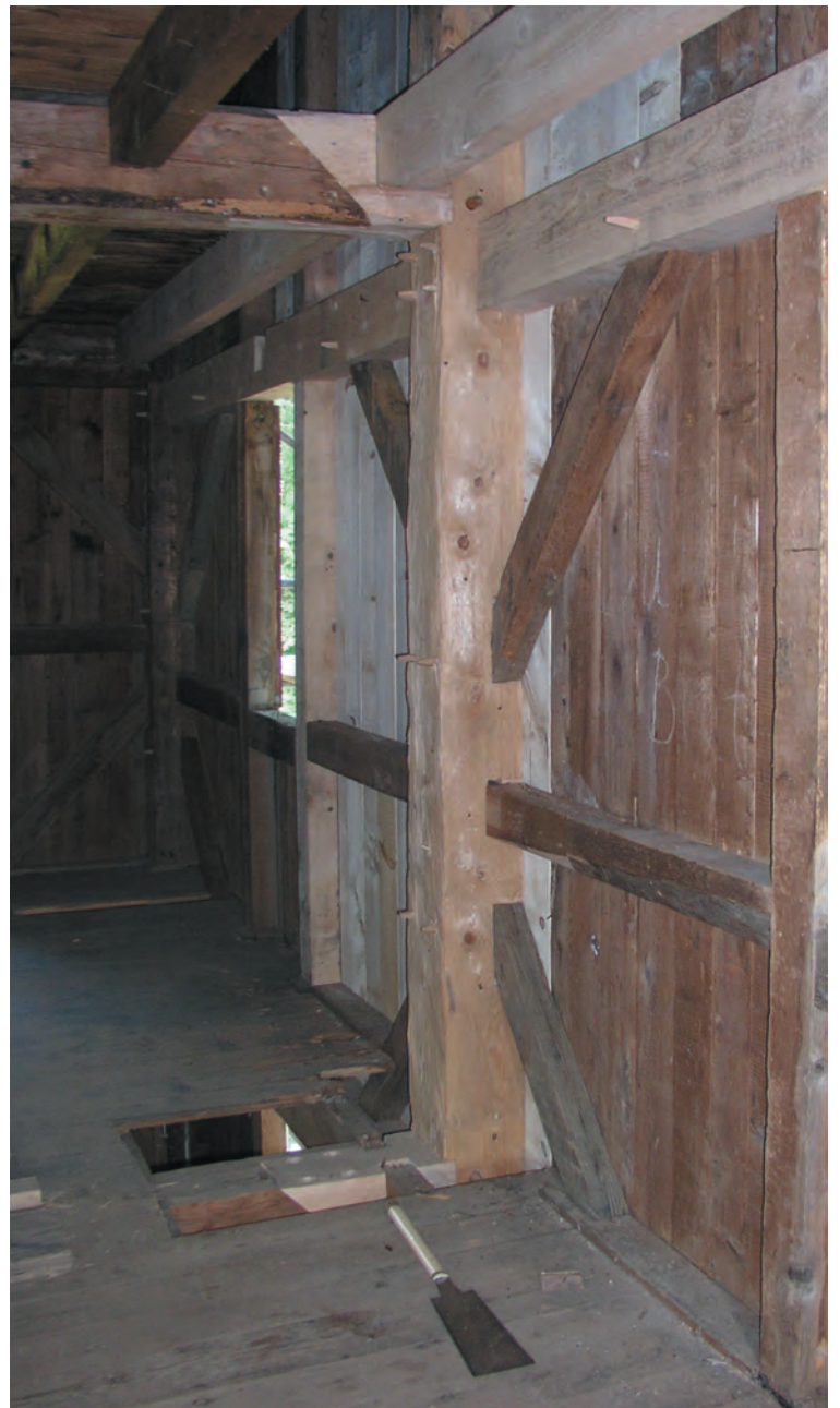
Fig. 4. Wall repairs shown above included new posts, girts and sheathing as well as carefully scarfed tie beam ends. Some braces, apparently original, were recycled from a demolished Shaker structure.
