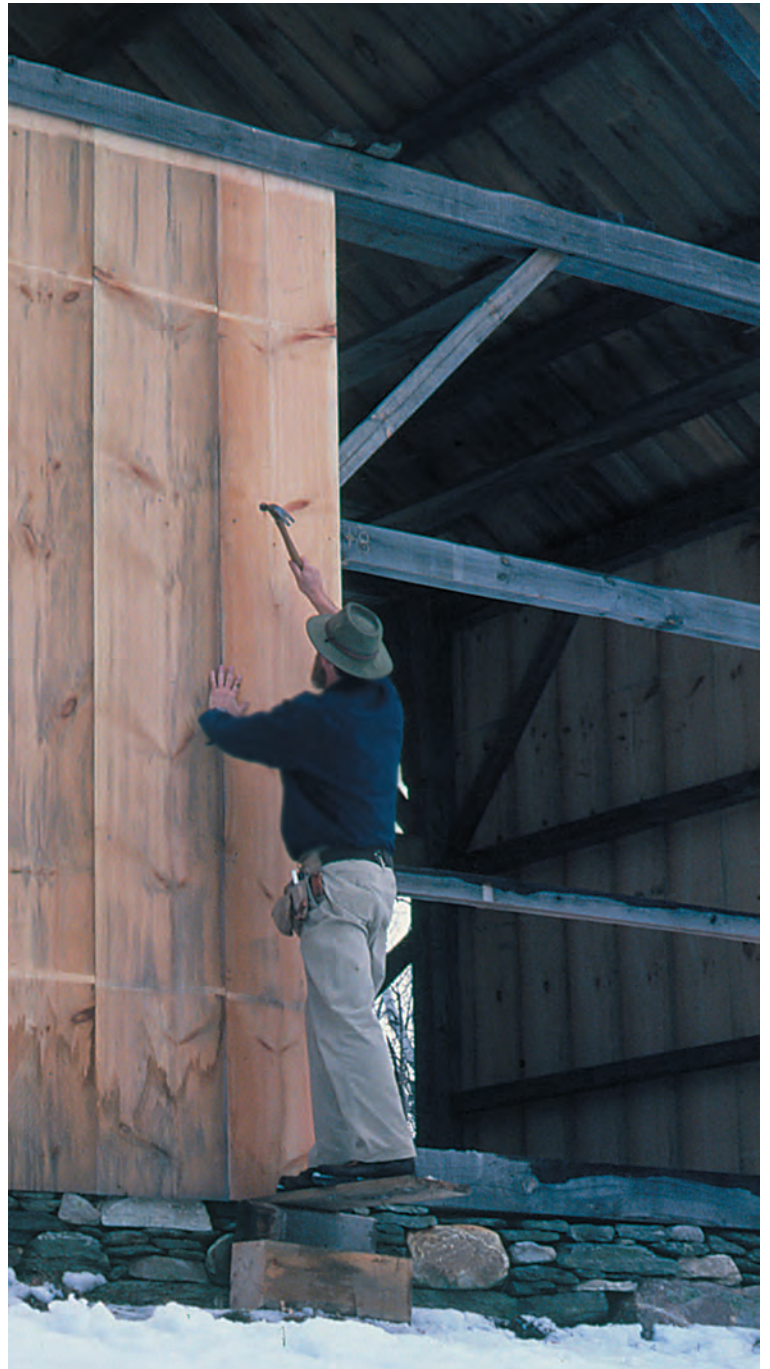
Fig. 1. Wide flitch-matched pine boards make quick work of the south gable end. Most of the boards had to be reduced slightly at their tops.
