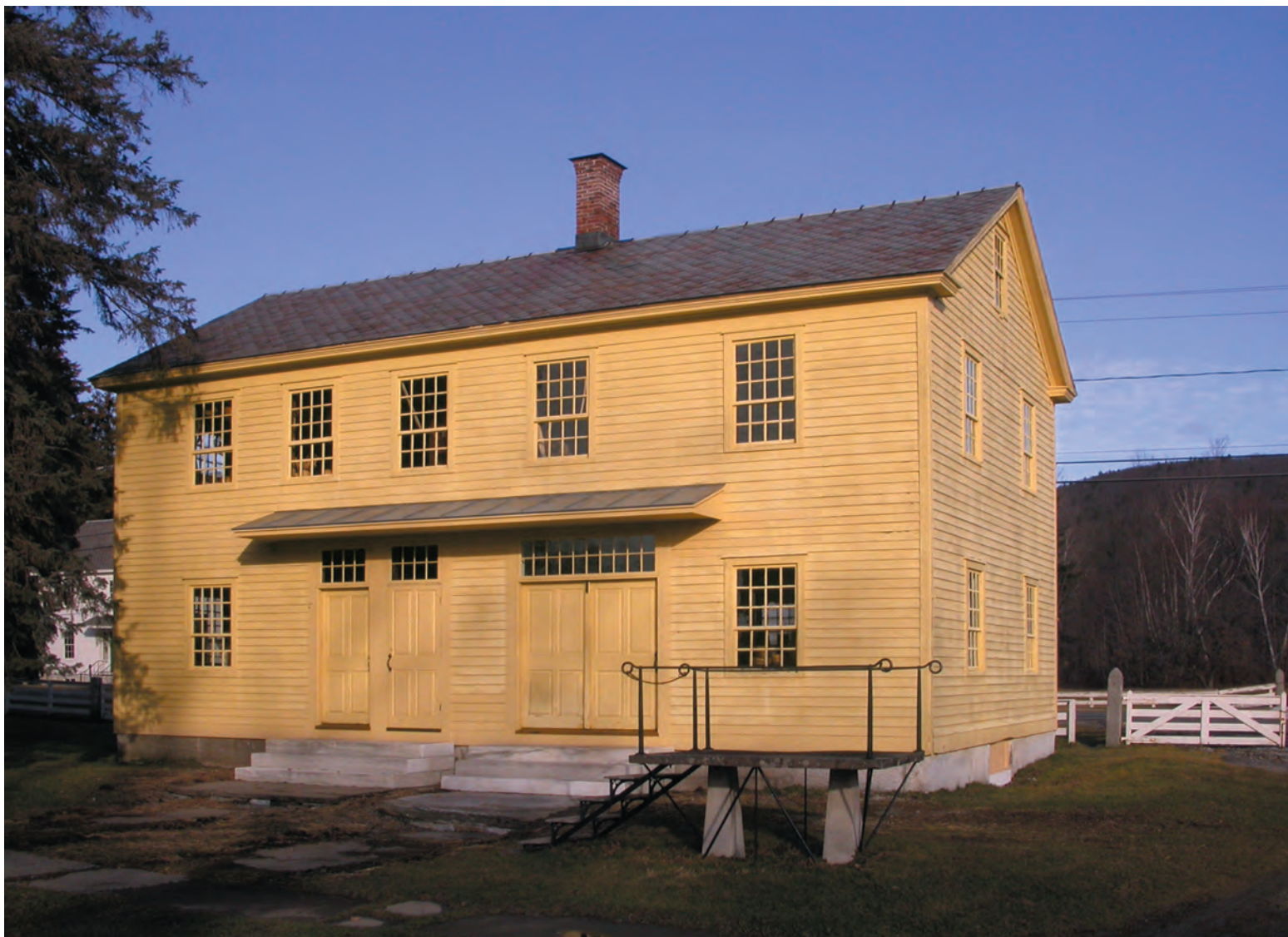
Fig. 1. The Brethren's Shop at Hancock Shaker Village repaired, with scarfed-in sills and posts, woven-in exterior finish and a new pentice roof to protect the entry. The iron platform on posts in the foreground is a carriage mount.
