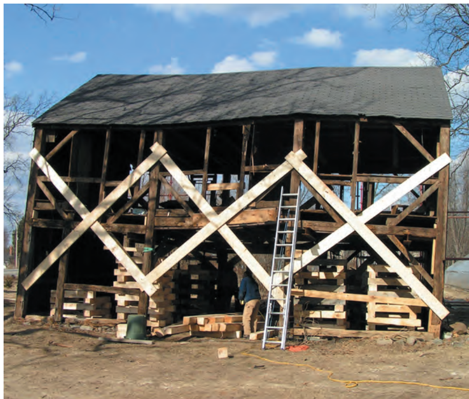
Fig. 1. Stabilizing a building can effectively replace its functional elements.
