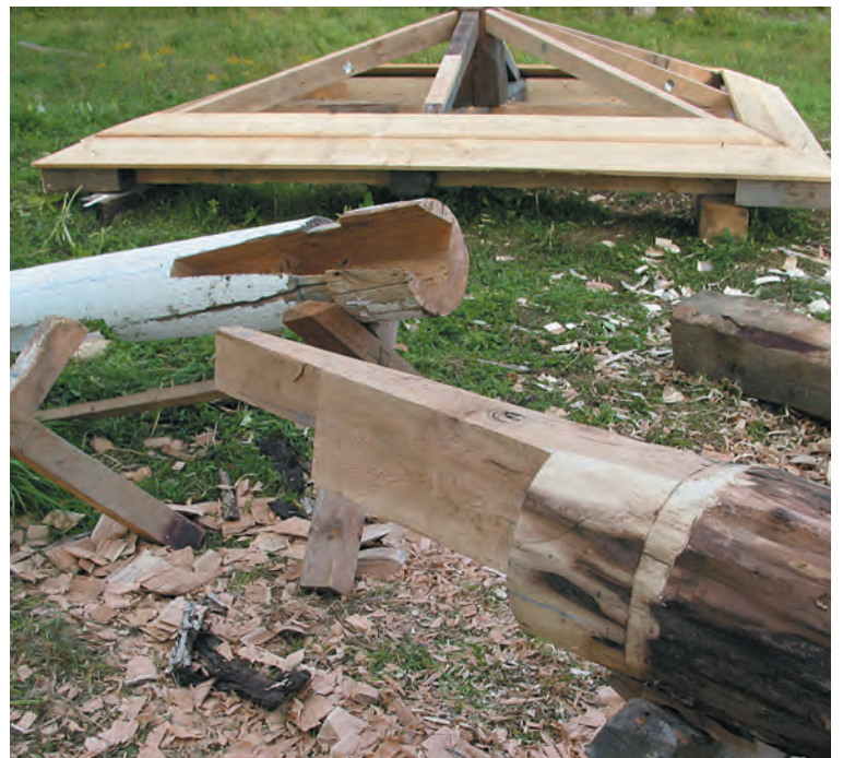
Fig. 2. Scarfing painted remnant column to new base. Newly re-framed tower roof, partly boarded, in the background.
