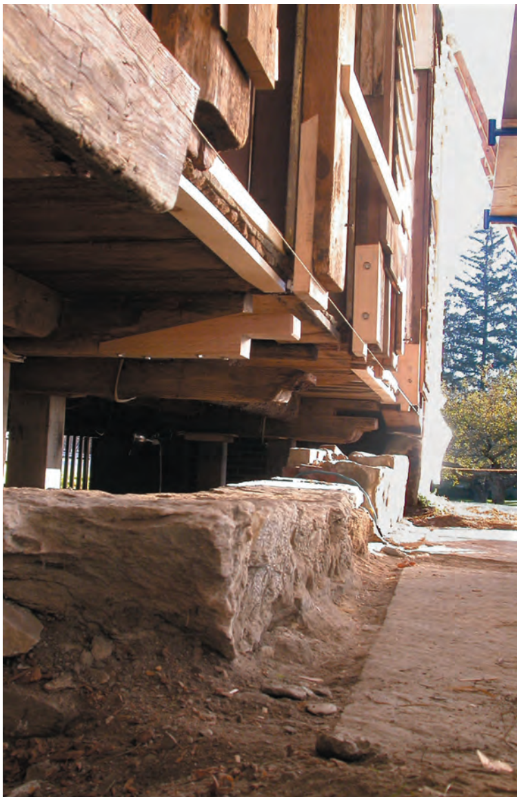
Fig. 4. Sill and foundation stone removed, repairs advanced on girder and post ends.
