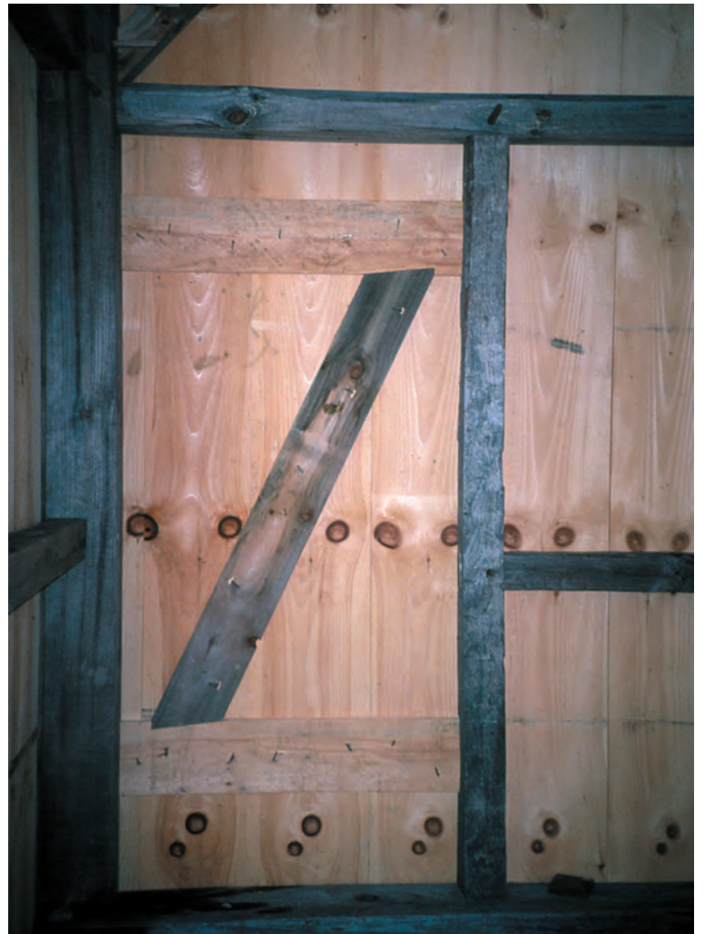
Fig. 9. Completed animal door viewed from inside. Clinched nails holding strap hinges and sheathing can be seen on battens and let-in brace. Flitch-matched sheathing boards form striking patterns.
