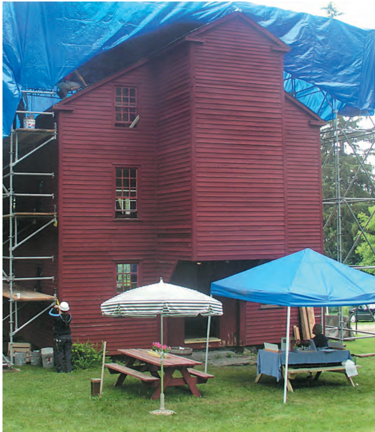
Fig. 3. Granary was fully staged and, with the roof wide open, tarped to protect interior surfaces and time-consuming frame repairs. Lunch was taken in style.
