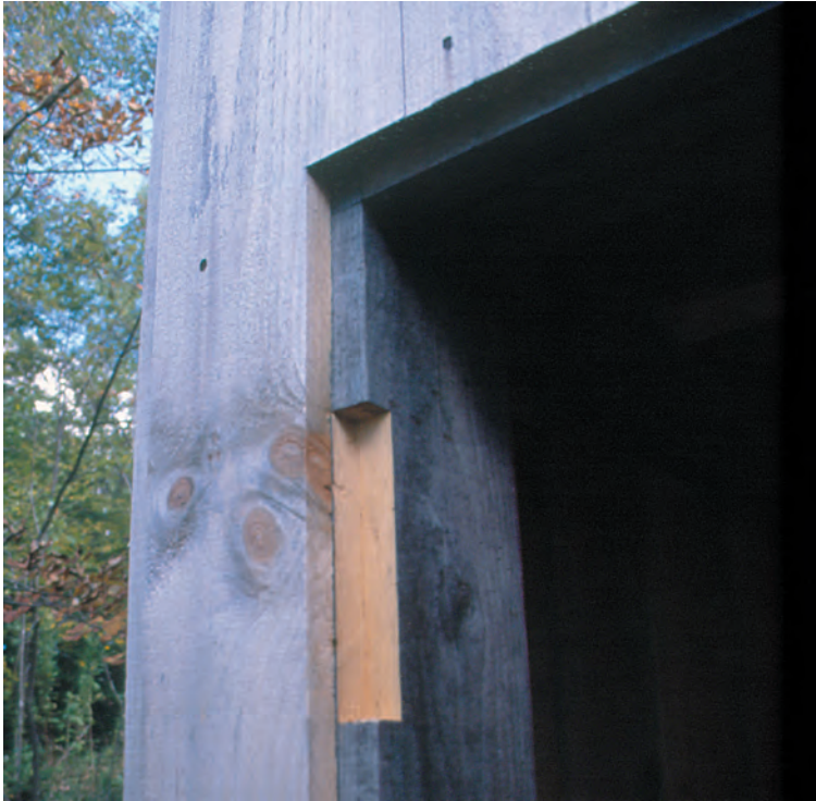
Fig. 6. Rabbeted notch in doorpost for an upper batten.
