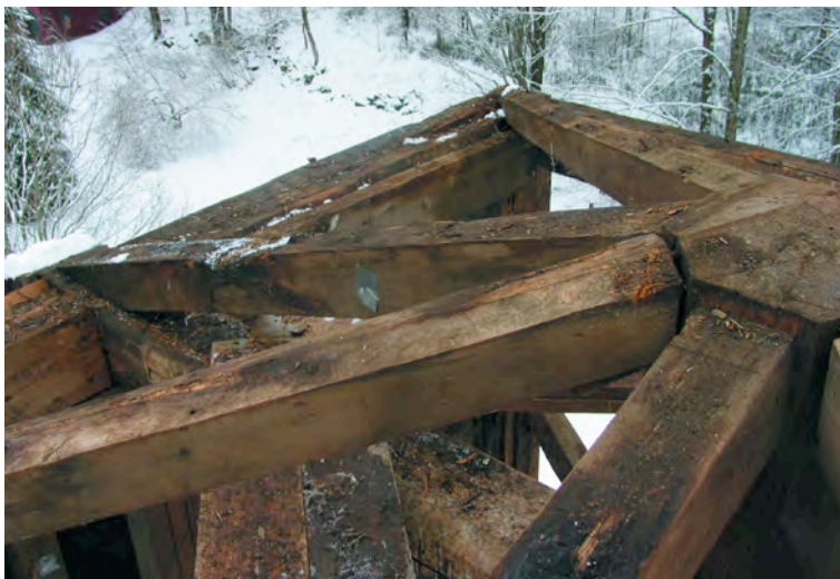
Fig. 2. Original South Woodstock bell deck. Since belfry is open to weather on four sides, deck must be framed and sheathed to shed water. Rafters measure 4 \times 4\frac{1}{2} , hips 3\frac{1}{2} \times 5 . Short kingpost is 14 in. across flats.
