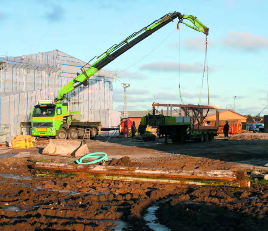
Fig. 9. Unloading trusses at site. Building underway is fully enclosed.
