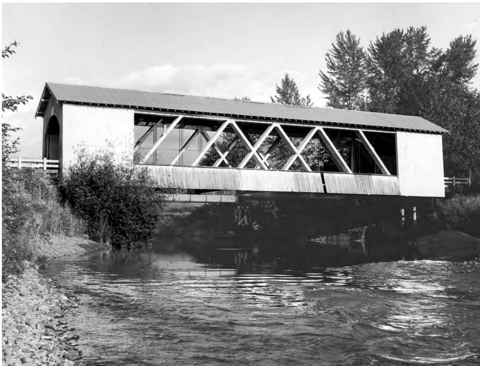
Fig. 5. Gilkey Bridge, Linn County, Oregon, built in 1939, with open sides but covered bottom chords. In the background (visible under the highway bridge) is a railroad bridge, itself once covered.
