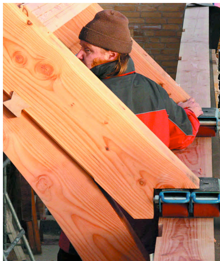
Fig. 11. Stefan Hildebrand rolls truss to position on skates. Pairs of shoring jacks assisted removal of skates and final descent of truss.
