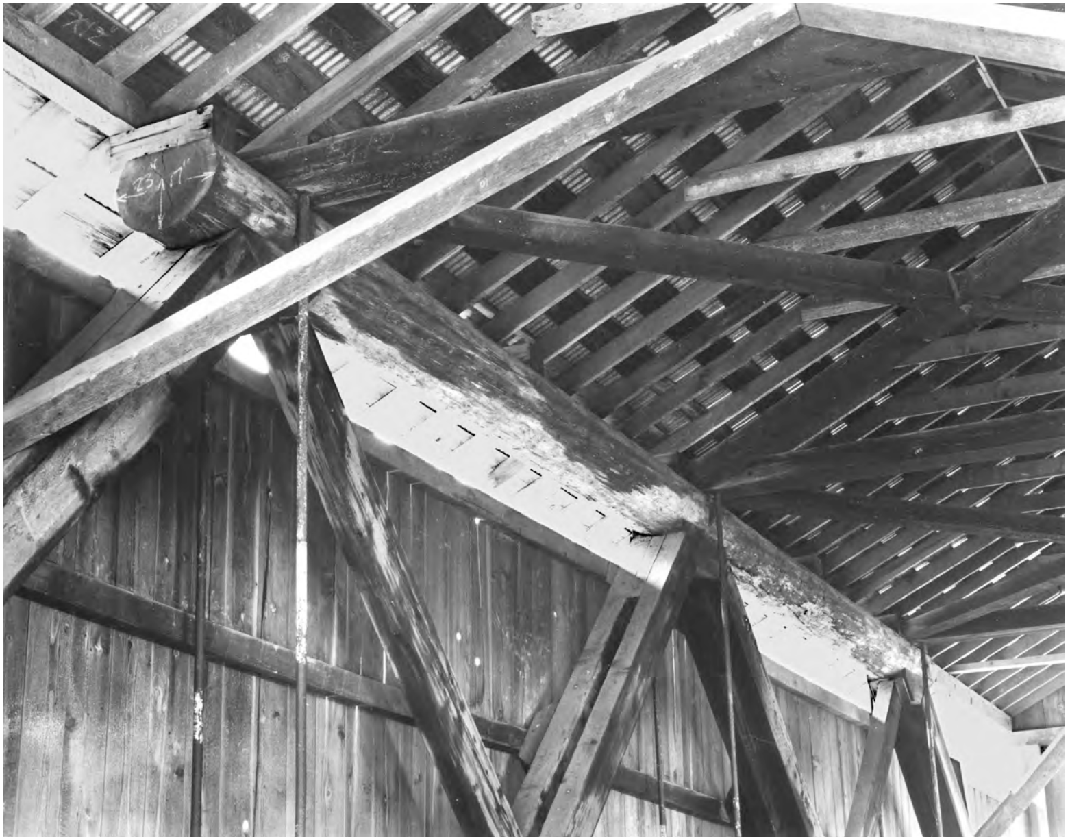
Fig. 8. Top chord of Cavitt Creek Bridge (in fact over Little River), Douglas County, Oregon, built in 1943. Use of a log is impressive but unusual; standard practice was to square the timbers. Dimensions on near end were probably added by inspectors during load-limit calculations.
