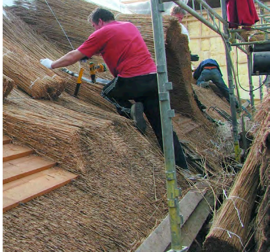
Fig. 14. Algis Kucinskis wiring down bundles between dormer windows, thatching boss Michael Jahrle just visible behind thatched dormer, Ramunas Lukasuskas busy at the far end (see also Fig. 13).
