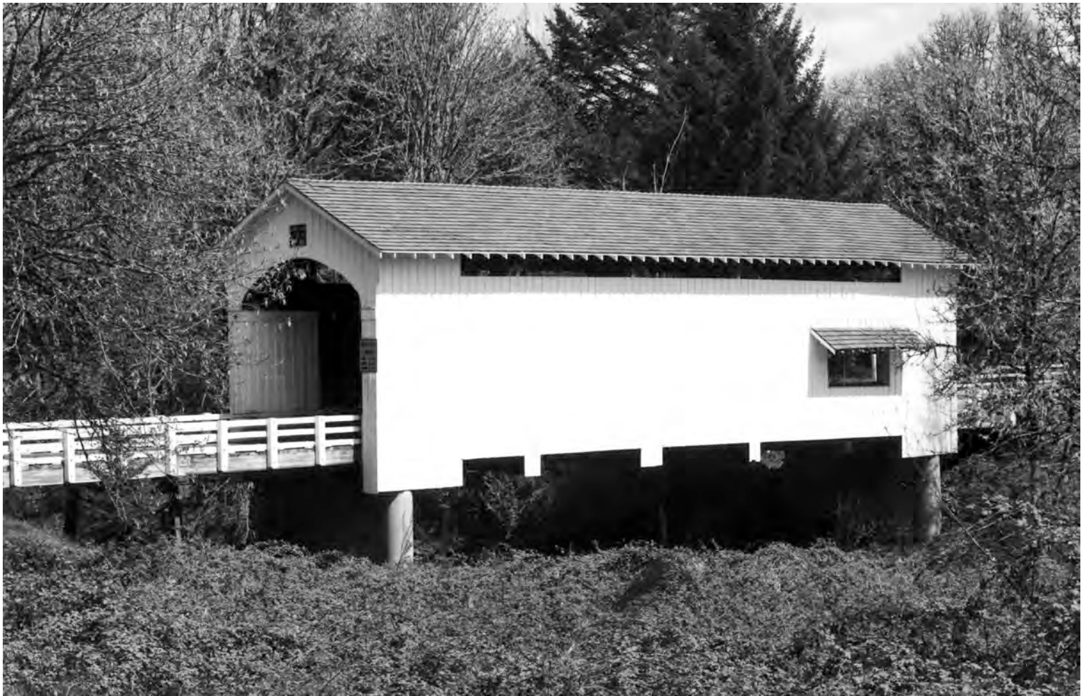
Fig. 6. Earnest Bridge, Lane County, Oregon, built in 1938. Far end opens onto curve in road; note window for visibility.
