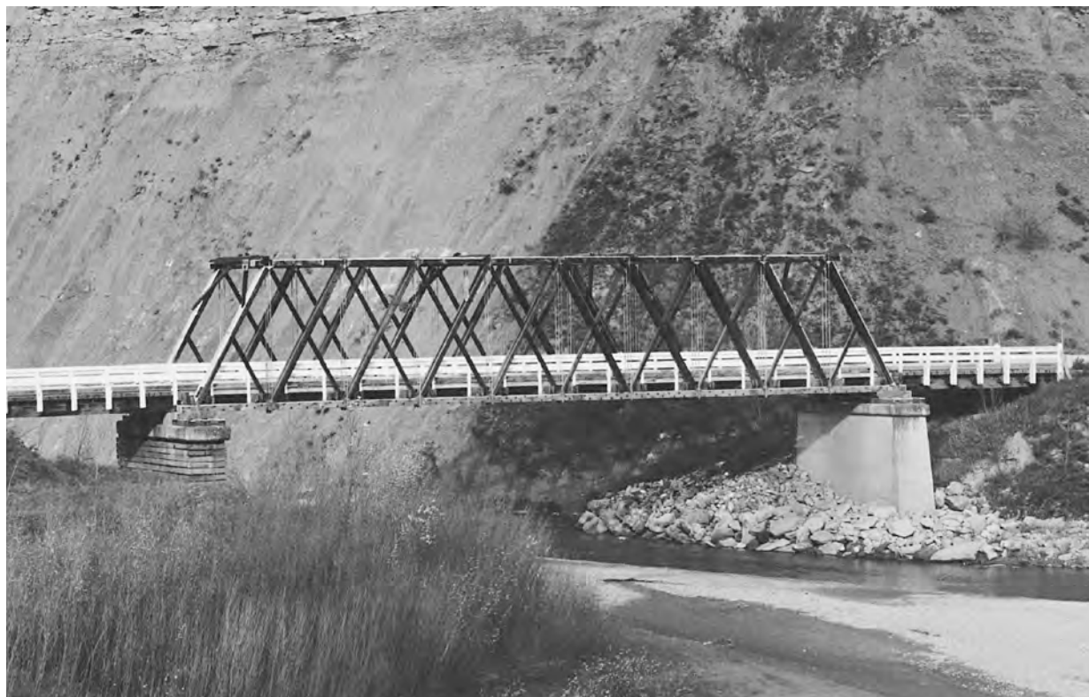
Fig. 3. Moose Mouth Bridge over Alces River south of Clayhurst, B.C., Canada, built in 1961. End panels are cut off such that top chords end just past last set of rods. Howe trusses built in British Columbia since the 1930s used chords fabricated from smaller sticks pinned with sections of steel pipe like treenails, with no space between sticks.
