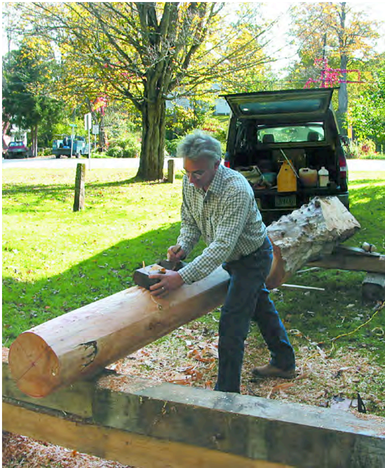
Fig. 9. Author smooths one of two new replacement columns, laid out, sawn, shaved and planed rather than turned as were originals. Bully surface where left rough suggests difficulty of finding good butternut today.
