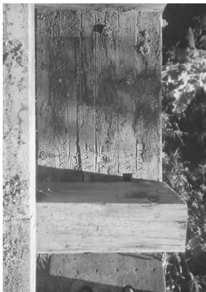
Fig. 4. Marriage marks on shear blocks and bottom chord, top view looking down. Tracey Mills Bridge, Carleton County, New Brunswick, built in 1936. Note angle block at bottom.
