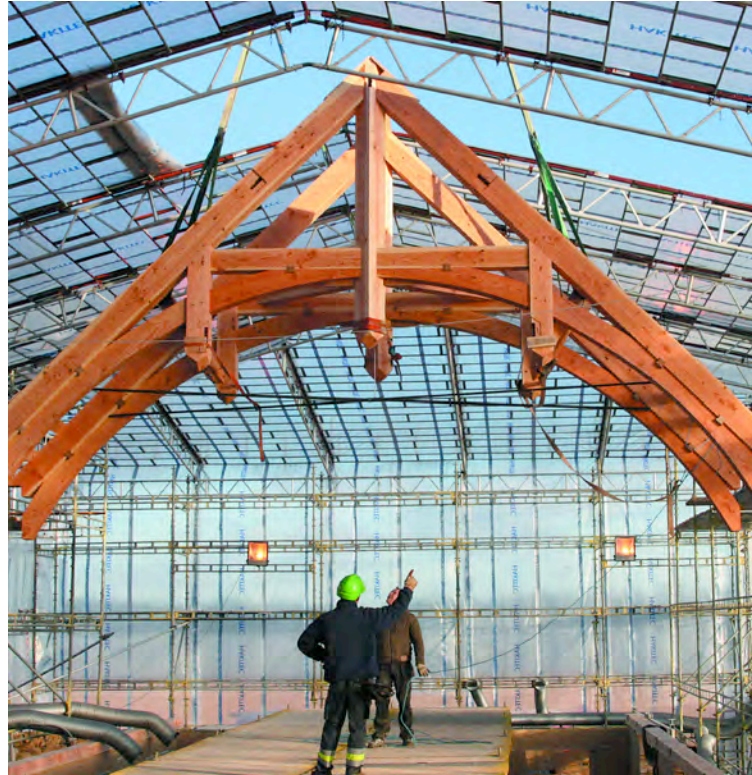
Fig. 10. Double truss of Danish Douglas fir flown in through roof.
