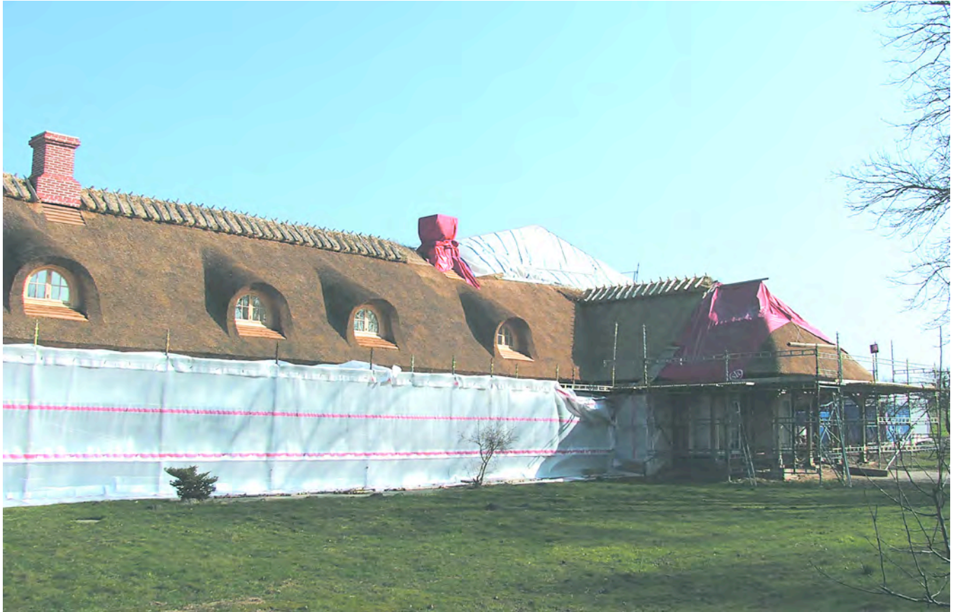
Fig. 1. Thatched house under construction at Stubbegaarden, Denmark. Great room is under tarped scaffold roof.
