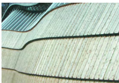
Fig. 4. Gridshell construction details. Above, assembling and bolting together a node with patented system of plates. Above right, European larch glulam arch over entrance. At right, cladding of UK-grown red cedar. Boarding is laid to account for expected cupping.
