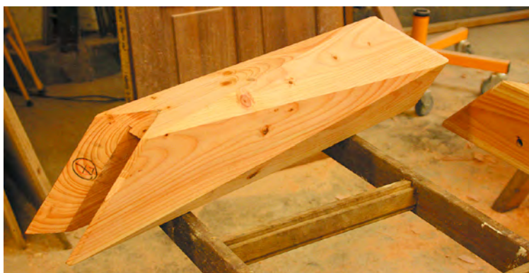
Fig. 7. Short brace is rotated to simplify connection at one end, with serious consequences at the other.
