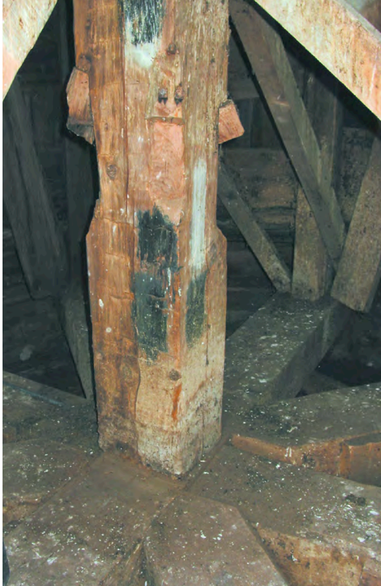
Fig. 17. Mast for Strafford spire is footed in eight-legged crab in belfry roof, which also forms base of octagonal lantern.
