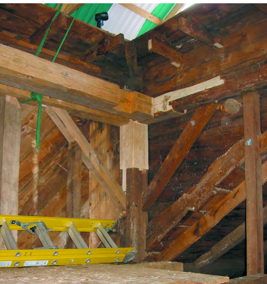
Fig. 13. Tower required numerous scarfed repairs and whole-member replacements, using structural staging as jacking base for insertions.
