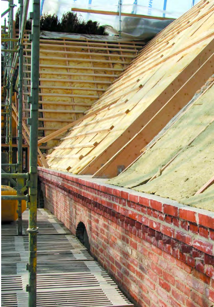
Fig. 12. Mineral wool thoroughly insulates cavities in roof and walls against air and fire movement. Treated fiberglass blanket will cover roof battens before application of thatch. All masonry is lime-mortared.
