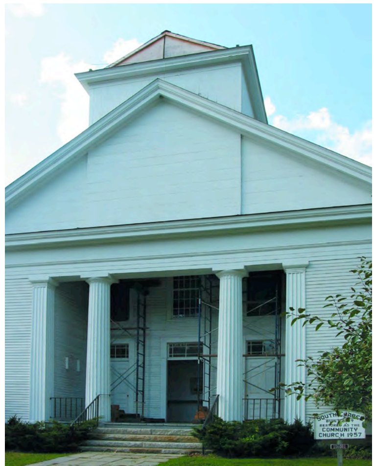
Fig. 4. Greek Revival facade of South Woodstock Community Church after removal of steeple upper stages and capping of tower with light temporary roof. Church was built in 1839 as South Woodstock Congregational Chapel and took its present name in 1957.
