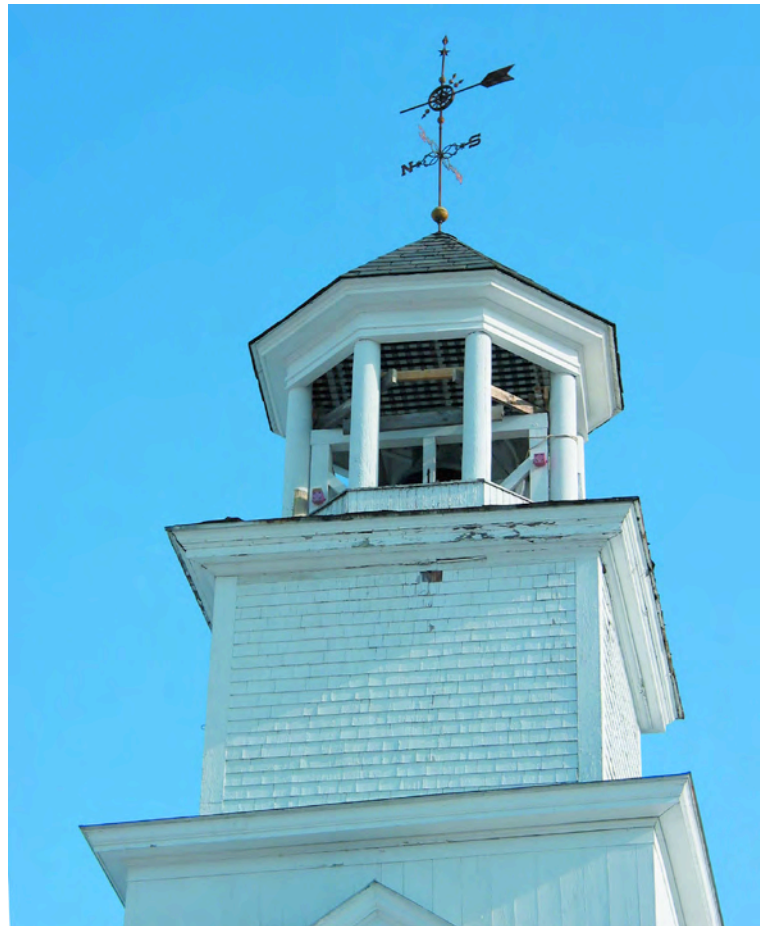
Fig. 3. Steeple of South Woodstock church before repairs. Compound tilt, somewhat unusual, includes typical backward lean from overloading of the first interior truss combined with sideward lean from rotting posts and sleepers along the south side of the tower.
