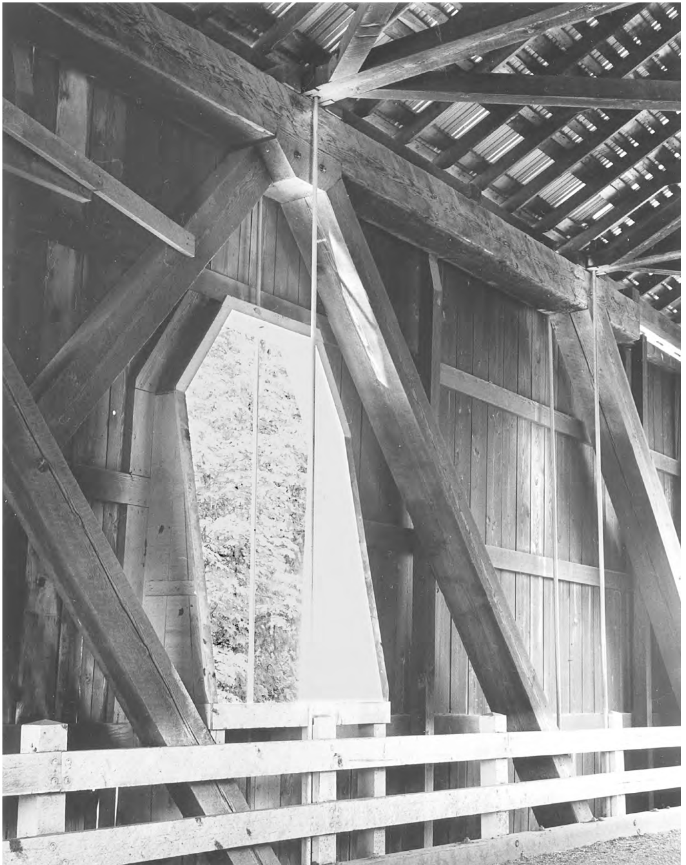
Fig. 9. Braces and counterbraces connected to top chord with an angle block. Block is let slightly into chord to prevent it from shifting. Oregon occasionally used iron angle blocks in its 20th-century covered bridges, but much more often used wood. At far right, note batter brace joint in top chord made with a dap instead of a block. Top chord is hand-hewn while braces are sawn. Hoffman Bridge, Linn County, Oregon, built in 1936.
