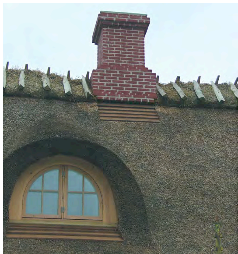
Fig. 15. Crowsfeet made of cleft oak saplings bolted together hold down thatched ridge by their own weight. Wooden boarding laid shingle fashion serves as exterior flashing under window and chimney.
