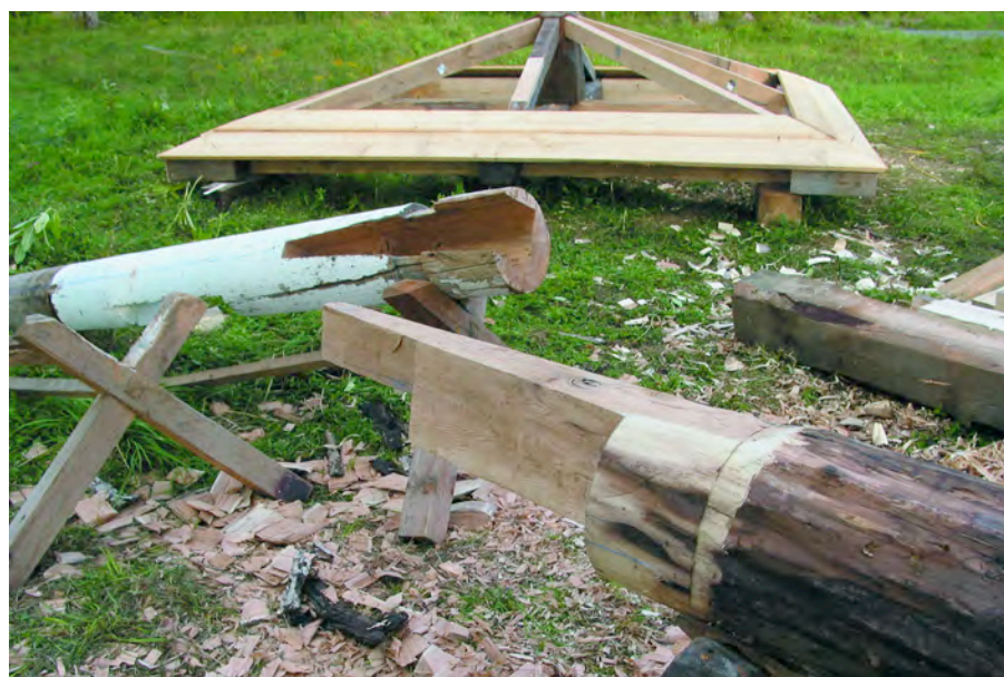
Fig. 8. Distinctive scarf joint in progress between new column bottom and old column top. Mostly rebuilt bell deck in the background.
