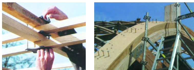
Fig. 4. Gridshell construction details. Above, assembling and bolting together a node with patented system of plates. Above right, European larch glulam arch over entrance. At right, cladding of UK-grown red cedar. Boarding is laid to account for expected cupping.
