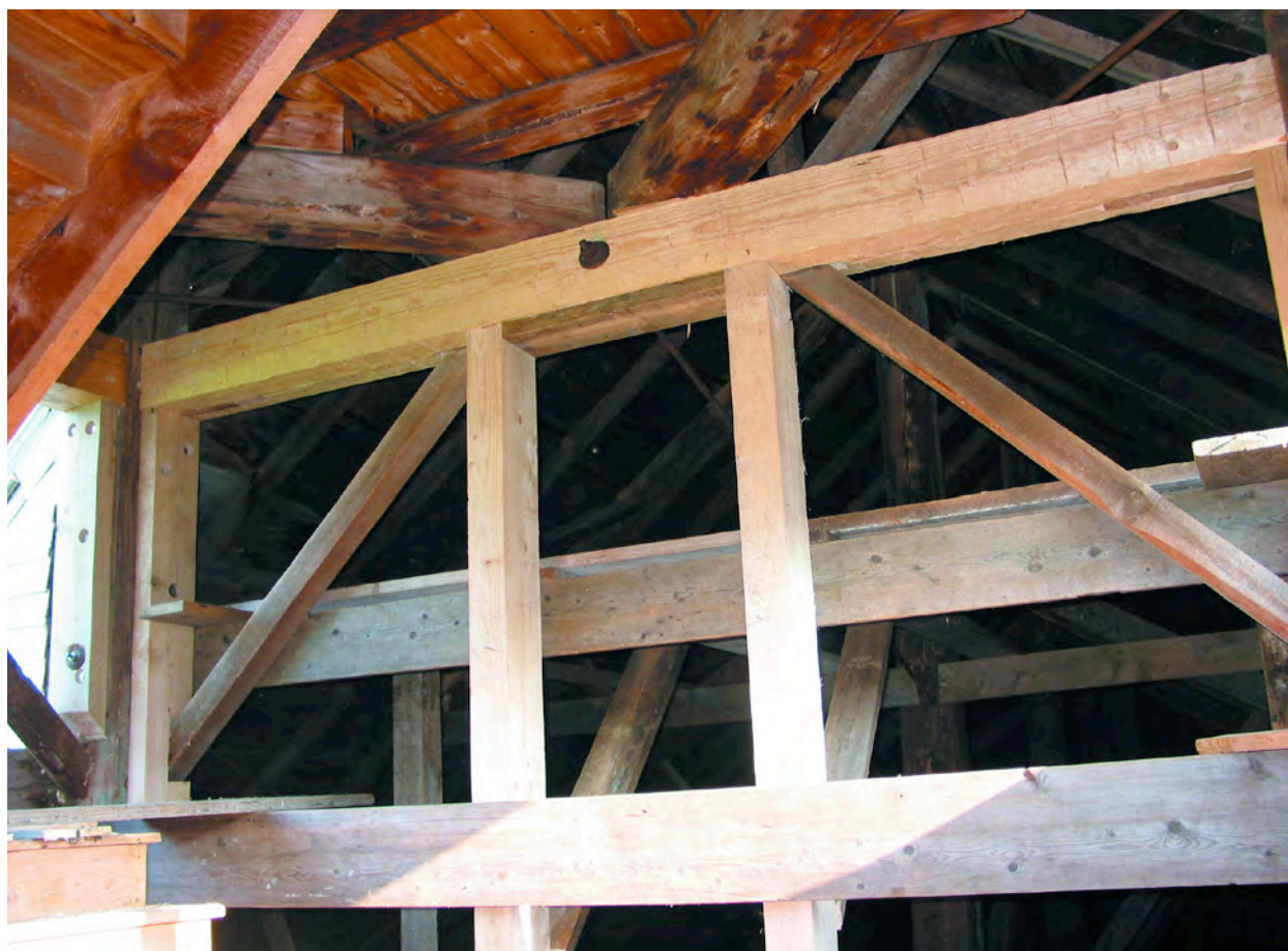
Fig. 20. New spruce tower girt supports diagonal sleepers carrying upper stages. Bolted 4x9 sisters at each end relieve 2-in. splined tenons of shear forces; long braces and median posts stiffen middle of girt against bending. At girt center, nipped iron rod (old but not original) runs back to tie beam of second interior roof truss.
