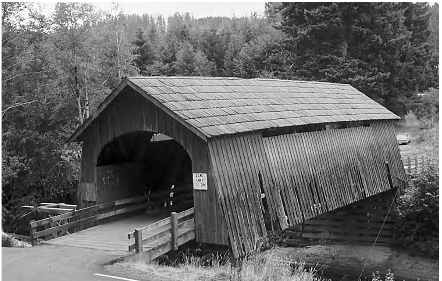
Fig. 7. Fisher School Bridge, Lincoln County, Oregon, built in 1919, with broadly flared siding.
