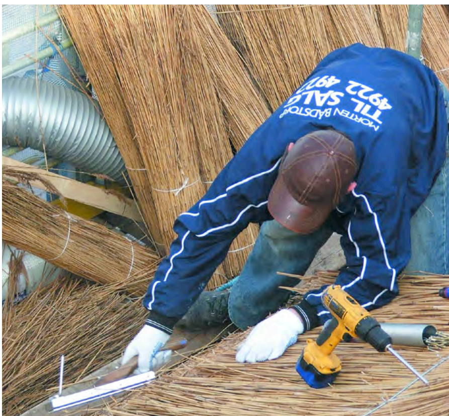
Fig. 13. Ramunas Lukasuskas uses petting board to stroke and shape bundles of thatch. Gloves protect hands from abrasive thatch. Drill drives long screws prefitted with two wires into roof batten below; thatcher then ties wires around bale. Heavy wire at lower right holds down entire course of bundles.
