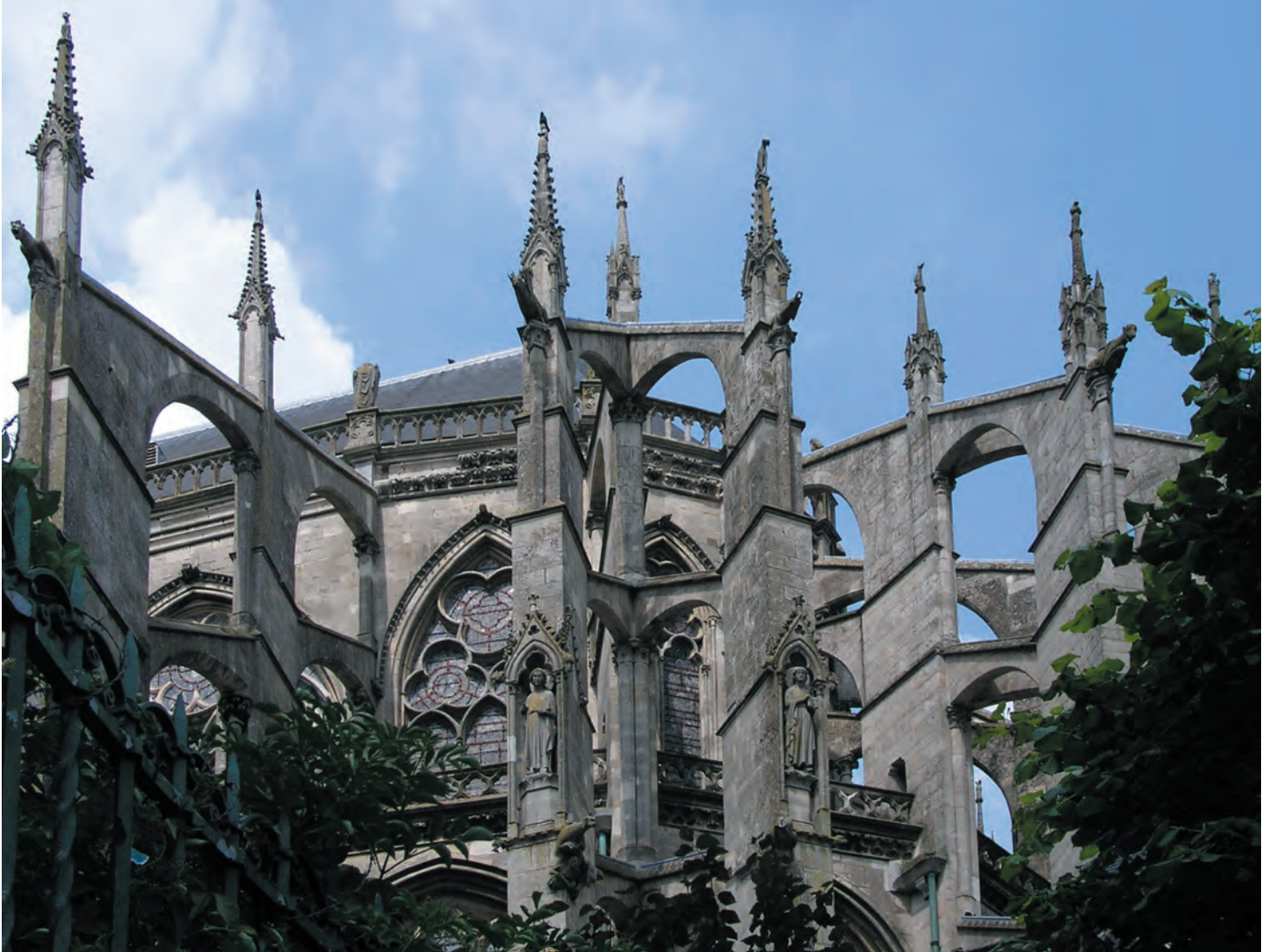
Fig. 1. Cathédrale Saint-Julien, Le Mans, with unique split buttresses configured to flank windows in first-story choir below.
