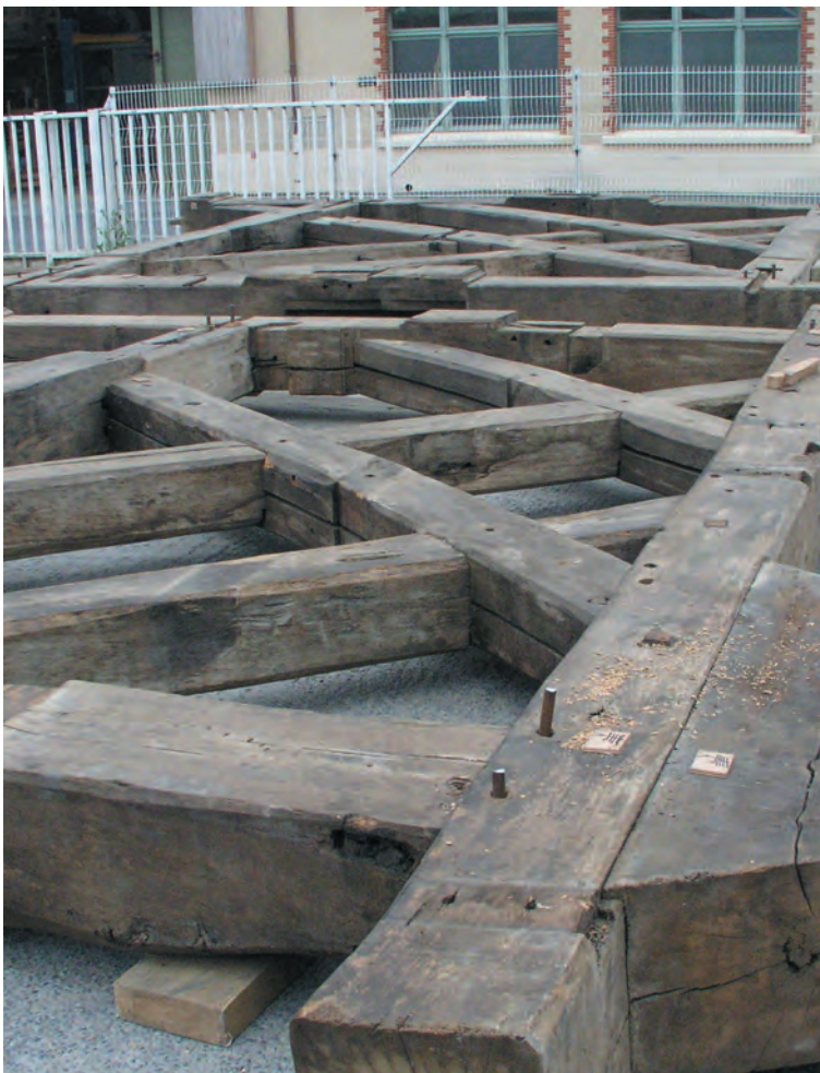
Fig. 5. Perrault sawyers prepare large bandsaw blades in immaculate sawmill. Log on carriage will yield a timber about 30 in. square. Figs. 6–8. Below, below left and above left, sophisticated 18th-century timber work from the north tower of the Église Saint-Sulpice in Paris, under repair at Ateliers Perrault near Angers.
