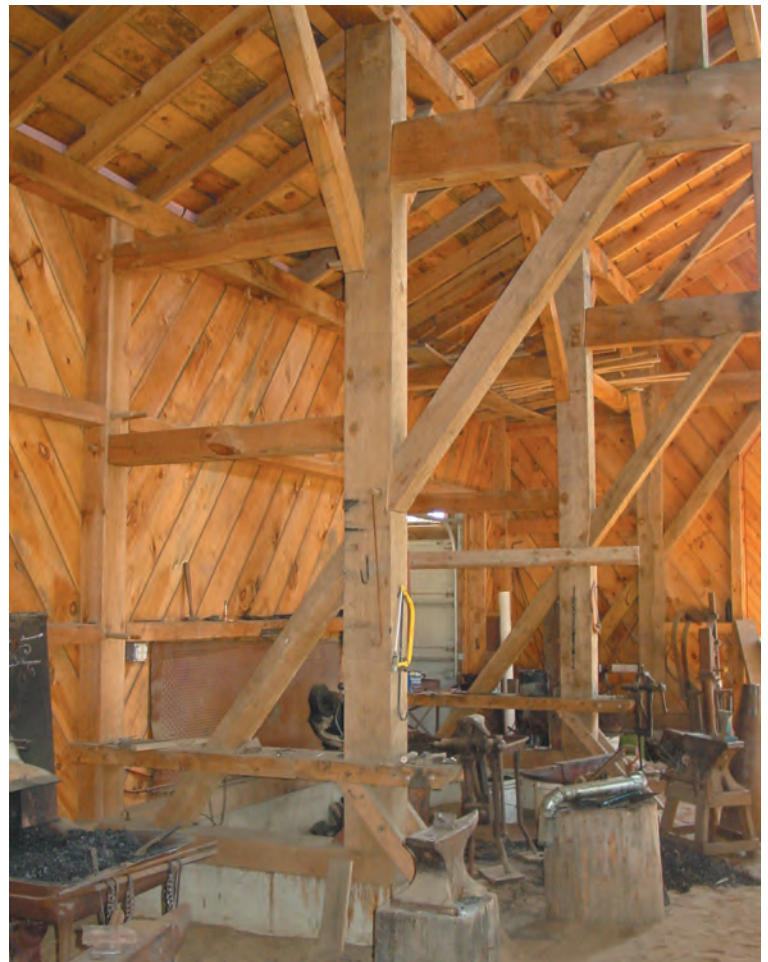
Fig. 1. The Herb Nehring Blacksmith Shop at Tillers International, Kalamazoo, Michigan, incorporated large diagonal braces, tension joinery, diagonally sheathed shearwalls and a flexible roof diaphragm to achieve adequate racking resistance for code wind loads. Design by Dick Roosenberg, Tom Nehil, Amy Warren.
