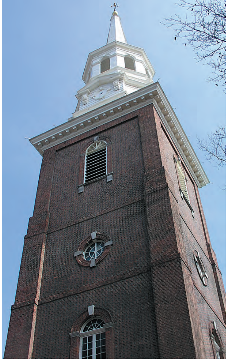
Fig. 5. Christ Church, Philadelphia, 1754. Tower stands free of church body, supports two wooden stages and a spire framed platform style.
