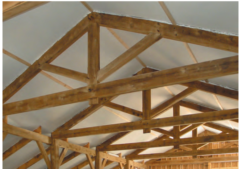
Fig. 17. Typical modern kingpost truss with diagonal web members to support rafters. White oak 6x12 rafters and tie beams span 30 ft.
