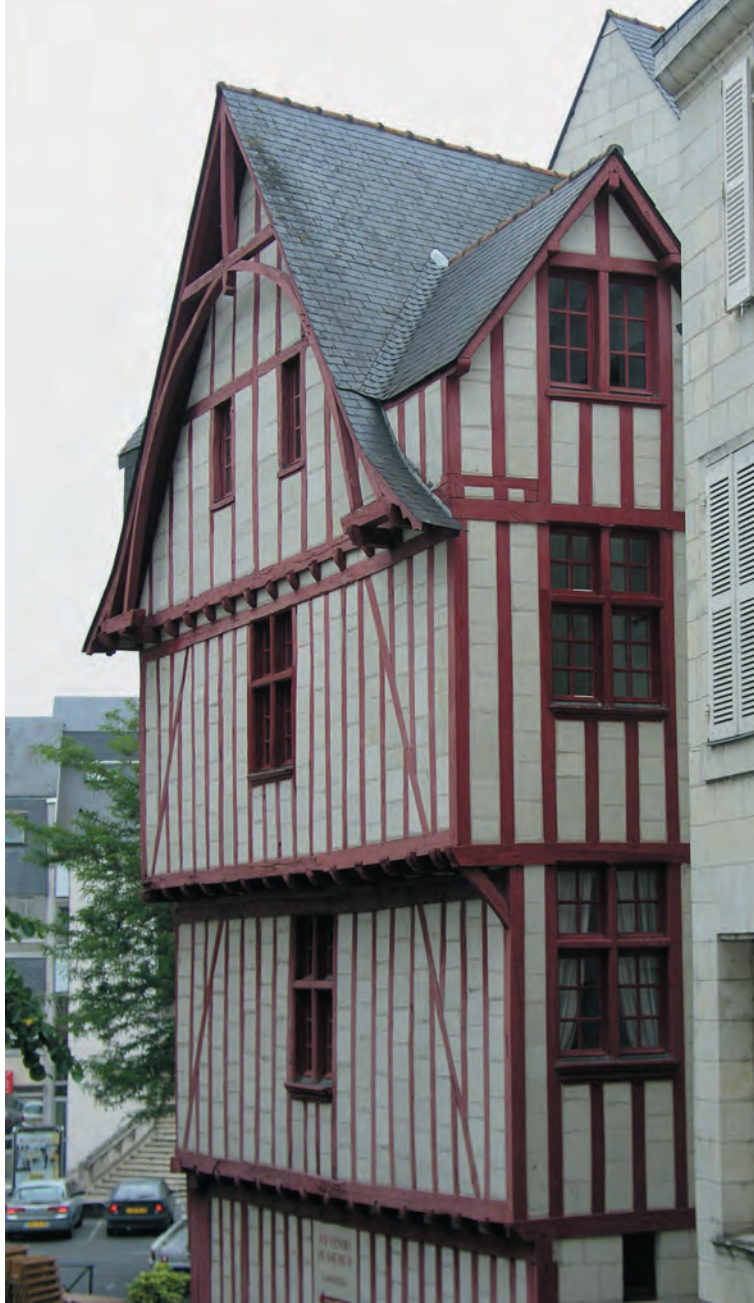
Fig. 11. Tufa (soft limestone) infilled timber frame in Saumur.
