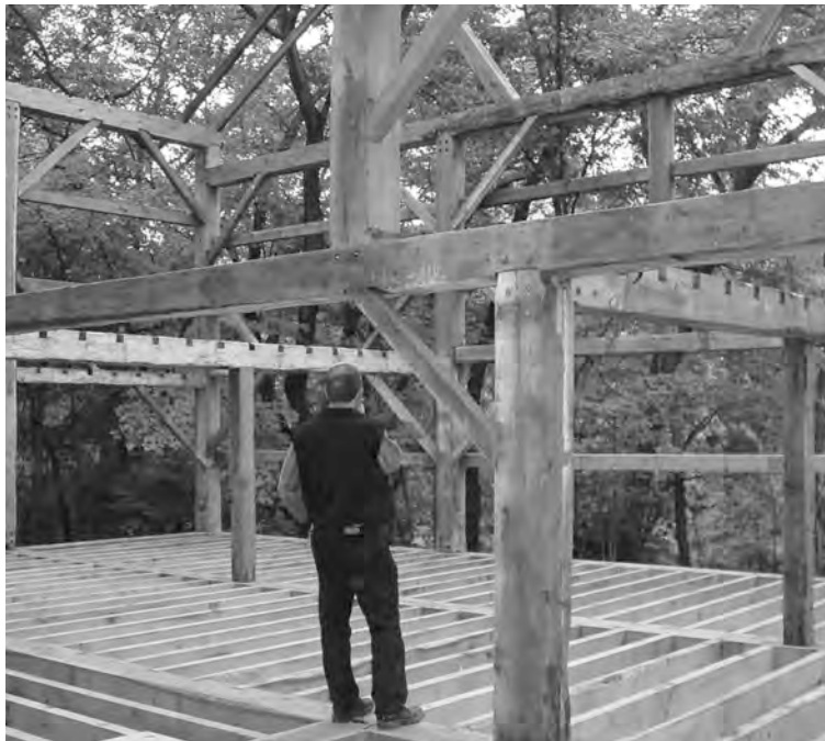
Fig. 6. Knee braces can effectively widen a support and stiffen beams, helping to transfer loads to posts.
