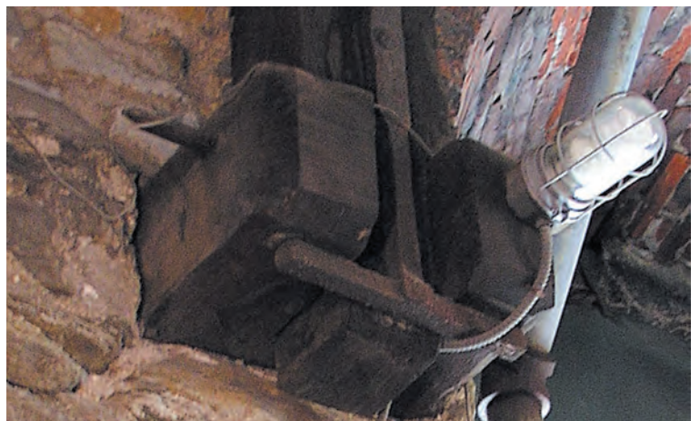
Fig. 6. At Christ Church, forged iron bar and wood corbel buried in stone rubble anchor first wooden stage above to masonry tower.
