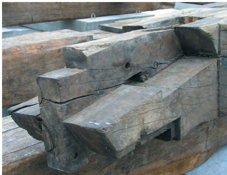
Fig. 5. Perrault sawyers prepare large bandsaw blades in immaculate sawmill. Log on carriage will yield a timber about 30 in. square. Figs. 6–8. Below, below left and above left, sophisticated 18th-century timber work from the north tower of the Église Saint-Sulpice in Paris, under repair at Ateliers Perrault near Angers.
