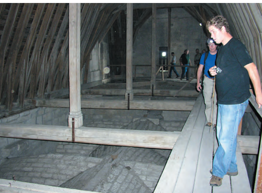
Fig. 18. Inside kingposted roof of Saint-Gatien.
