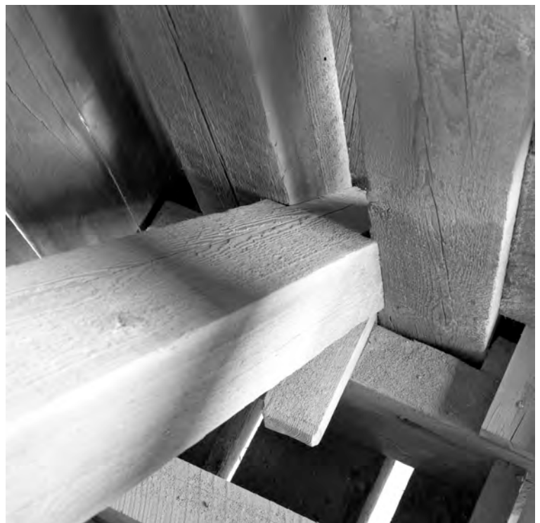
Fig. 4. Counterbrace wedge at the bottom instead of the top. Blair Bridge, Campton, New Hampshire, built 1869.
