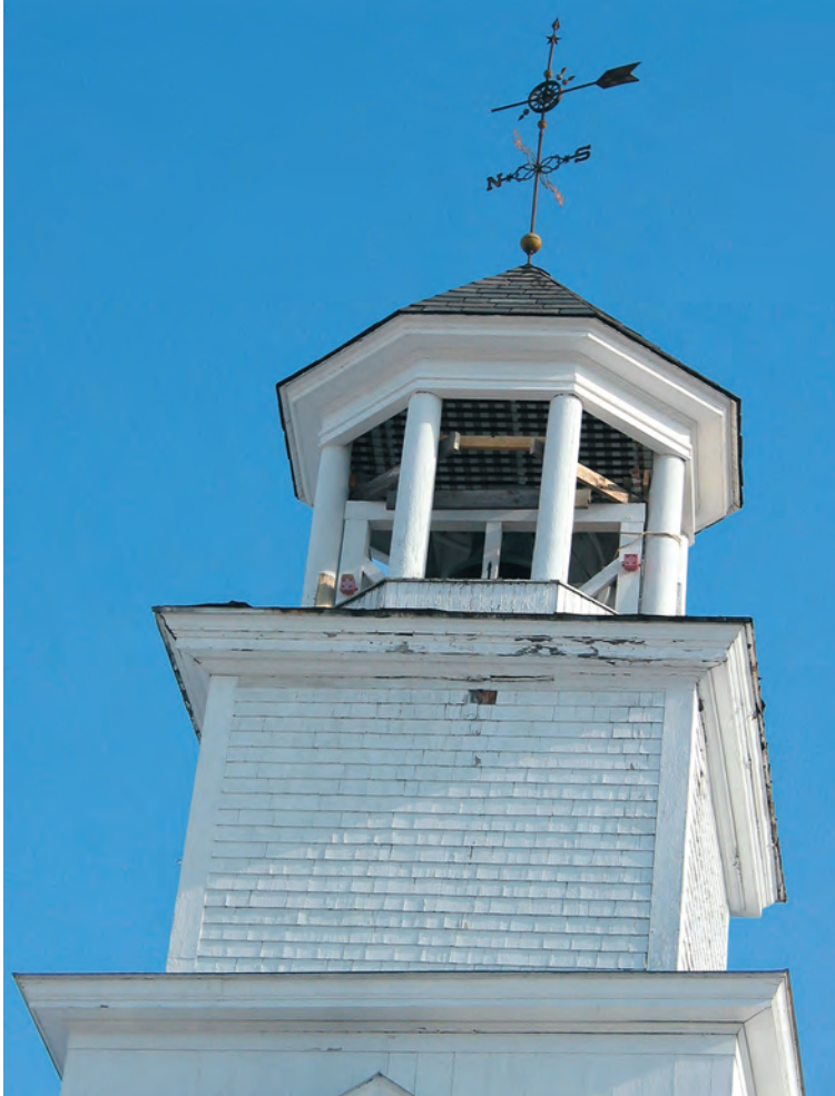
Fig. 6. Decay in posts and supporting beams led to significant distortion of steeple at the South Woodstock, Vt., Community Church, 1836.
