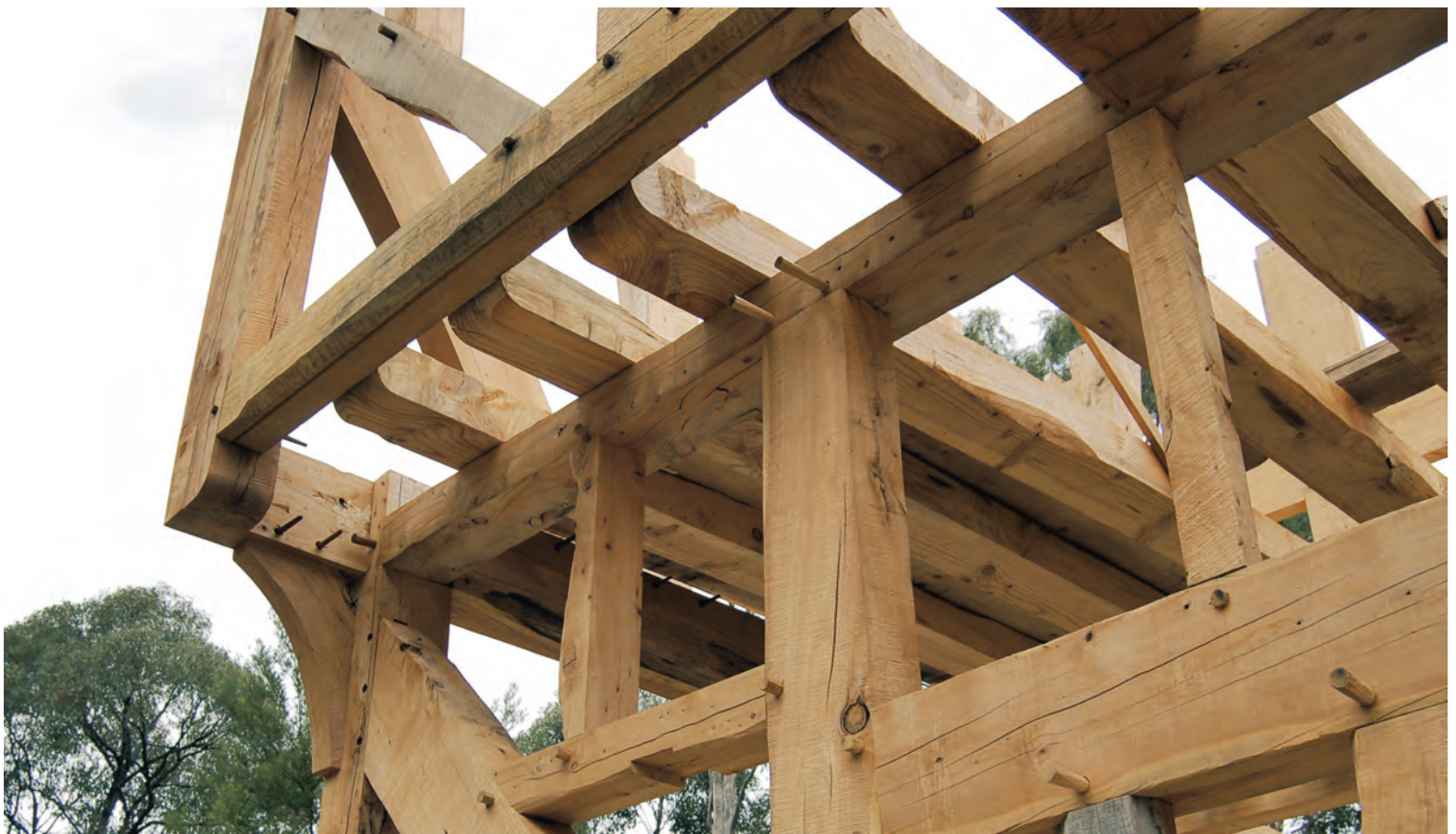
Fig. 7. Jetty bressummer rabbet shelters ends of 7x5 pine floor joists. Note distinct drip groove in underside. Tenons of wall girts support end posts.
