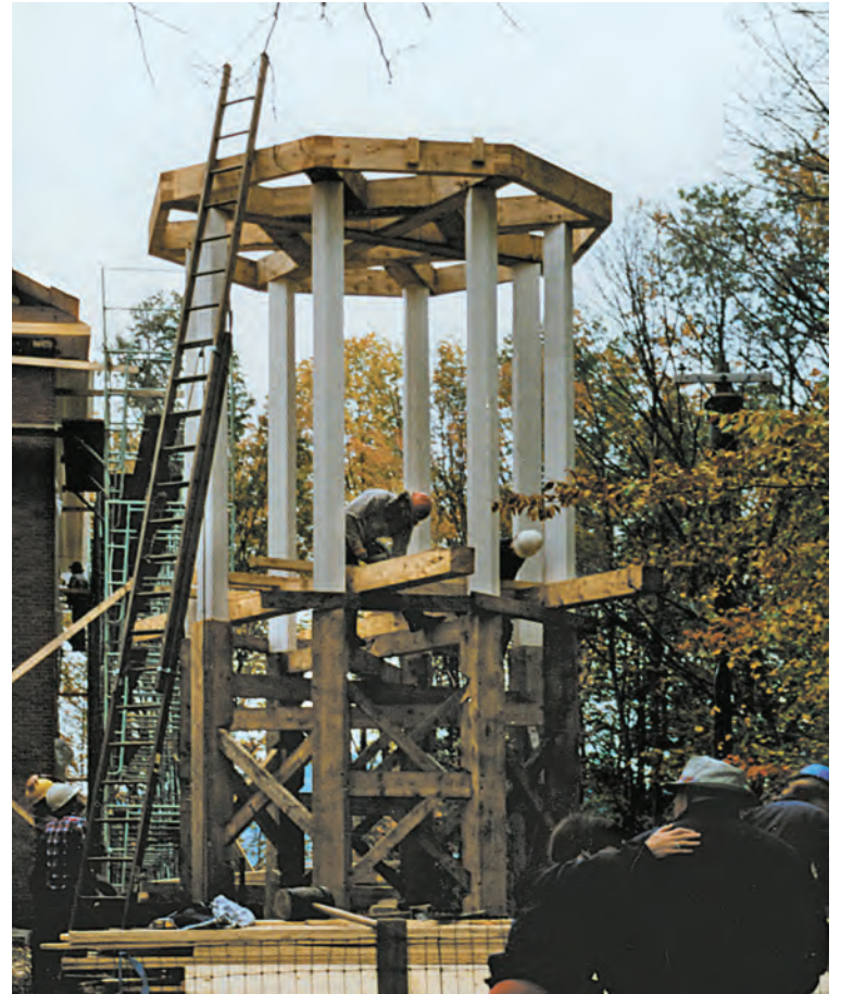
Fig. 24. Belfry frame with major crab installed on top to carry lantern. Workers rig heavy lifting timbers that will bear under the crab to transport the assembly to the meetinghouse.
