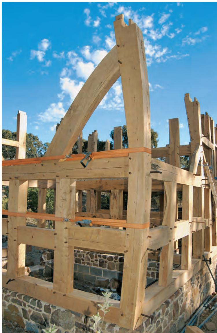
Fig. 3. Not a fisheye view. Swept corner post posed interesting problems.
