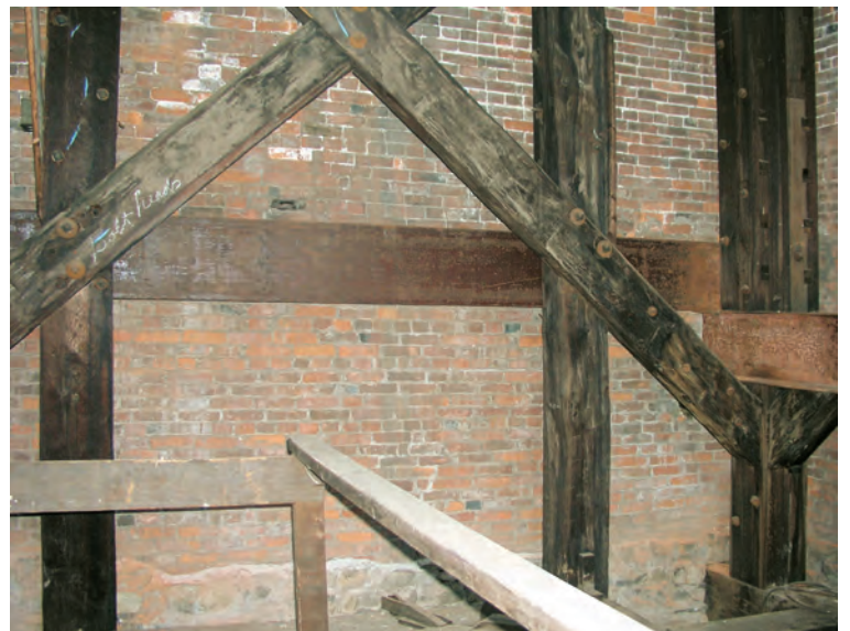
Figs. 7–8. Center Church, New Haven, Conn., 1811. Deep penetration of stages to those below successfully resists effects of wind. Below, lowest wood-framed stage is deeply lodged in brick tower.
