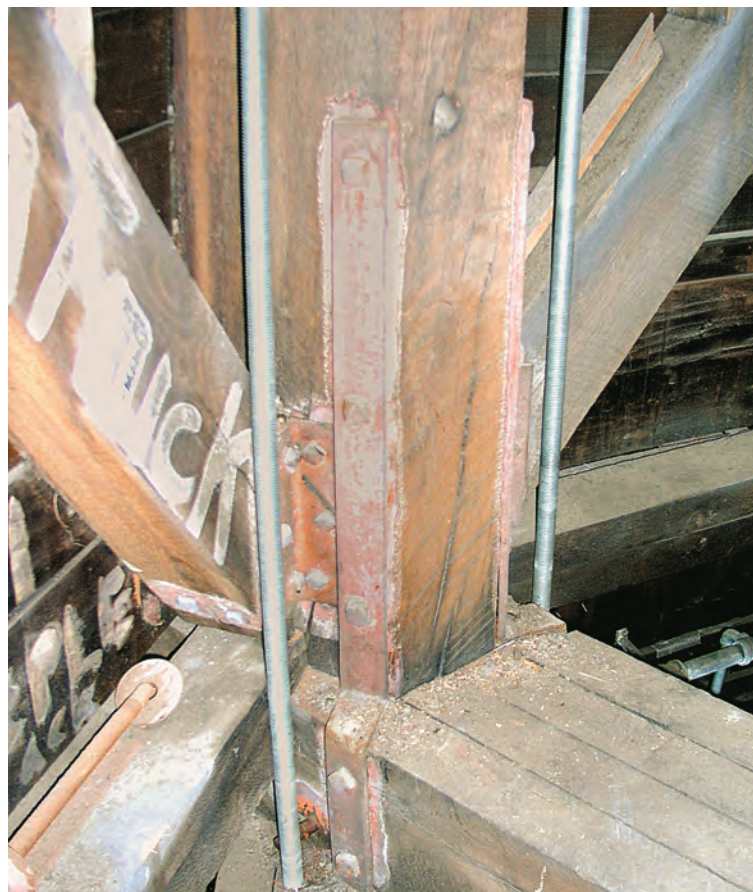
Fig. 5. Laminated beams replaced rotted material at Christ Church in 1771. Iron straps appear to be original, rods 20th-century.
