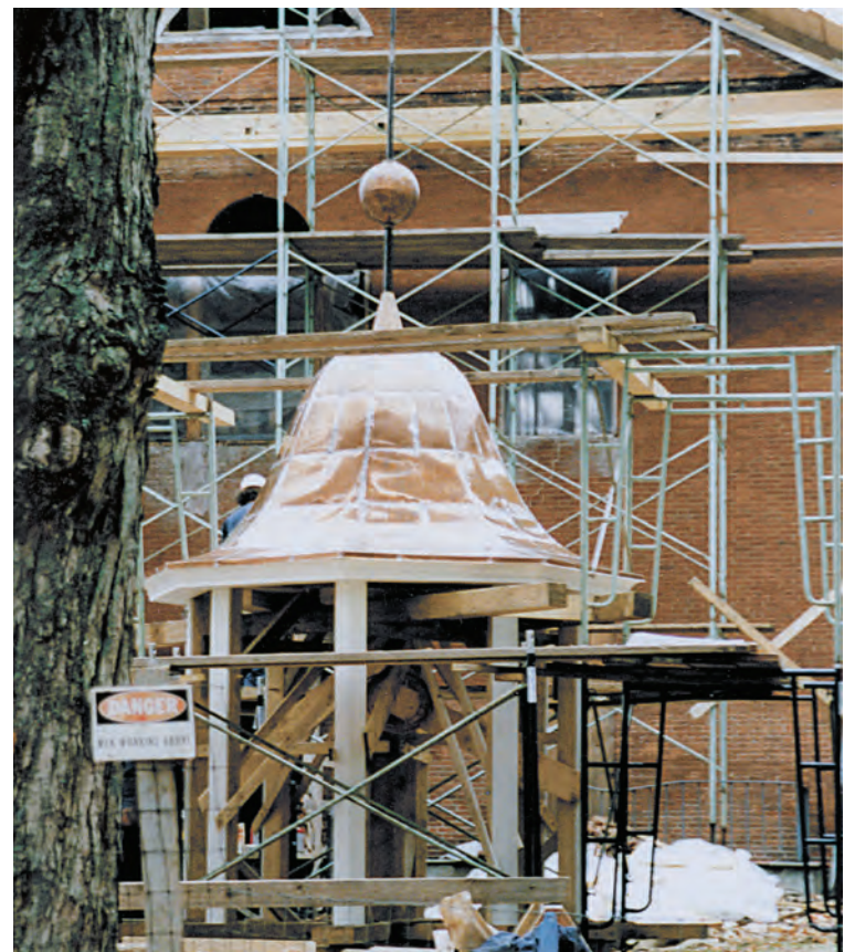
Fig. 25. Lantern covered by soldered copper cupola roof, topped by mast with orb (weathervane unseen above), awaits lift to top of belfry. Timbers just under cornice will be strapped to lift the stage.
