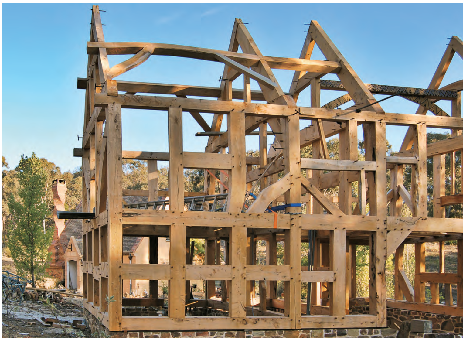
Fig. 9. Main frame complete, with straps and chain for troublesome crossframe three post left in place. Purlins lock to each other or to a rafter; wind braces are taper-lapped to rafters and purlins. House in background with twisted chimney dates from 2000.
