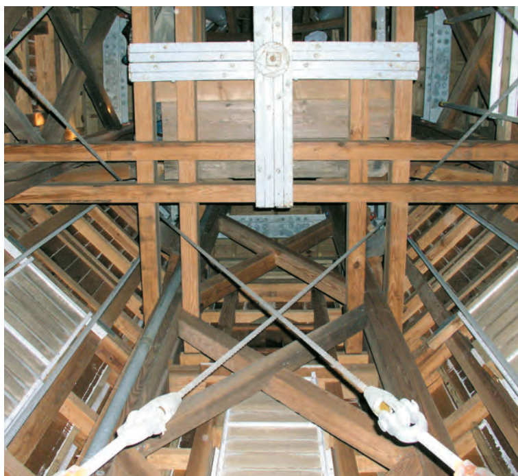
Fig. 3. Restored middle-stage framing (octagonal stage, Fig. 2) of steeple at Salem. Tall spire above is tied down via long central bolt terminating at laminated crossing that bears up against partners in middle stage.
