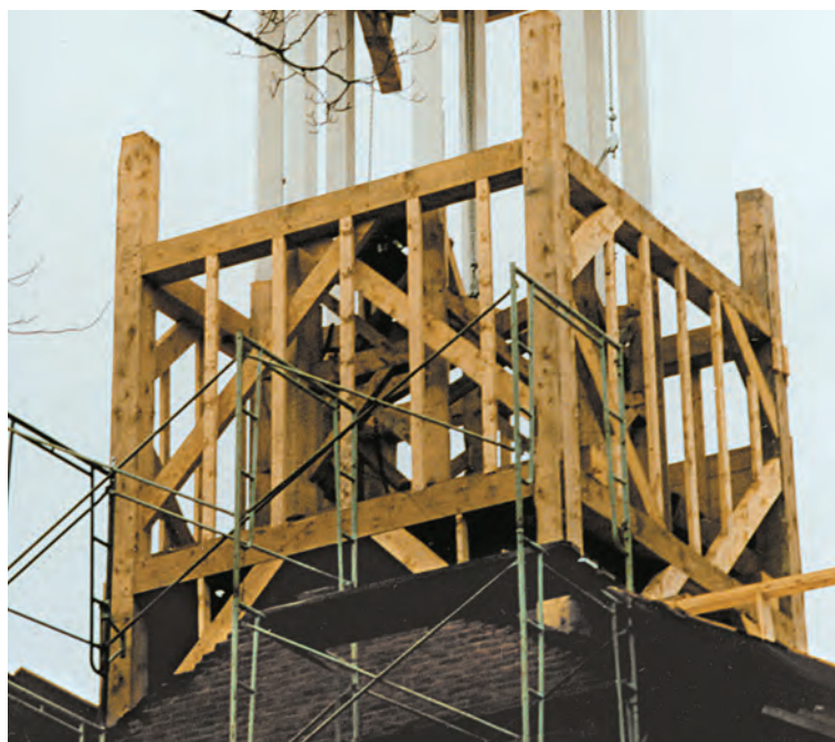
Fig. 21. Weathersfield tower frame in place, well braced and studded for exterior finish. Posts descend to long sleepers in attic and carry short sleepers halfway up to foot belfry posts. See also Fig. 17.
