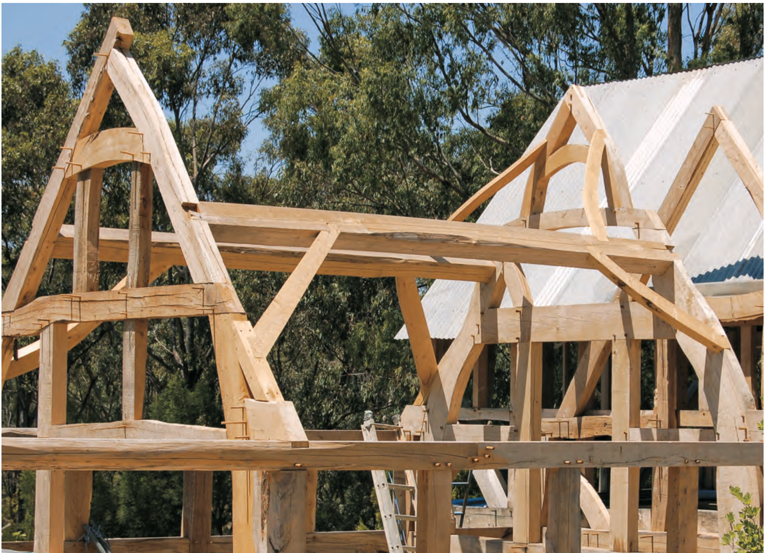
Fig. 10. Framing of the ell continues. Note two tiered-cruck, spur acting as truncated tie, short bridled scarf in plate (three pegs) and lap-jointed wind braces. Additional crucks will rise to the left. The whole will be cob-walled and lime-plastered.
