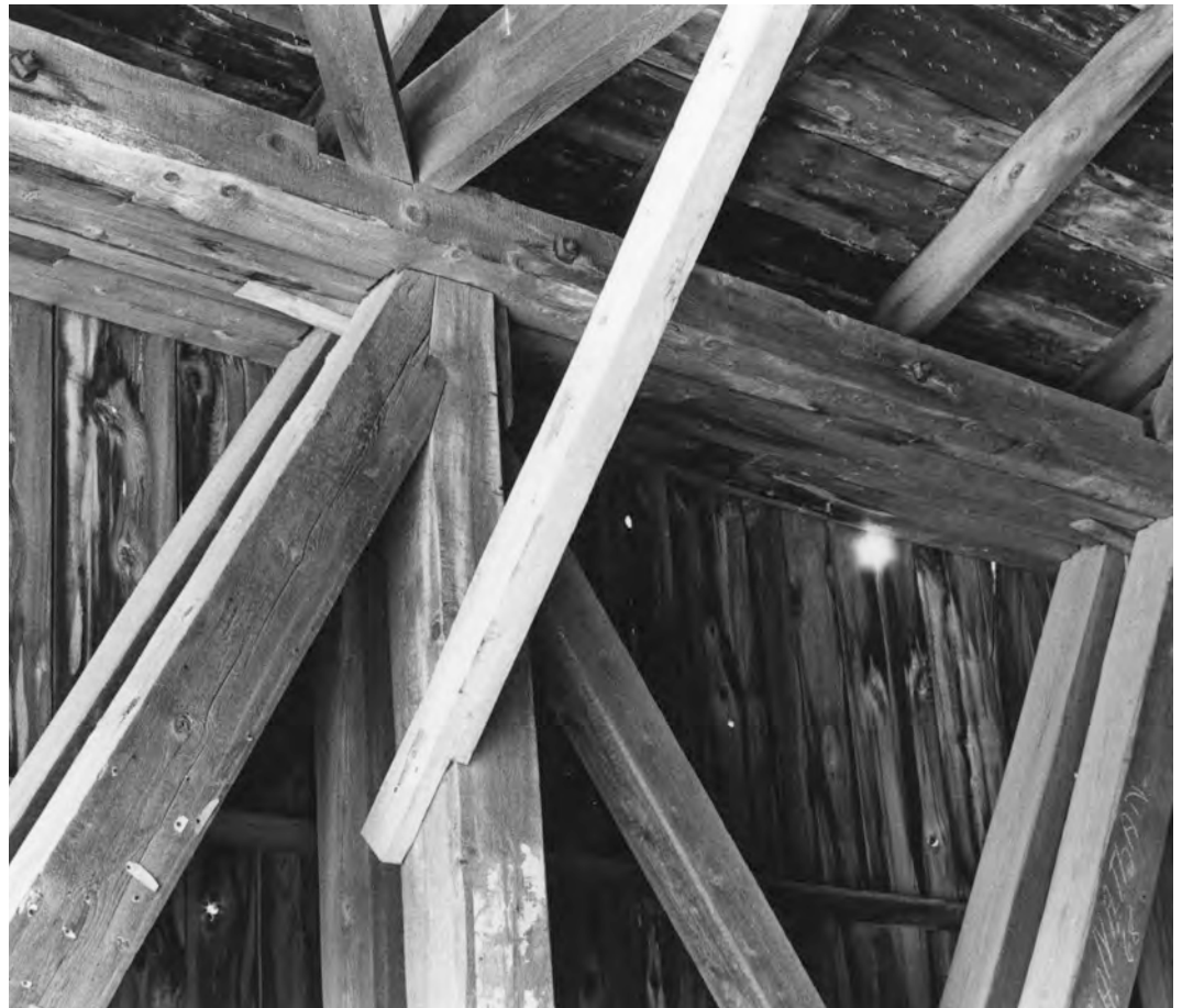
Fig. 3. Framing details of Long truss. Thin ends of counterbrace prestress wedges poke out between braces. Behind the near post an additional wedge can be seen intended to snug up the housed joint, a detail often omitted. Low's Bridge shown, between Guilford and Sangerville, Maine, built in 1857 by Leonard Knowlton and destroyed by flood in 1987, when it was the extant Long truss most closely resembling the patent (though the colonel would have recommended more post-top relish). Jan Lewandoski built a new Long truss bridge here in 1990.
