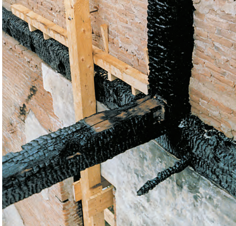
Fig. 20. Charred remains of inset plate, front tower post and long sleeper to carry steeple. New material is part of front-wall shoring.
