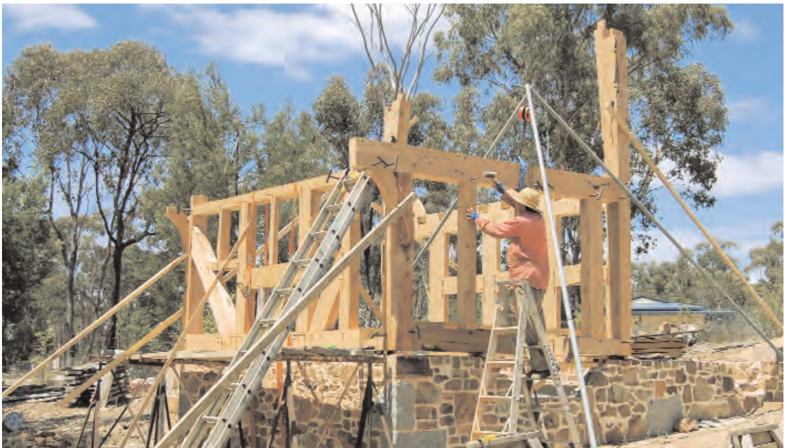
Fig. 6. Author pegs off first wall girt, which passes corner post to form end support for jetty. Pipe tripod with block and chain raised the beam.
