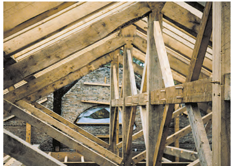
Figs. 18–19. Weathersfield truss fly-in was complicated by making up the closed mortise and tenon joinery of many connecting members.
