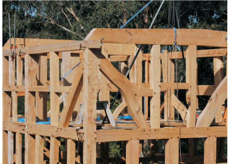
Fig. 8. Shear legs tied off to wall, last tie beam raised over top plates.
