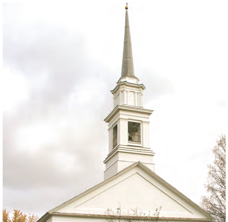
Fig. 11. Steeple at Castleton, Vt., Federated Church, 1832, showing thickened belfry corners to conceal telescoped posts from above.
