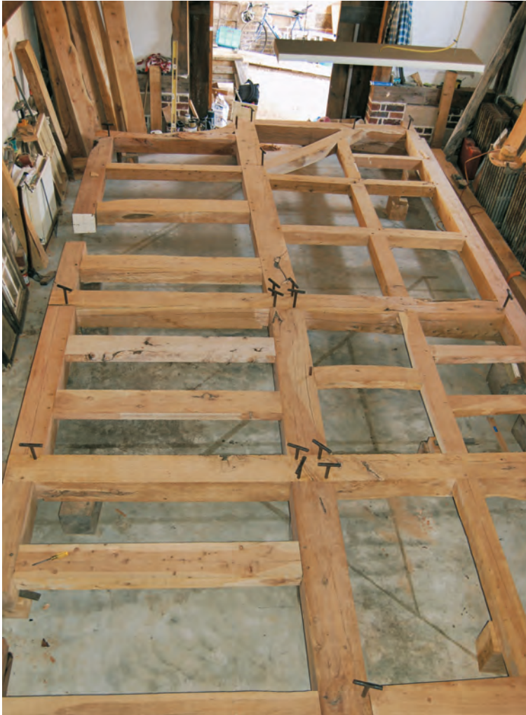
Fig. 5. West wall frame completed on floor of barn, little room to spare.
