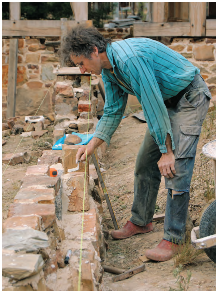
Fig. 2. Author built lime-mortared stone foundation quickly with stone gathered from property.
