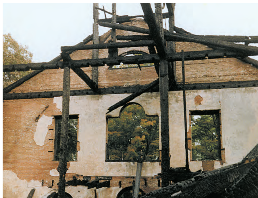
Fig. 16. Weathersfield standing timber remains included three tower posts, inset front plate, sleepers, first truss tie beam and vestibule posts.
