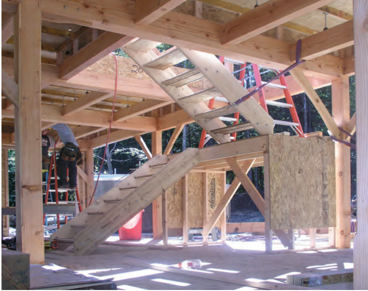
Fig. 2. Solid temporary stair is far safer than ladders.
