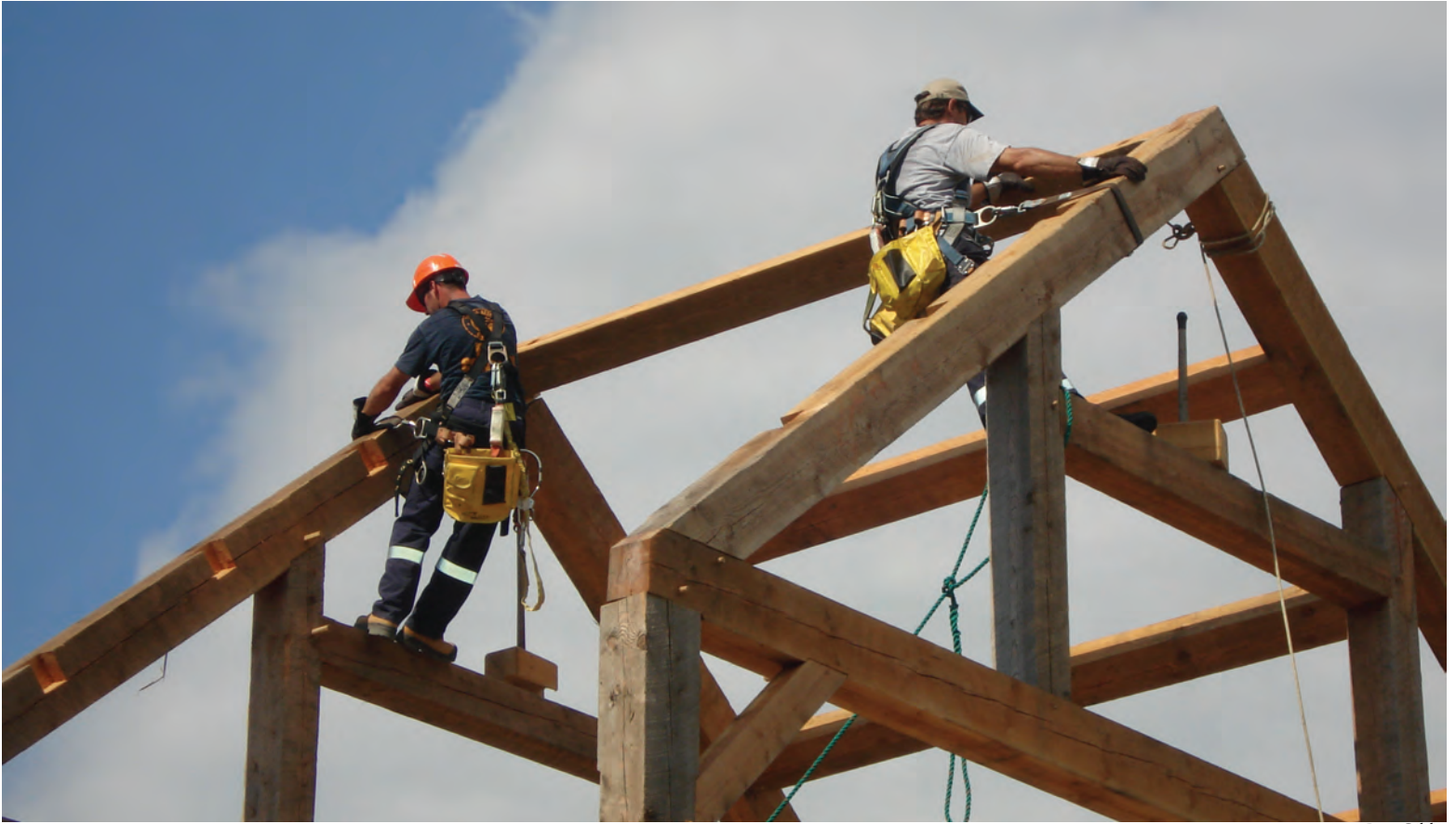
Fig. 1. Framers setting common purlins and using work-positioning restraints (fall limited to 2 ft.). Shock-absorbing fall-arrest devices worn on the back will be secured when detaching positioning devices to get around obstacles such as post on left. Commanders sitting unsecured on beams may have been deemed impractical to attach via lanyard to framer or frame, as are smaller tools routinely. Controlled-access zone beneath.
