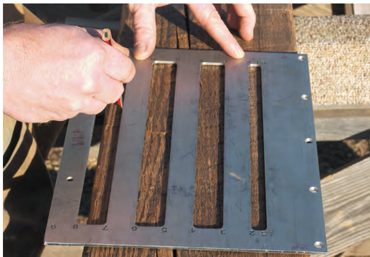
Fig. 12. Marking reduction at rafter foot using a Borneman template.
