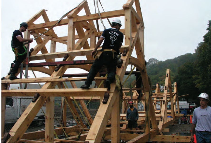
Fig. 4. Assemble as much as possible on the ground.
