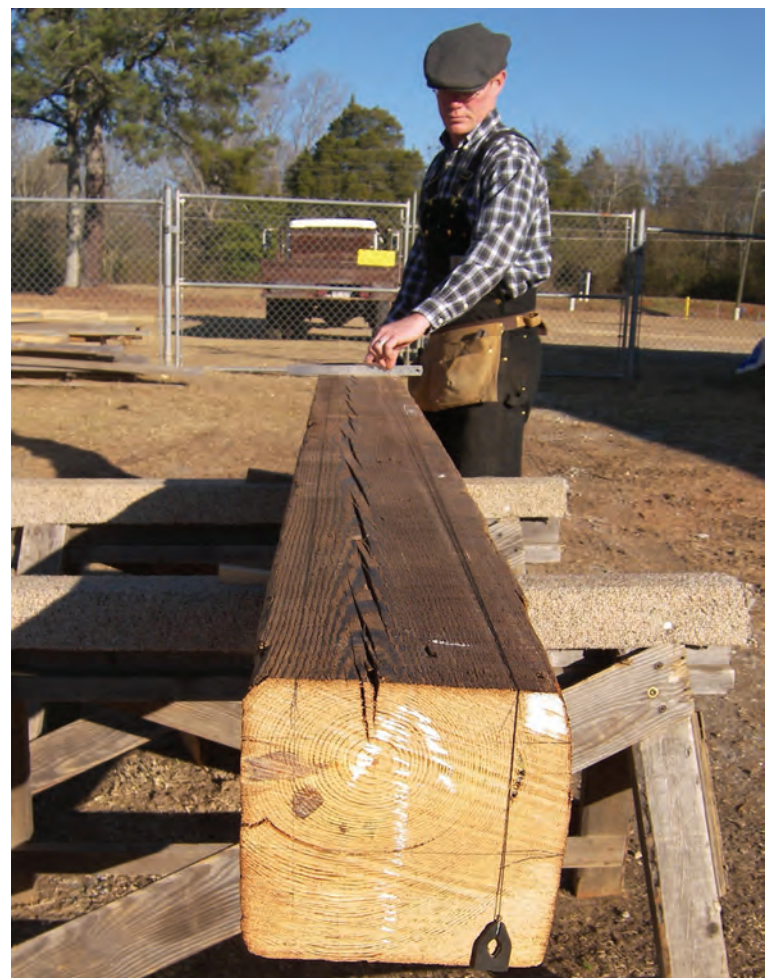
Fig. 8. A straightedge set under a taut chalkline can be rolled on edge, allowing fingers to grasp the fine line easily.
