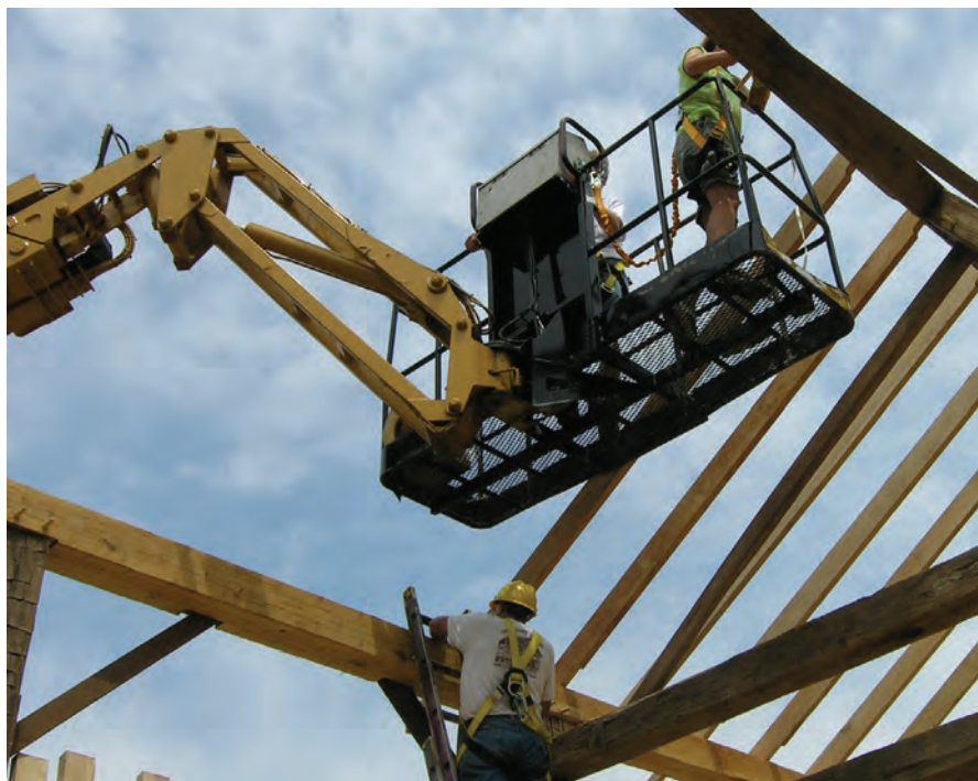
Fig. 6. Mobile elevated work platforms offer ideal positioning and leave no structure behind.
