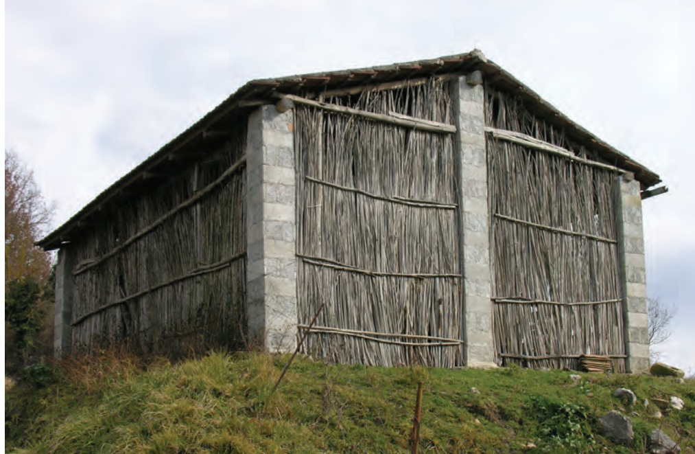
Small modern barn nearby replaces wood posts with concrete block posts but retains fratticco rush infill. Plaster omitted in favor of ventilation for hay inside.
