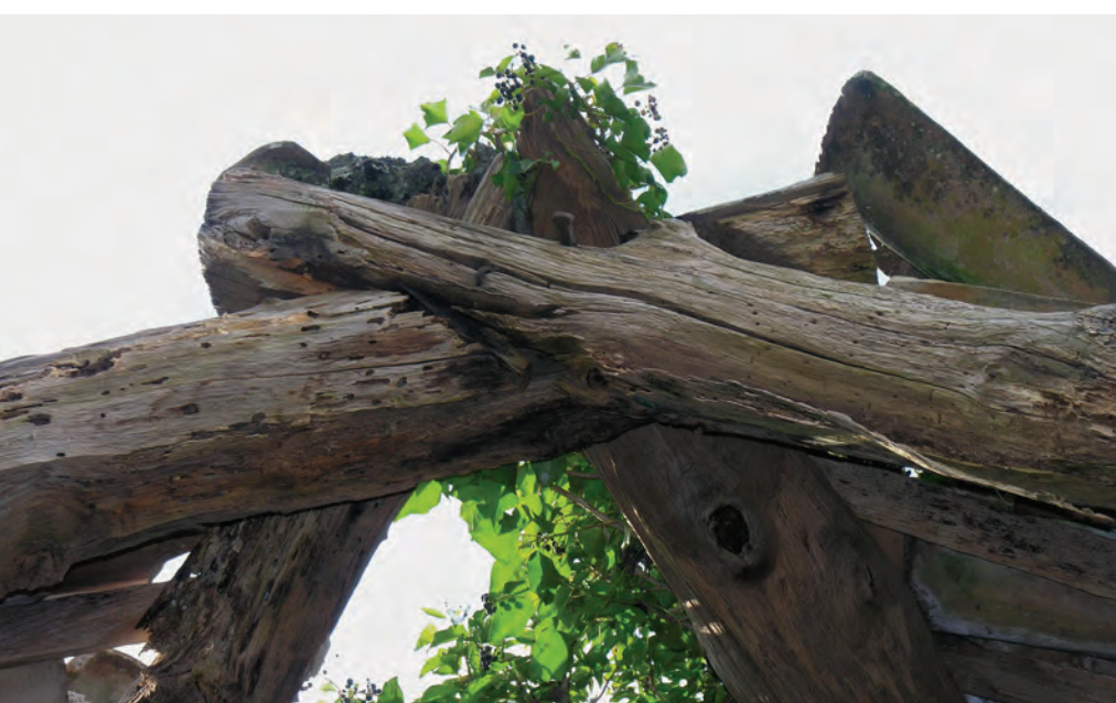
Remains of the cabin near an abandoned rural stone house built around the beginning of the 19th century. Typical fratticco post joint clasps plate in natural crook. Lapped rafter peak clasps ridge.
