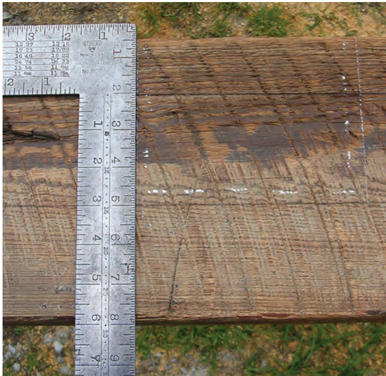
Fig. 9. Marking sides of a purlin housing by squaring down to the 4½-in. line. Square is registered on the 1½-in. line.
