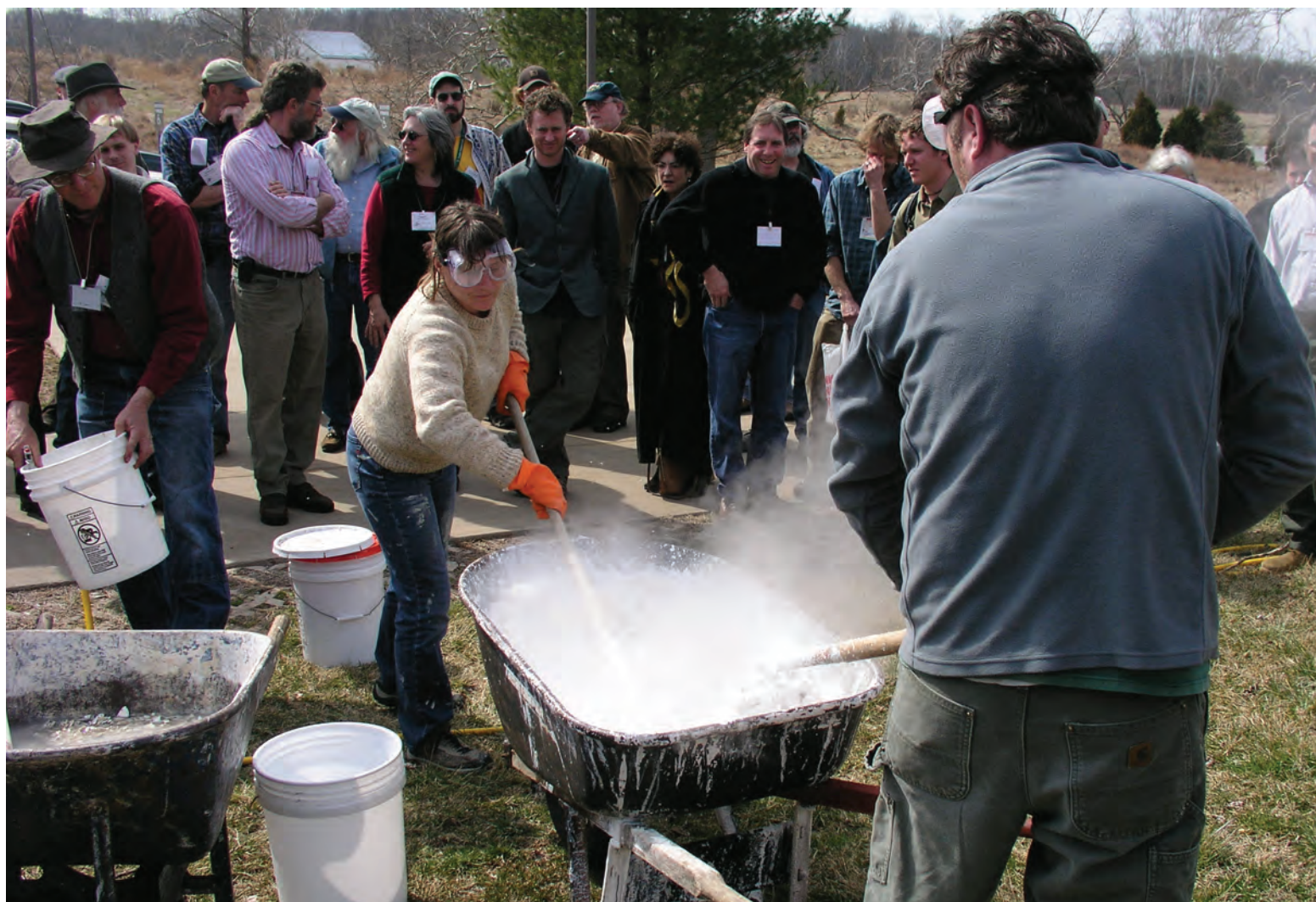
Slaking lime at TTRAG '08, heat of reaction dramatically vaporizing excess water. Left to right: Michael Burrey, Penelope Austin, Sean Mears.
