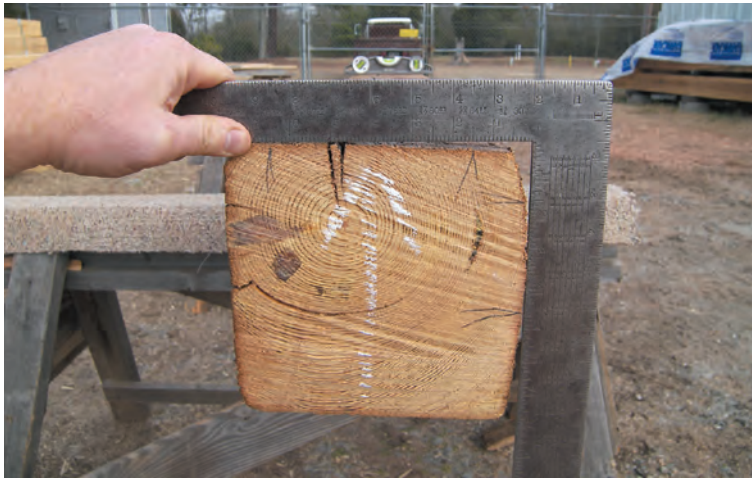
Fig. 6. Marking line locations on endgrain. A knifed notch at the arrows will later keep the stretched line in place.
