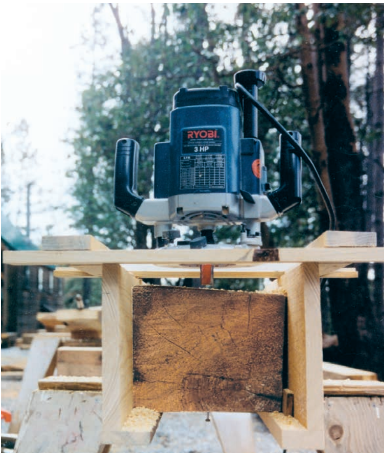
Fig. 6. Router mounted on jig ready to produce housing parallel to reference surface (underside of timber in photo).
