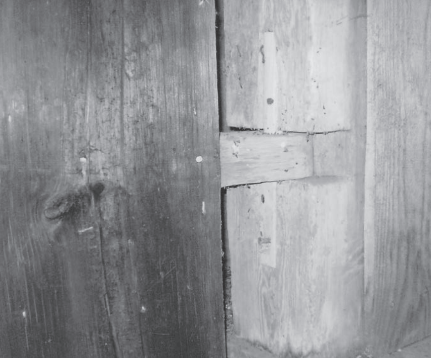
Fig. 3. Detail of oak lower door hinge, seen from outside, showing wood pintle let in and nailed to doorpost. Hinge strap measures 3x4 at the pintle. Door has been opened about 120 degrees.
