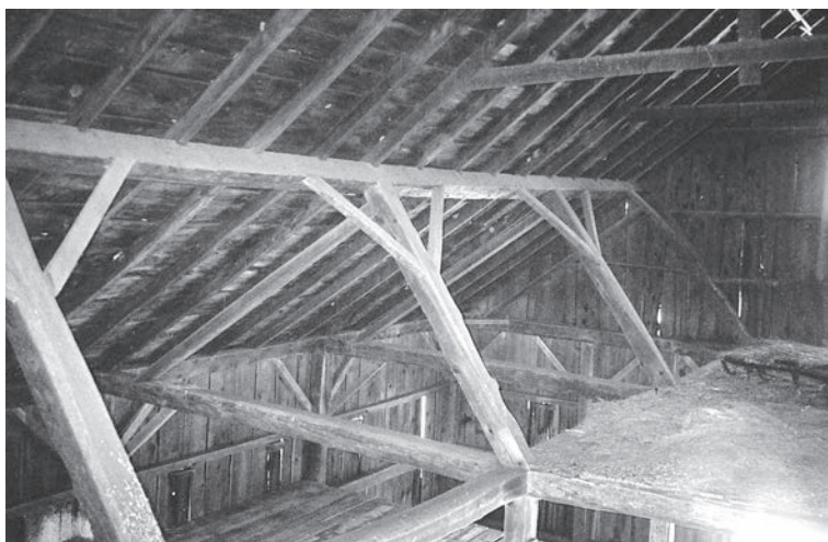
Fig. 2. Purlin on canted posts supports discontinuous rafters. Note ties at plate level.
