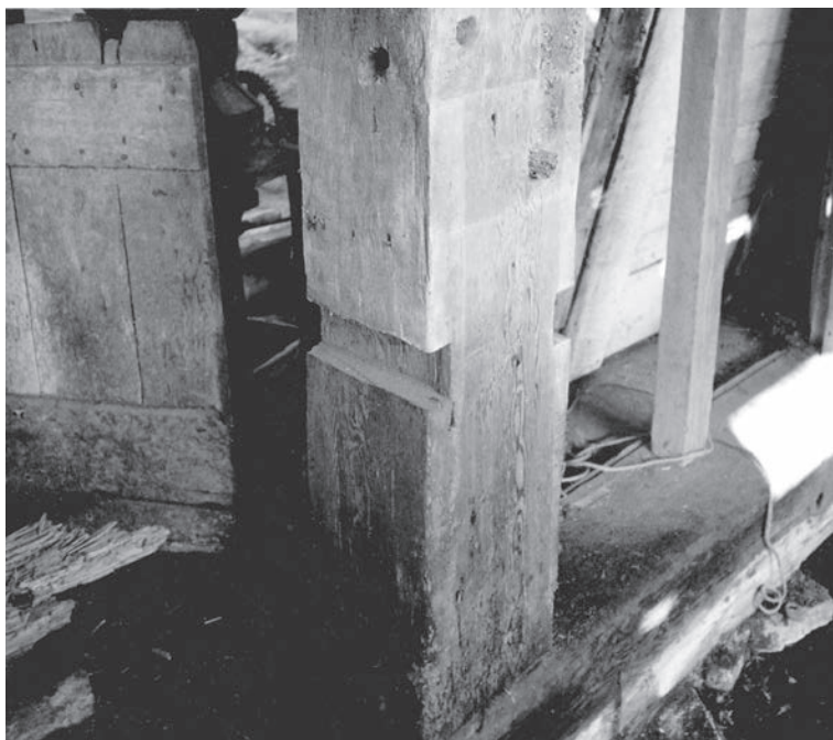
Fig. 10. Trench in H-frame post for edge of manger board to carry grain for animals. The Wemple barn had such boards at two levels.
