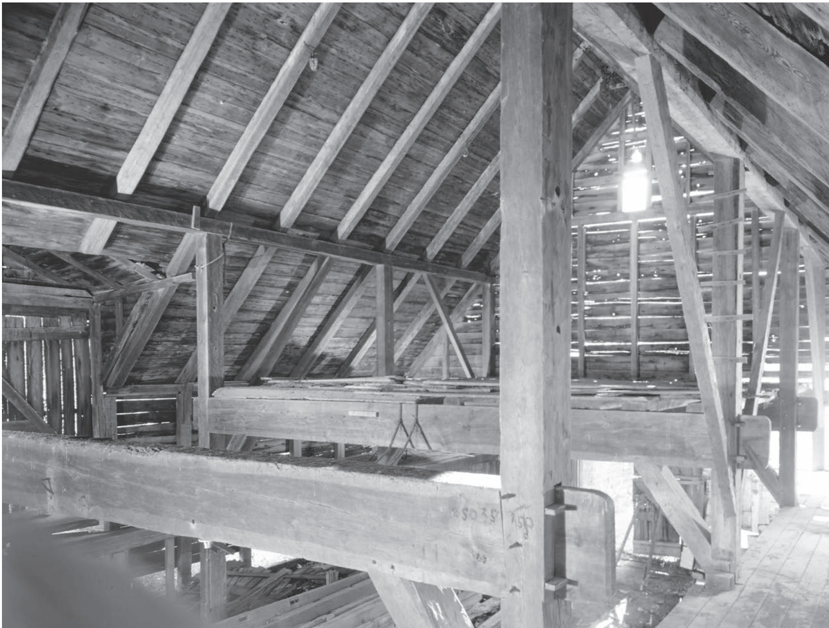
Fig. 6. Recent general view of Wemple barn interior, showing three central H-frames, long purlin braces and roof framing. Purlins run 56 ft. unscarfed, rafters 30 ft. Anchorbeams, 30 ft. tip to tip, measure about 12x22. At left, sidewall wagon entrance cut in 19th century.
