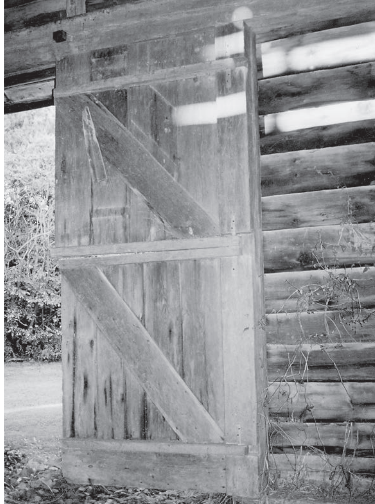
Fig. 4. Complete 12-ft. wagon door leaf in original divided condition. Battens are fastened from the inside.
