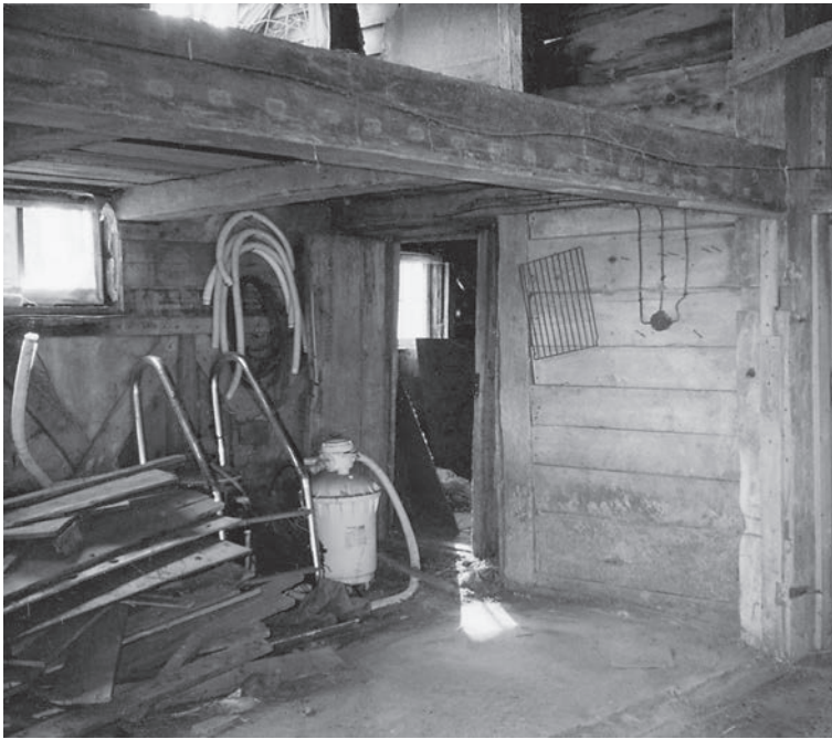
Fig. 9. Manger beam (running left to right in upper part of photo) shows ghosts of manger stakes that held feed above and ahead of the animals. The stakes ran down at an angle a short distance into the central aisle, terminating in a rail above the floor. H-frame post at right.
