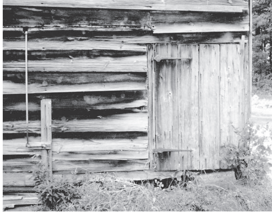
Fig 5. Animal doors on wrought hinges served horses and cows at respective corners of one gable end.
