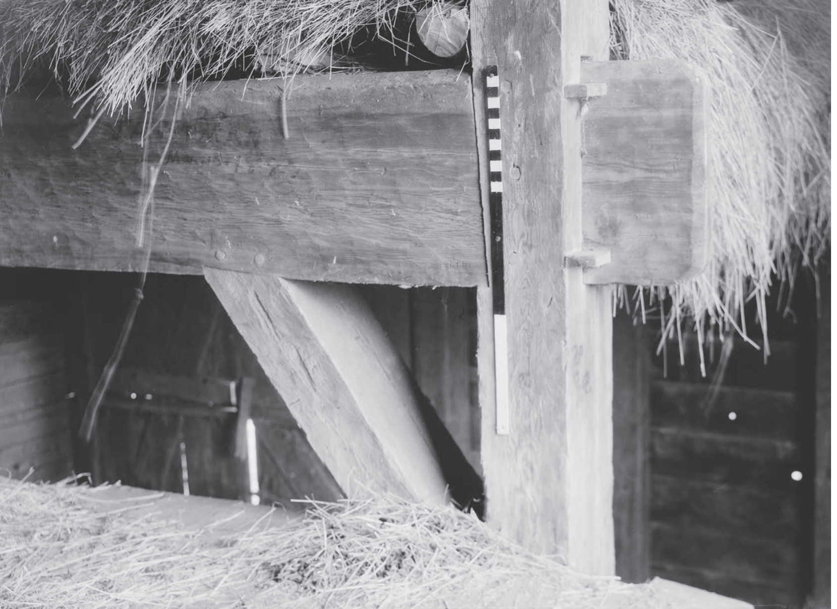
Fig. 7. Diminished shoulder anchorbeam, extended tenon with outside wedges and partial view of H-frame endpost and diminished shoulder kneebrace, all pitch pine except for the oak wedges. Three 1-in. pins secure the connection as well. Hewing and joinery are exemplary. The scale is 3 ft. long, partially subdivided into inches. Historic American Buildings Survey photograph by Nelson E. Baldwin, after 1933.
