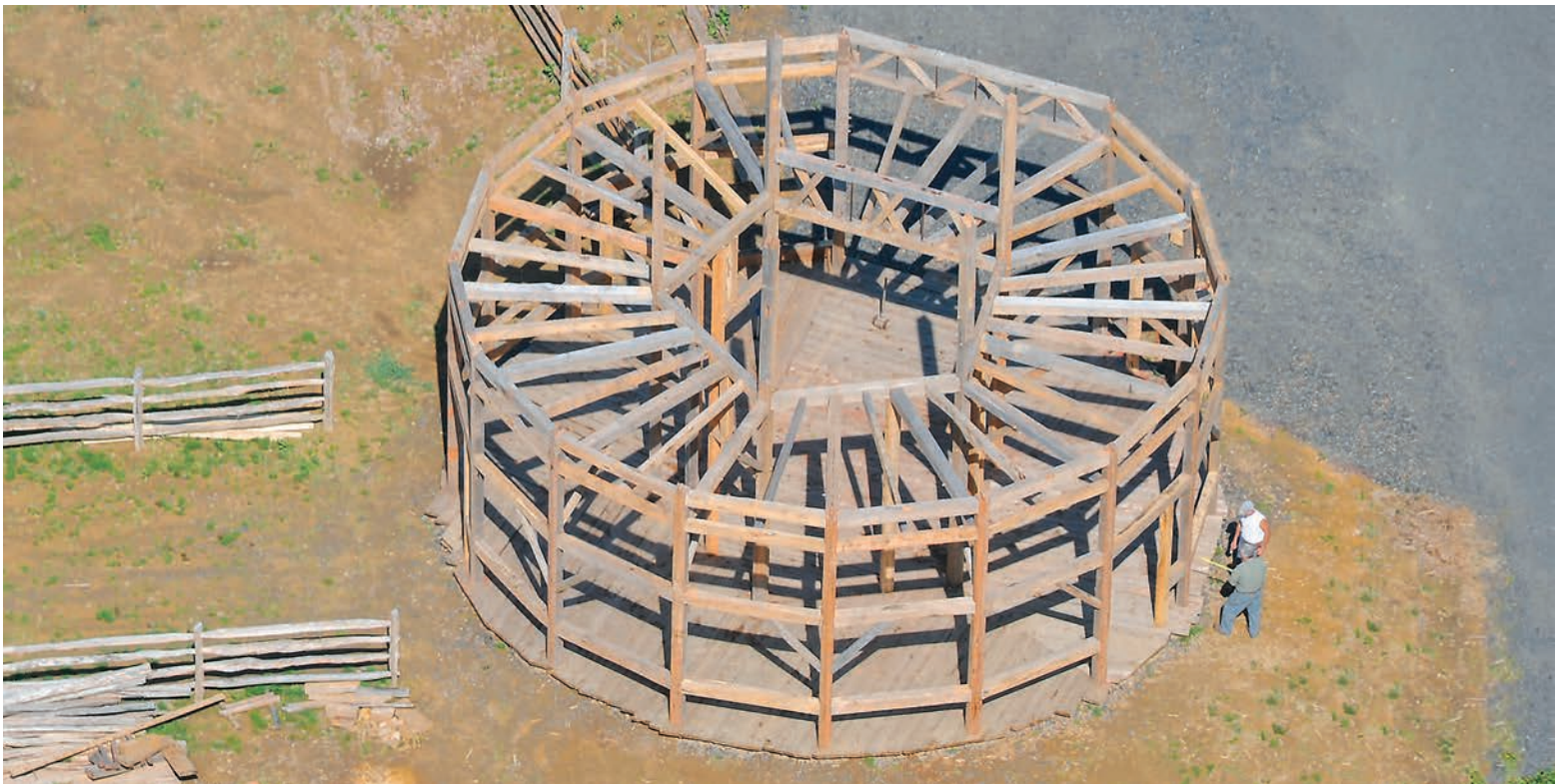
Fig. 11. Barn takes shape with addition of perimeter elements. Central opening, entrance bay, joists and ties plainly visible from above.
