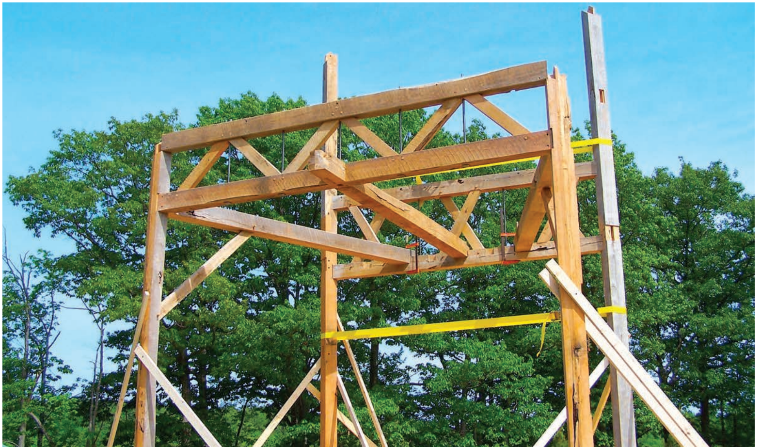
Fig. 9. Second raising assembly added truss over doorway and joists to make up main entrance bay.
