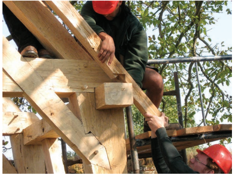
Above, Laurie Smith describing the compass-obtained layout for the brace end and the peg hole. Above right, the layout executed on a passing brace. Below, daisy wheel layout yields proportions of garden shelter. Below right, the shelter frame completed in the garden.
