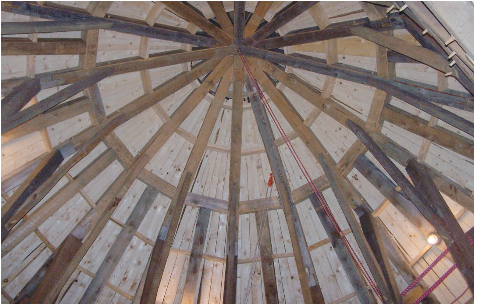
Fig. 15. View of underside of finished conical roof. Braced rafters are scarfed at inner posts.
