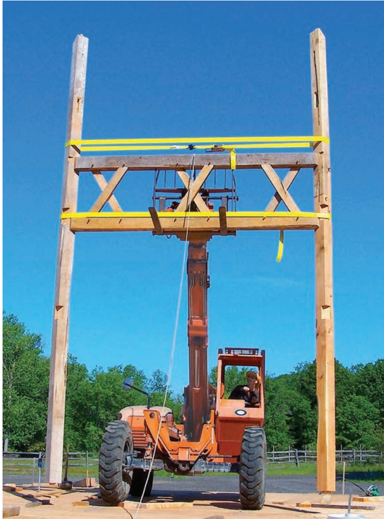
Fig. 8. Lull forklift and first assembly, truss over pentagon opening.
