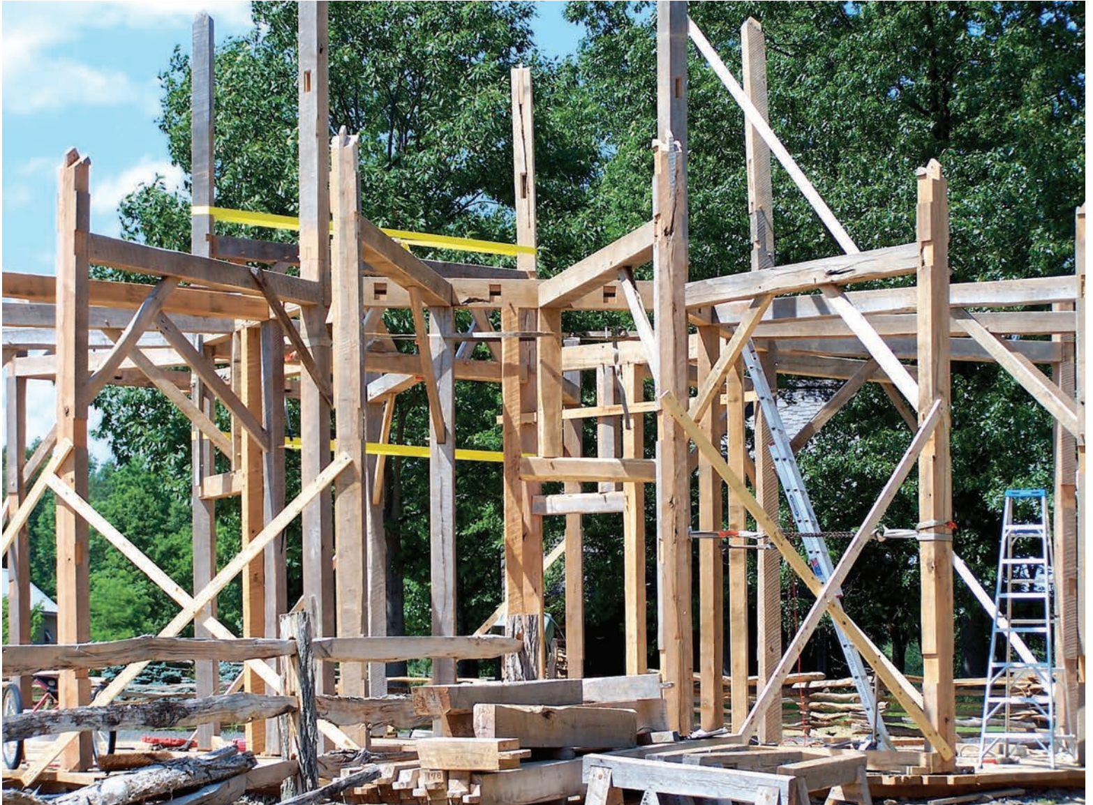
Fig. 10. Half-bents installed around structure, ready for wall girts, braces, plates and rest of joists. Ties run post to post, joists header to post.
