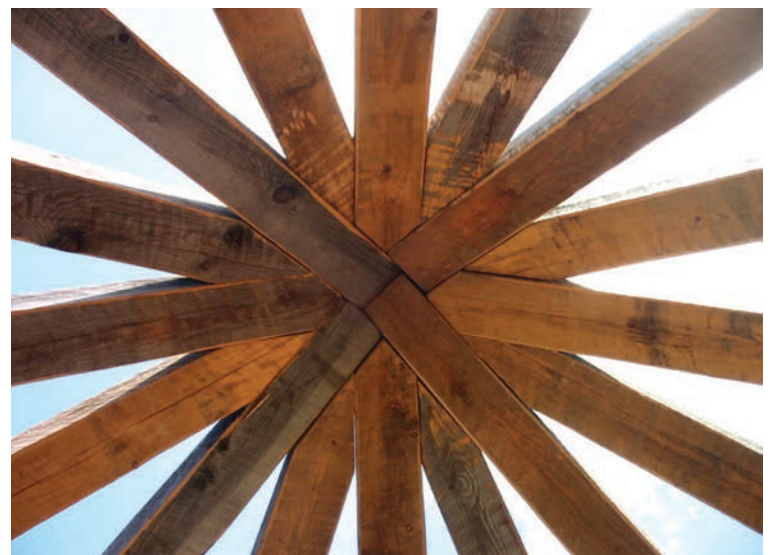
Fig. 13. Built-up peak joint, seen from below, begins with tenoned rafter pair, then adds housed pair, then 45-degree-nosed pairs, and last 22.5-degree-nosed pairs.
