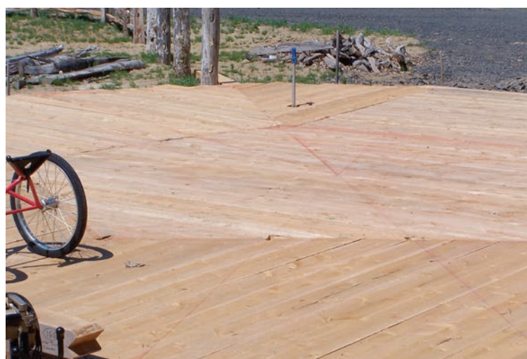
Fig. 7. Actual lines snapped on hemlock deck. Note post mortises.
