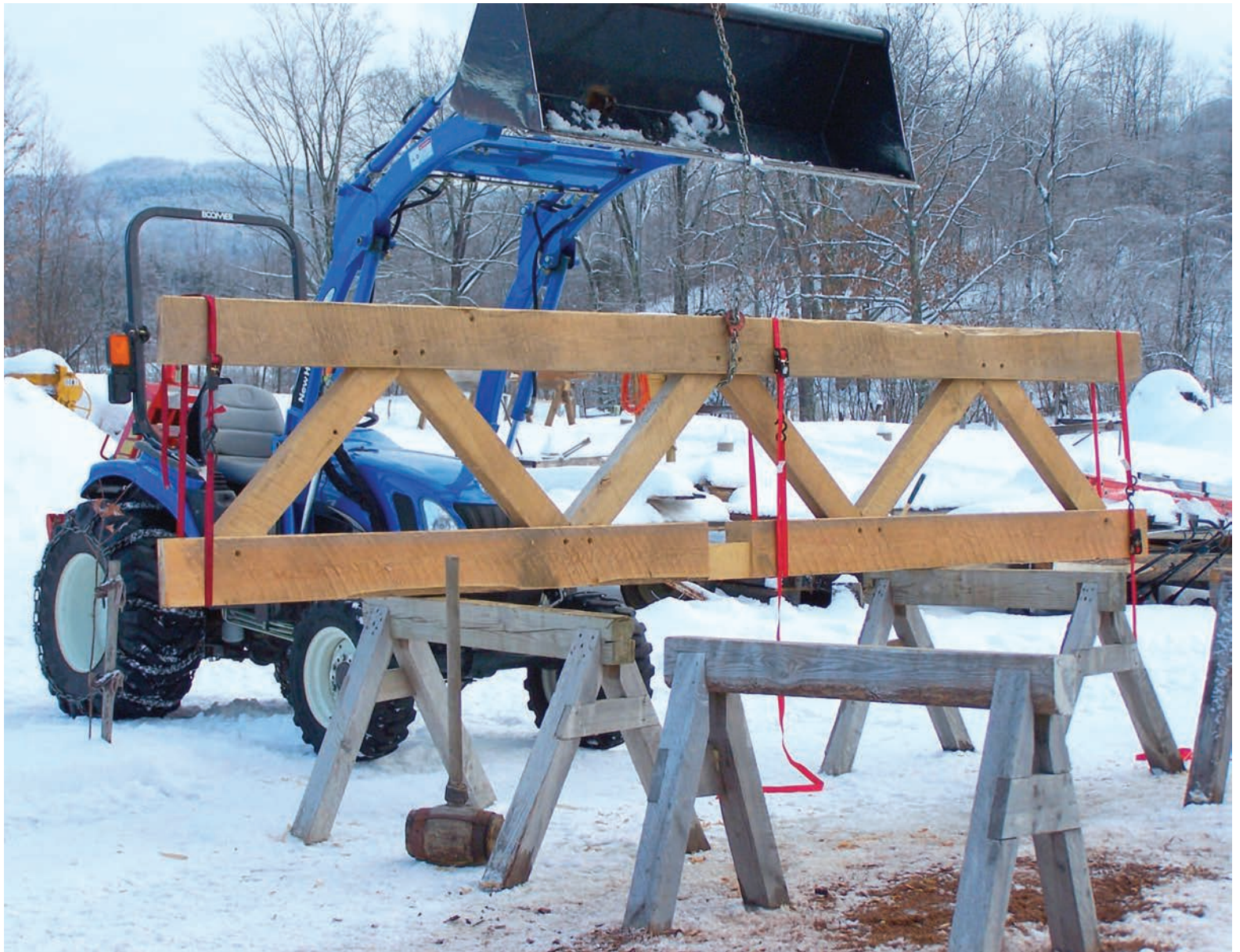
Fig. 4. At author's framing yard in Belcher, N.Y., building locust truss to bridge barn door opening. Steel tension rods not yet installed.
