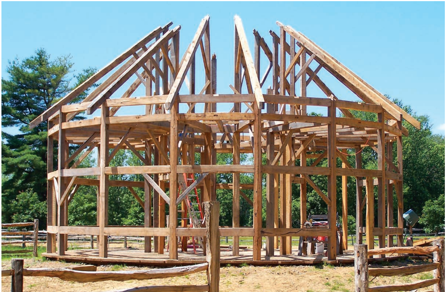
Fig. 12. Lower rafters with braces in place, spanning inner and outer posts. Scarf joints await upper rafters.
