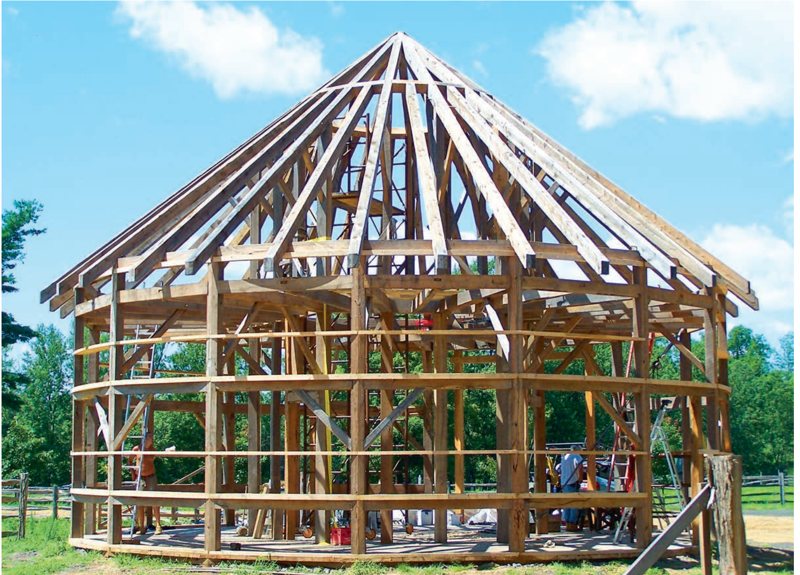
Fig. 2. Locust and hemlock 40-ft.-dia. round barn frame complete. Nailers are sawn to template arc for vertical board siding. Posts are backed but parallel sided, requiring girts and plates to meet at non-orthogonal joints and braces to meet at compound joints.
