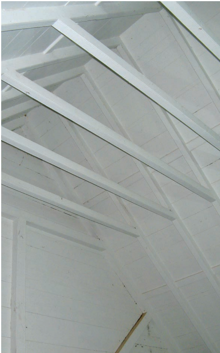
Fig. 6. Rectory roof framing comprises paired, collared rafters with mortise and tenon joinery and all members planed, beaded and painted.
