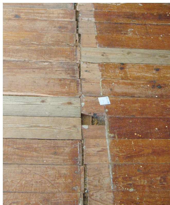
Fig. 3. Matched room-length yellow pine floorboards butt-joined under a partition.
