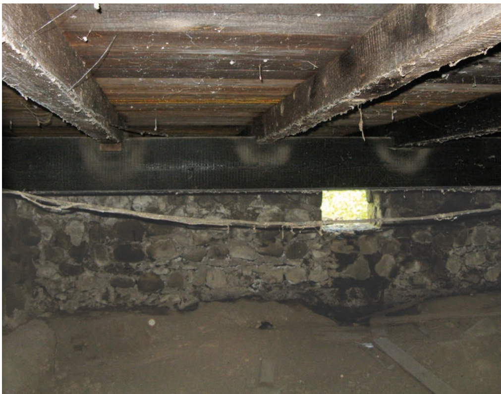
Fig. 2. Sawn girder and joists under rectory. Despite apparent ventilation, a radiating fungal decay has infected girder and joists.
