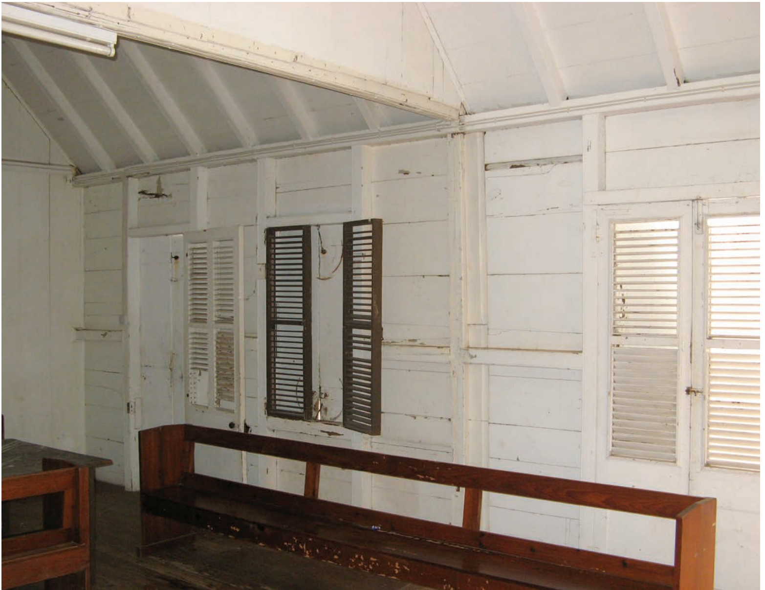
Fig. 4. St. Kitts rectory wall framing is as light as possible, with intermediate girts and horizontal sheathing used to stiffen the studs. All connections are pinned mortise and tenon. Some tie beams appear to lap over wall plates, as in Fig. 7, others join flush as in Fig. 8.
