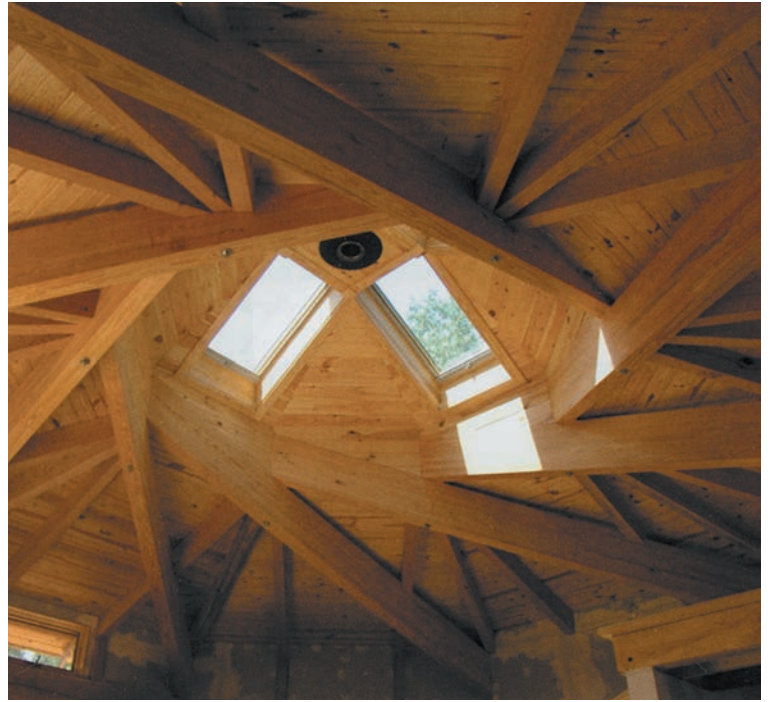
Gunn stovepipe opening is framed to accommodate planned chimney.
