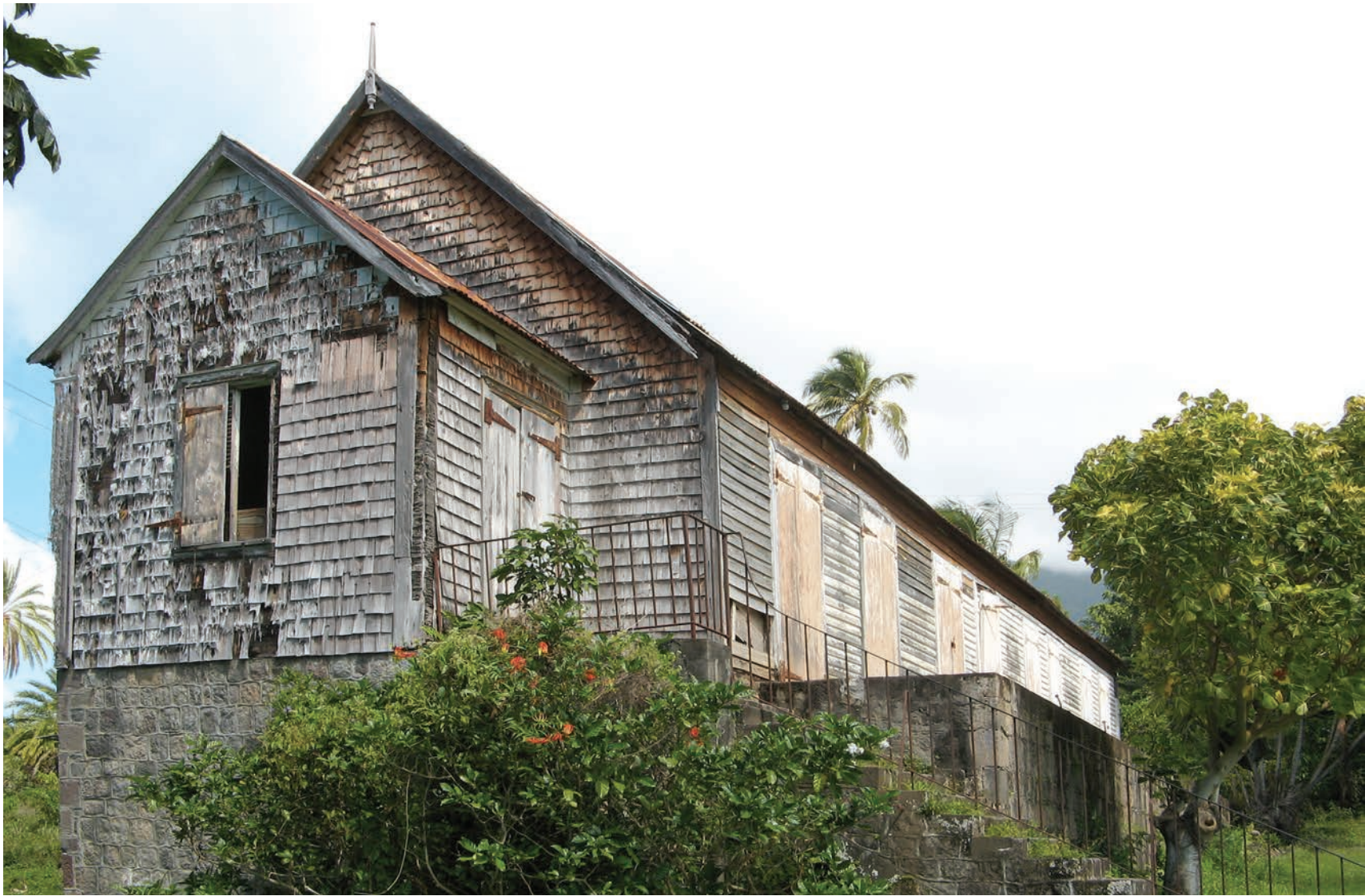
Fig. 1. St. Kitts rectory, ca. 1760, from southeast. Note shingled end with decorative treatment under rake and contrasting clapboards (planed and beaded) on eaves wall, whose doors open onto a stone terrace. Graceful ironwork and skilled stonemasonry are in good condition.
