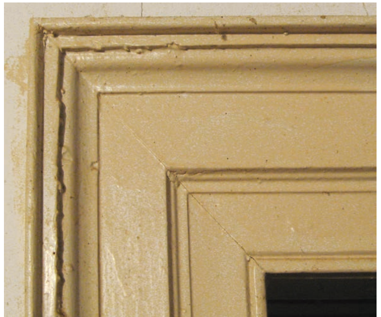
Fig. 9. Rectory double-fielded door casing. By 1775, miter for interior field and square cut for outer field had replaced full miter cut.
