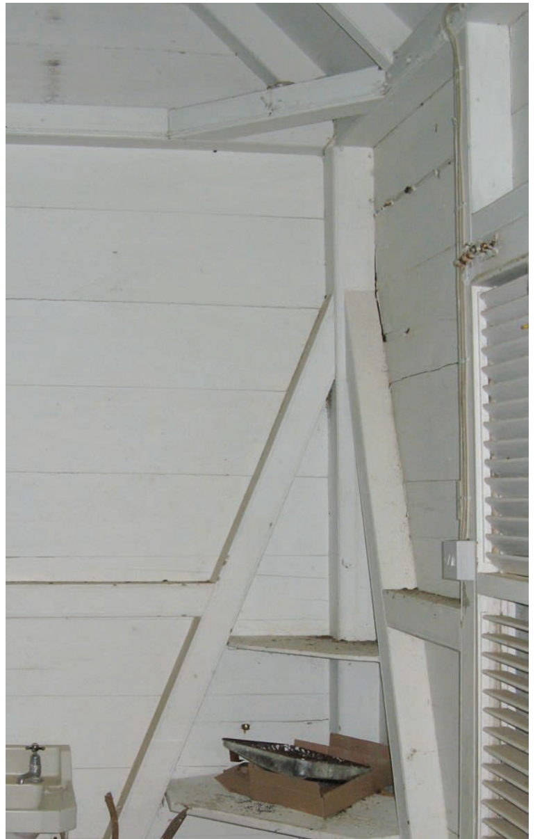
Fig. 8. Corner bracing is thorough, with relatively long down braces for the walls and short ties for the endwall and sidewall plates. Wall braces are further stiffened by intermediate girts.
