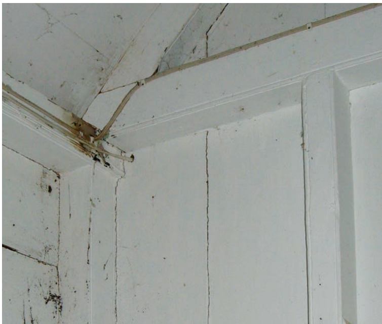
Fig. 7. Tie beam at some locations apparently laps over wall plates, though joint is invisible.
