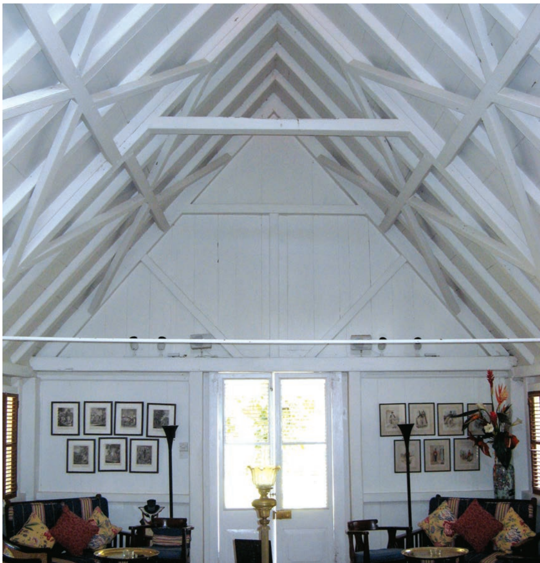
Figs. 11–13. At right, view of earliest part of L'Ermitage, with exposed wall and roof framing. Common rafter roof has few collars but purlins and many windbraces in second, inner layer. Tie beam at endwall laps over plates and is replaced at middle of room by iron tie rod passing through plates, below; near-X-braces join purlins and rafters in staggered connections, below and below right. All framing timber is lignum vitae , planed and painted.
