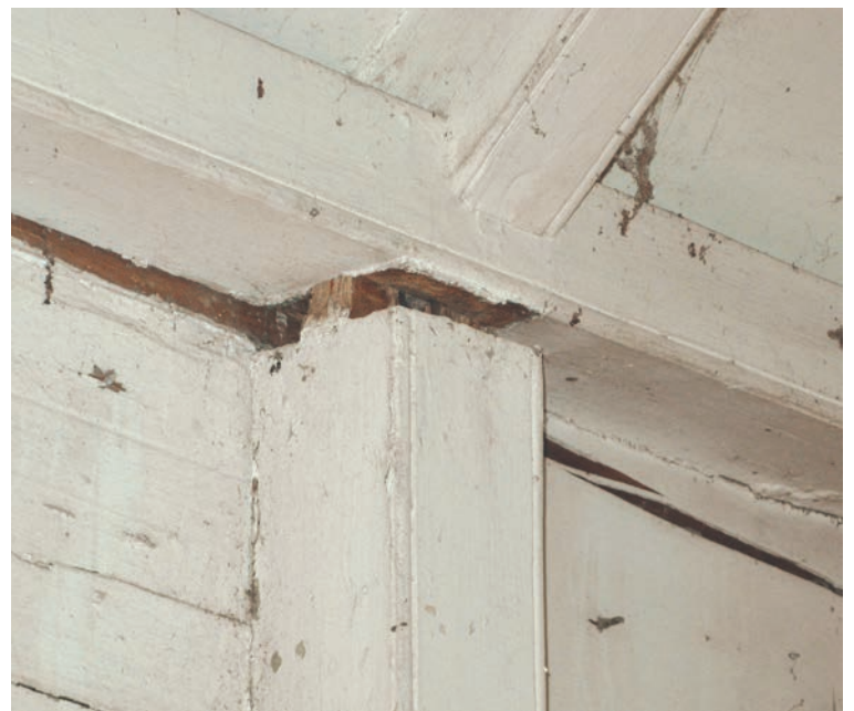
Fig. 5. Wall post subsided from termite damage in sill, mysteriously splitting wall sheathing; plate and rafter held up by roof sheathing.
