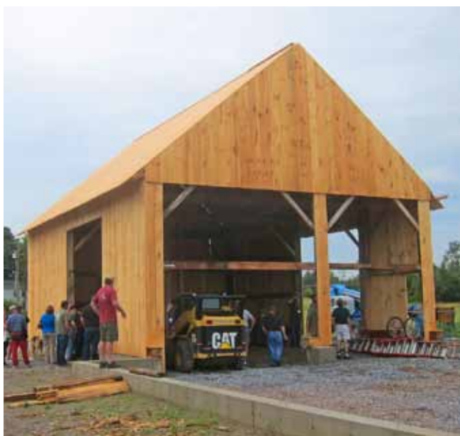
Above, Handy triple bypass barn, Williston, Vermont, late 1790s, showing in-kind repairs.
