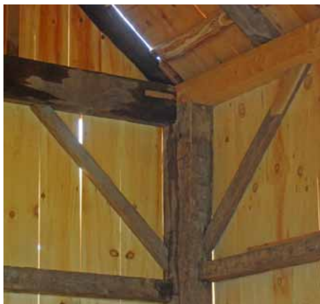
Above, Handy triple bypass barn, Williston, Vermont, late 1790s, showing in-kind repairs.
