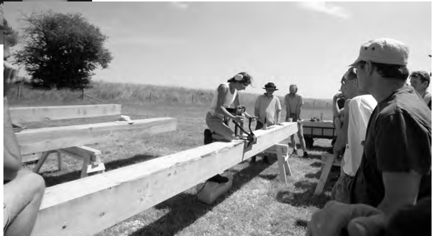
American Girl Timber Framer Donna (The Primo Donna) Williams from Virginia demonstrates the "chainsaw on a stick" Makita 1701B mortiscer, a highly favored power tool for making those slots in timbers. U.K. framers are slack-jawed in amazement.
