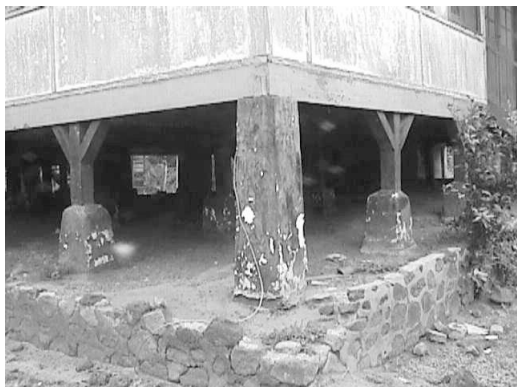
This detail of the living quarters the Germans built for themselves shows concrete columns about 4 feet apart supporting floor sills.
