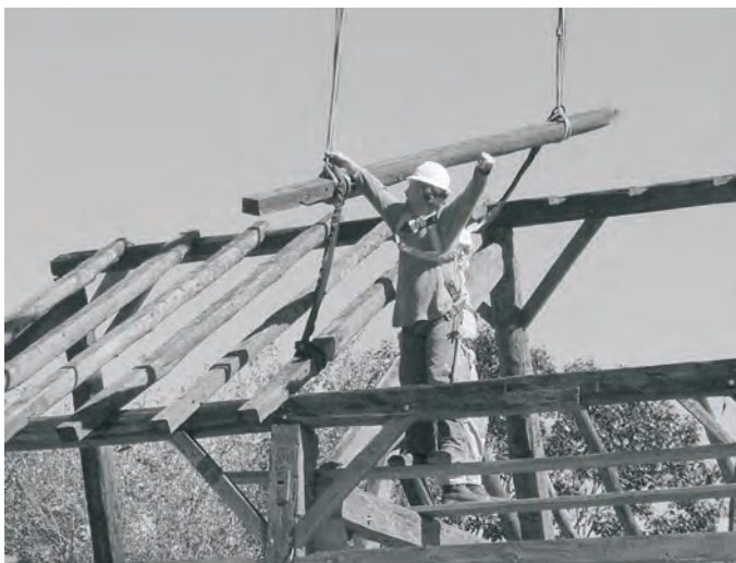
Facing page, Engineer Joe Miller (Grantham, N.H.) adds some high work to his résumé, setting x-bracing on the lower roof section. Far left, Will Truax hewing a replacement rafter. Left, Chris Newman setting multiples of lower rafters. Below, final pile of fun and crew before loading up.
