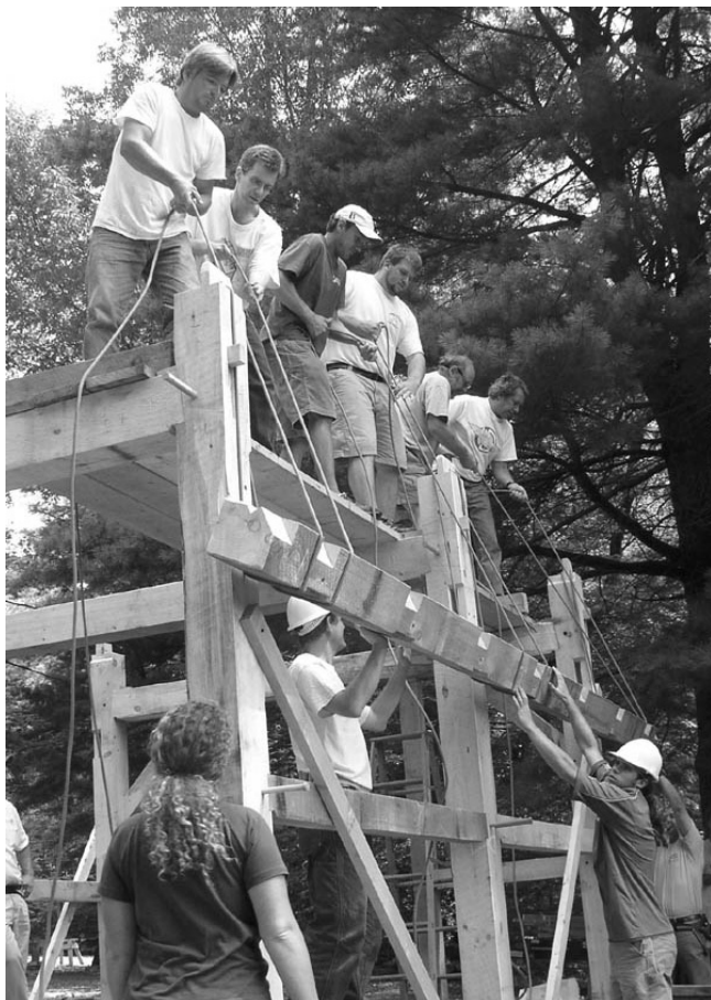
Facing page, from left, fitting up a door frame in a bent prior to raising. At right, Dave Carlon demonstrates the French method of drawboring—"point to the joint"—with Jason Long looking on. Paul Martin (behind Dave) appears skeptical, but it works!
