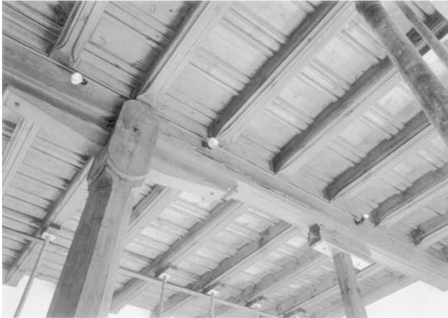
A photo from Vit Mlazovsky's talk at the Estes Park conference showing the dominant type of ceiling construction in the castle of Karlstejn (in Bohemia, Czech Republic). The main girder is partially damaged by a shear crack.
