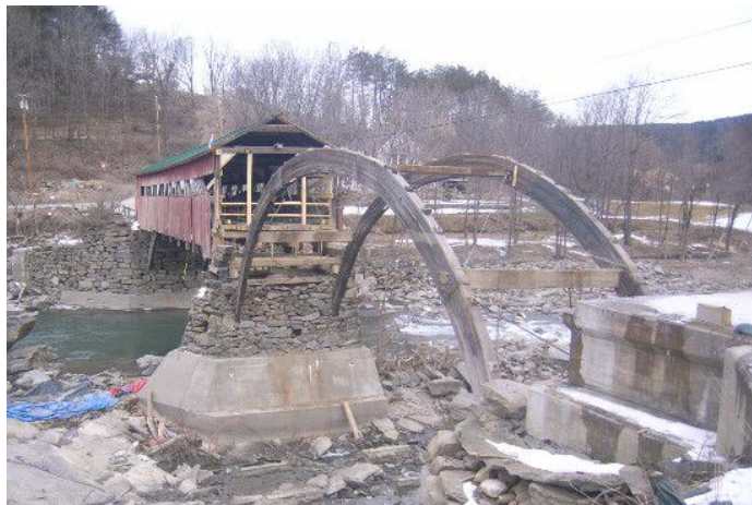
Taftsville Covered Bridge – rehab underway post Irene damage. A pair of the largest supplemental timber arches known to this author!
